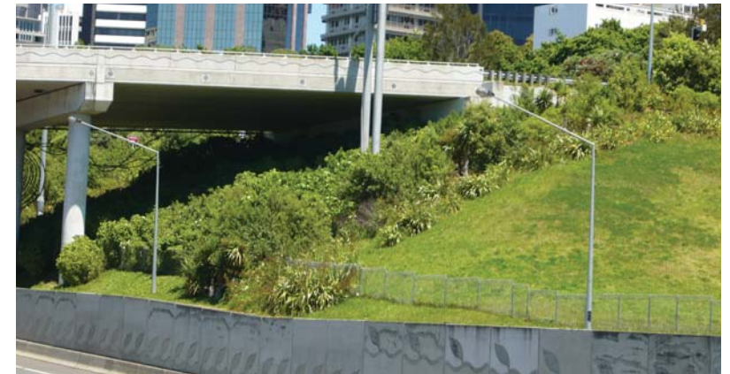
Continuous planting through open abutments strengthens a sense of visual continuity for the 'green' edges of the motorway. Careful selection of plant species together with adequate drainage will support this condition
