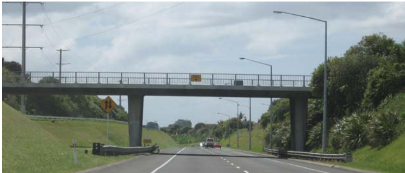
Above: This existing bridge on SH2 at Tauranga has a simple tapered column form that is a good precedent for the TEL. The open abutment optimises views along the highway while the shallow deck emphasises the horizontality of the structure.
