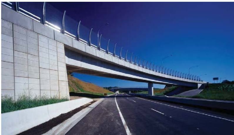
Below: Brunswick to Yelgun, Pacific Highway, NSW Australia. The setback below the parapet both breaks down the apparent depth of the structure and creates visual interest through the shadow line. The effect is streamlined and elegant.
