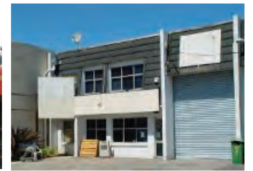
High stud industrial Buildings - south of Church Street
