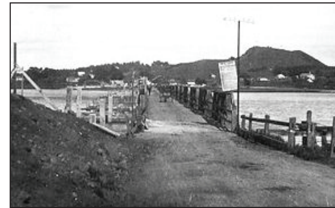
Mangere Bridge, Under Construction c1913
