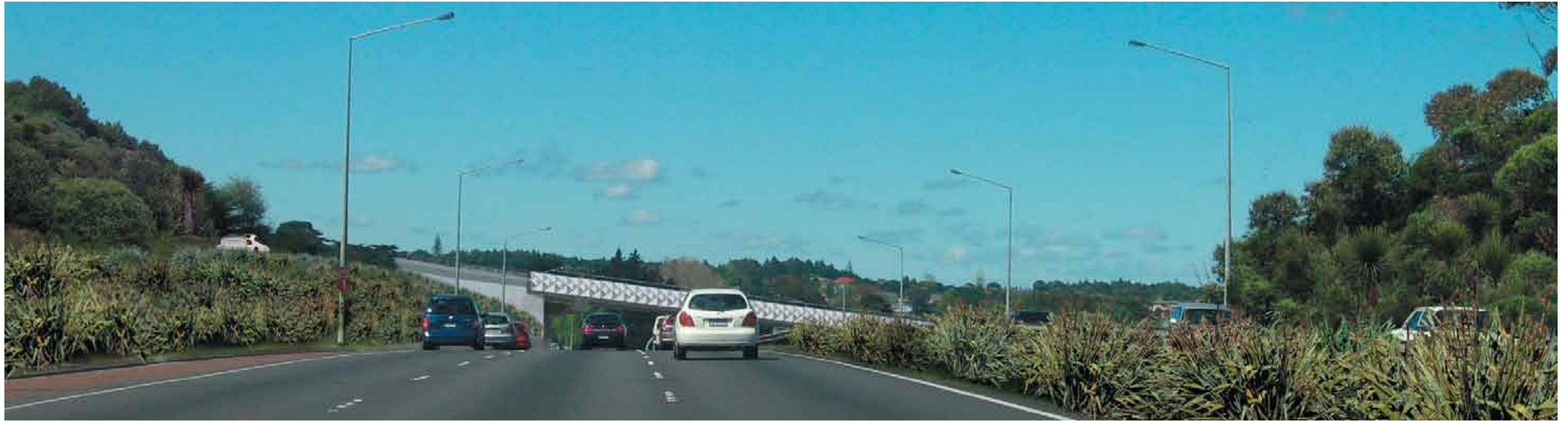
Figure 8.31 - Redoubt Road Flyover view Southbound from State Highway 1
