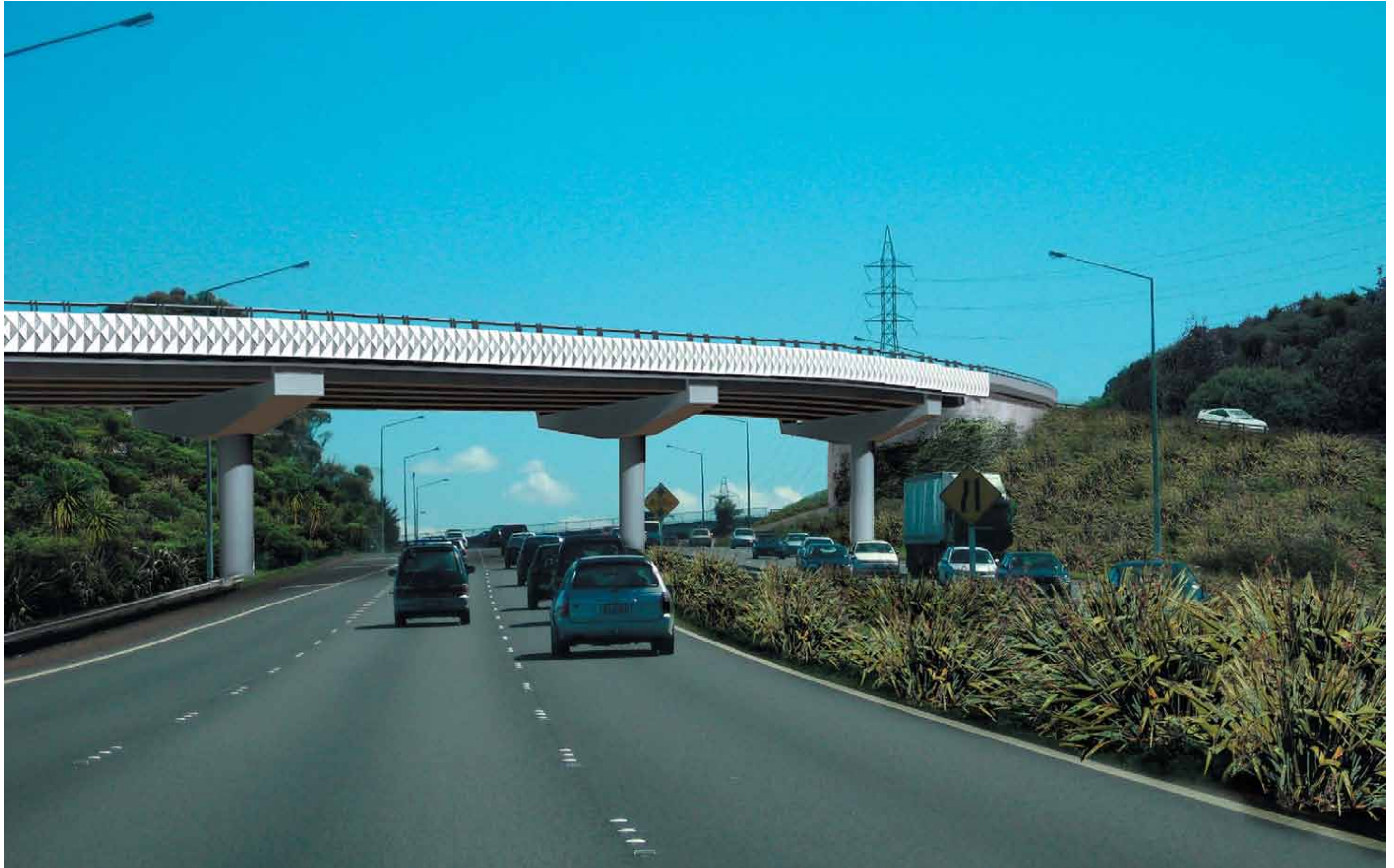
Figure 8.27 - Redoubt Road Flyover viewed from State Highway 1 northbound, showing piers with splayed crosshead beams and barriers
