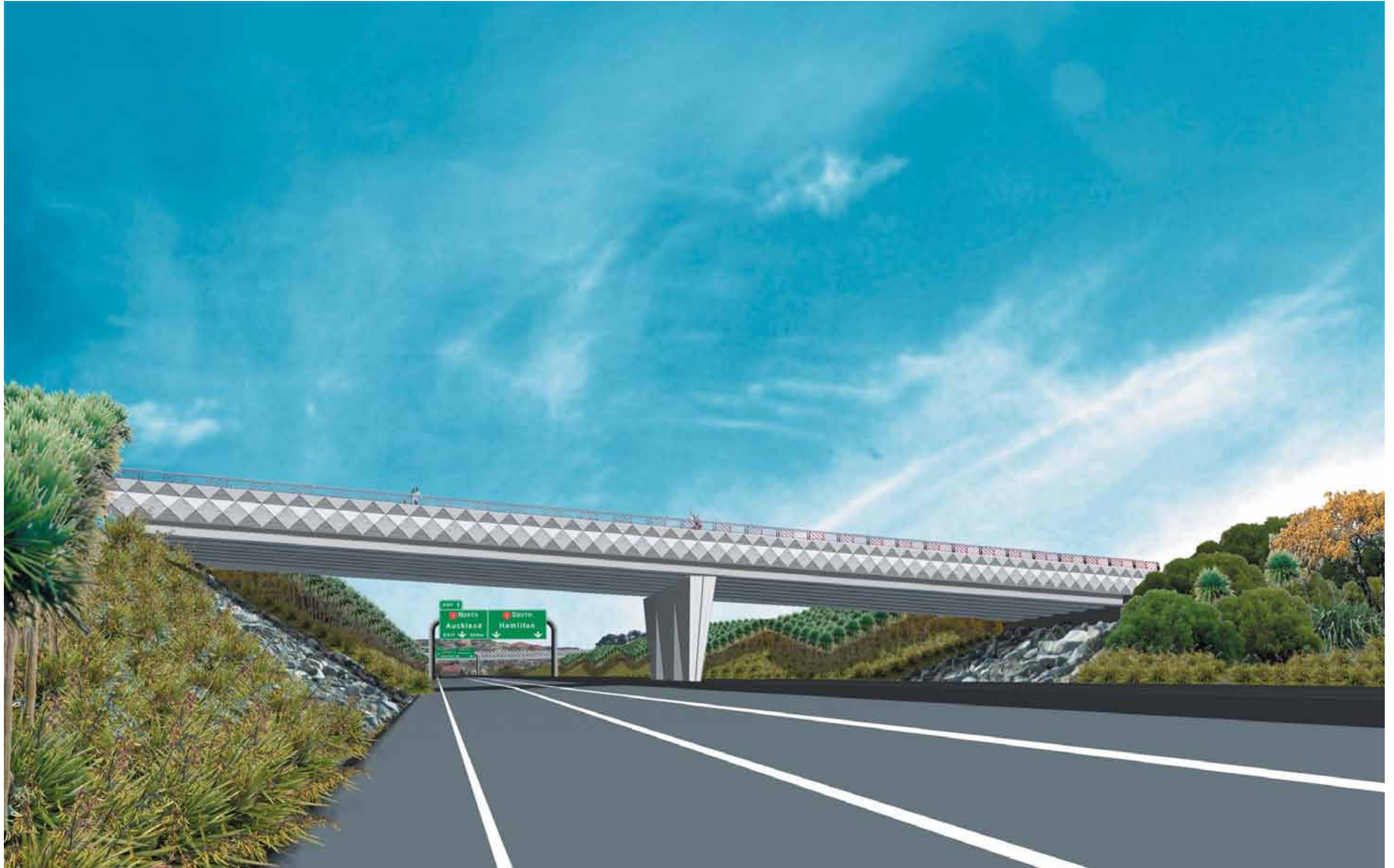
Figure 8.23 - Barrowcliffe Place bridge, eastbound view, showing triangular Pacifica motif and painted decorative railing to the barriers, in situ concrete tapered 'W' pier and volcanic rock lined spill through abutments. Great South Road bridge beyond
