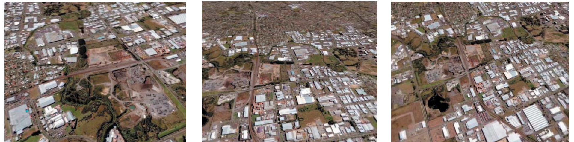
Figure 4.6 - Aerial photographs of the industrial context of SH20 Manukau Extension
