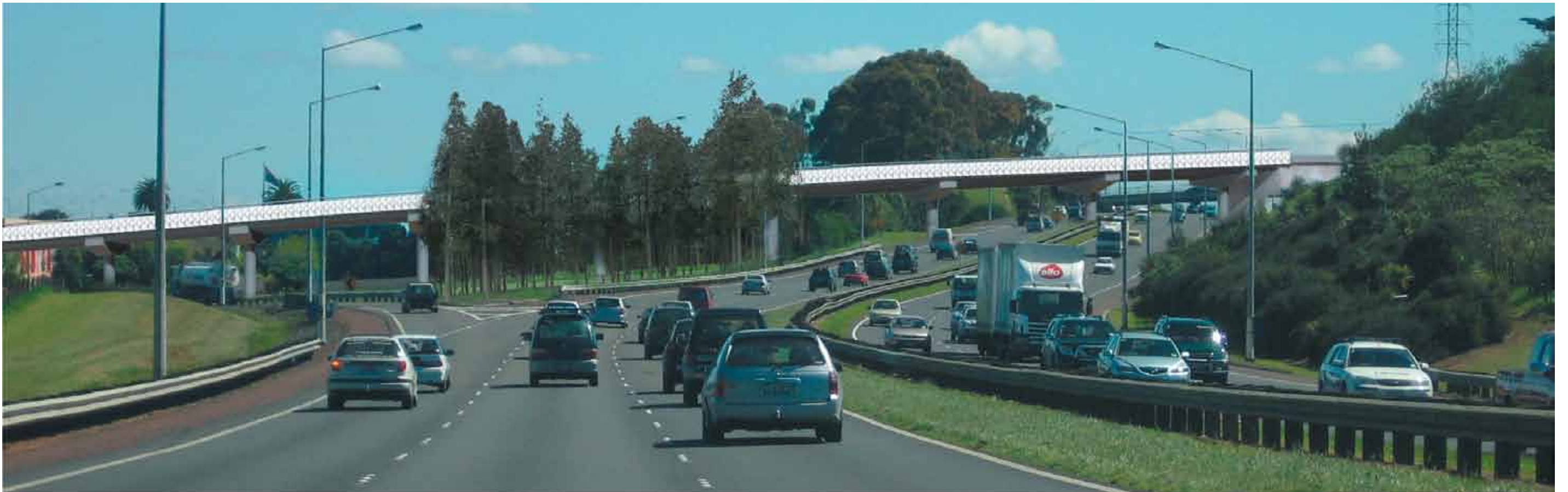
Figure 8.32 - Redoubt Road Flyover view Northbound from State Highway 1 approaching Manukau City interchange
