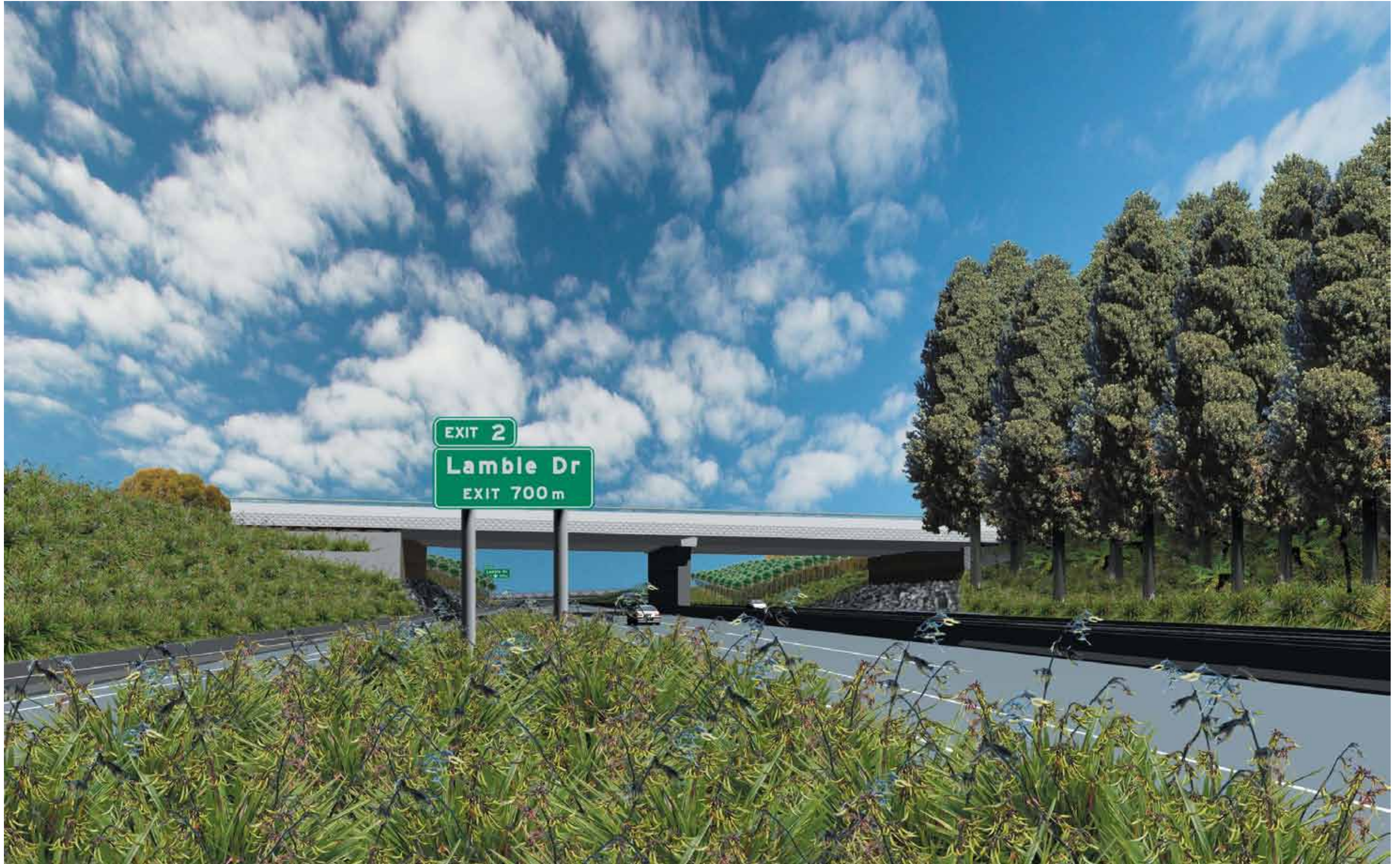
Figure 8.24 - Great South Road bridge, westbound view - the eastern entry portal to State Highway 20. Facetted Leading Edge barrier, heavily rusticated finish to both MSE abutment walls and central pier precast concrete cladding panels are the main features of this bridge
