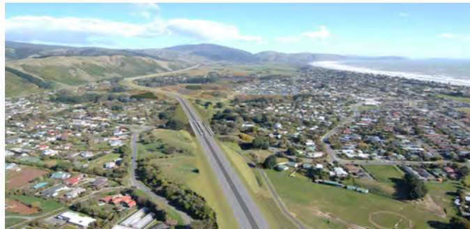
Figure 125 Indicative view south to QE Park with Raumati Rd crossing in foreground
