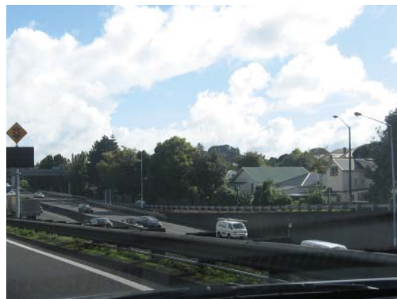
Houses at or slightly above level of motorway road level
