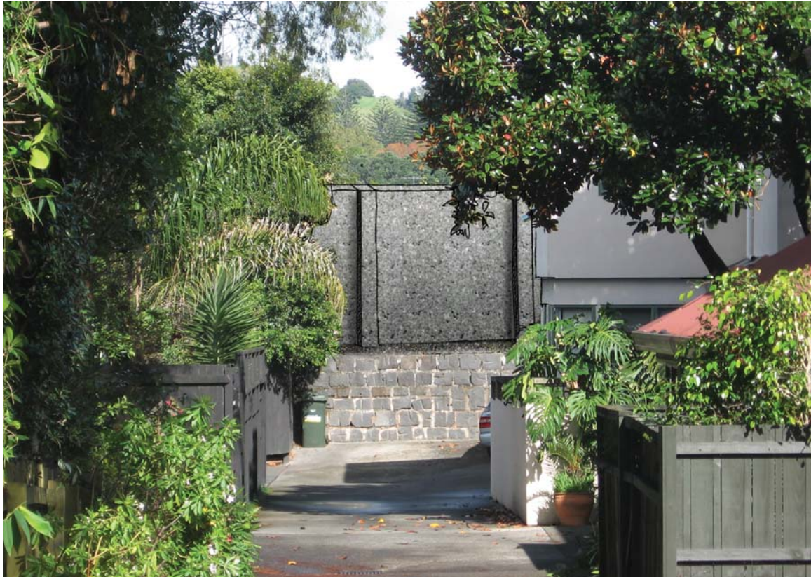
Existing Conditions & Examples of Concrete Noise Walls
