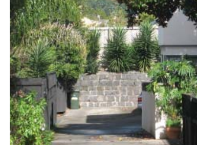
Care has been taken by some residents to create an attractive back garden incorporating existing retaining wall, timber fence and planting
