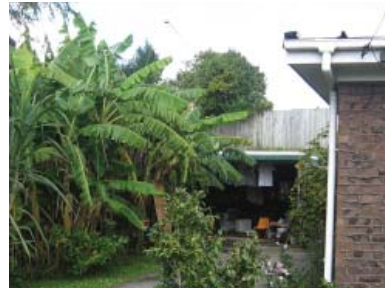
Carport built against existing retaining wall
