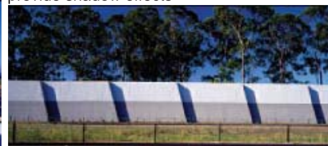
Concrete Panels staggered can provide shadow effects
