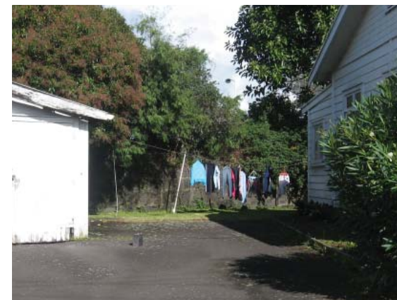
Existing retaining wall and vegetation screens the visual effects of the motorway
