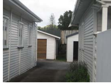
A variety of materials and finishes of boundary fence between two residential properties
