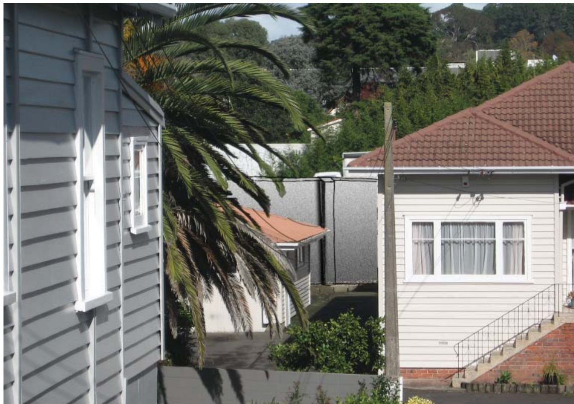
Existing Conditions & Examples of Concrete Noise Walls
