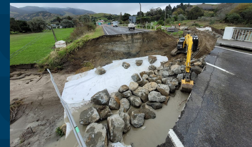
Repair of the Mangahauini Bridge
