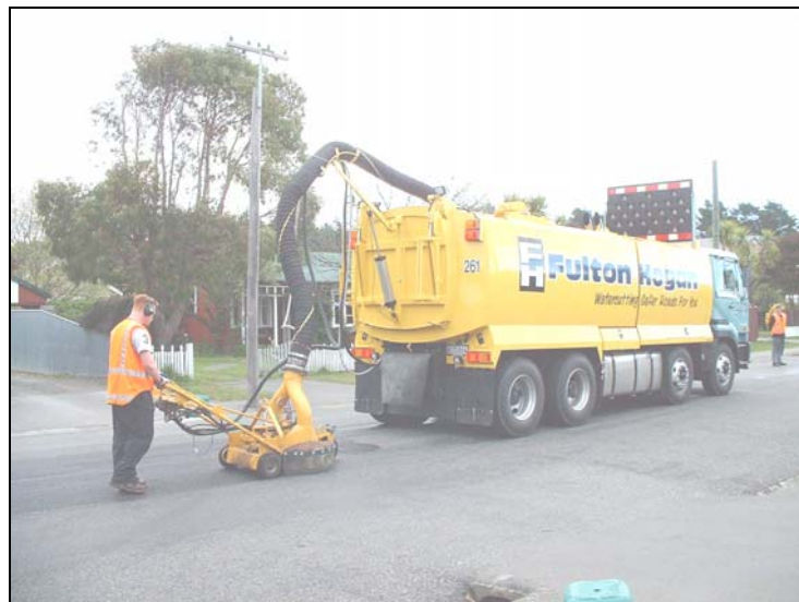
Figure 2. Water supply and vacuum recovery system
