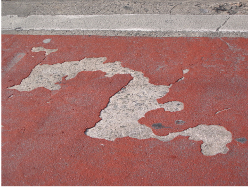
Figure 3: Cold Applied Plastic Coloured System applied to a concrete substrate
