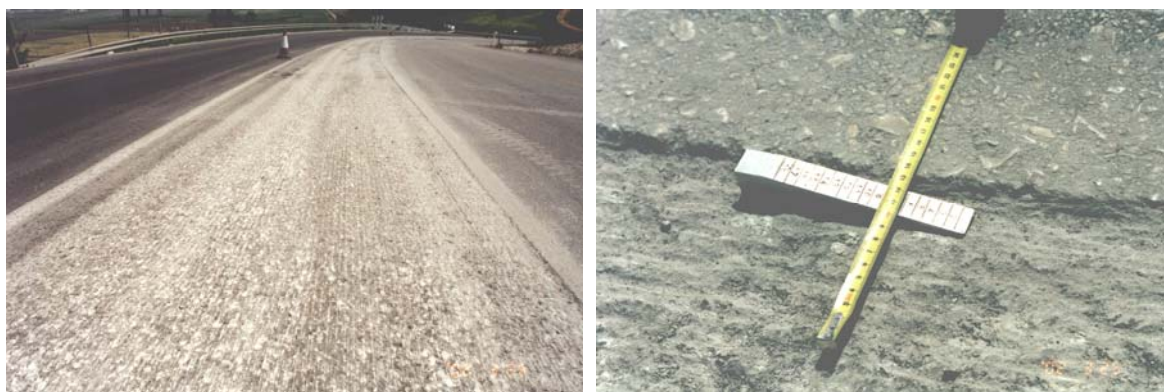
Figure 13: Examples of the results of a fine milling retexturing process
