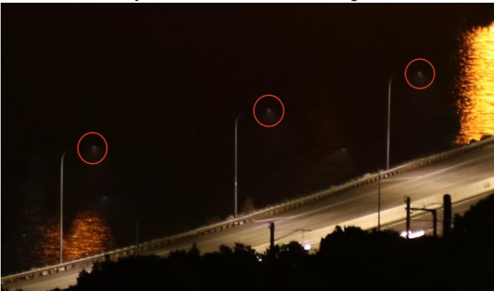
Figure 4-8: Lighting on the WUM showing that no direct light was coming from the LED luminaires. The position of the luminaires is circled in red.
