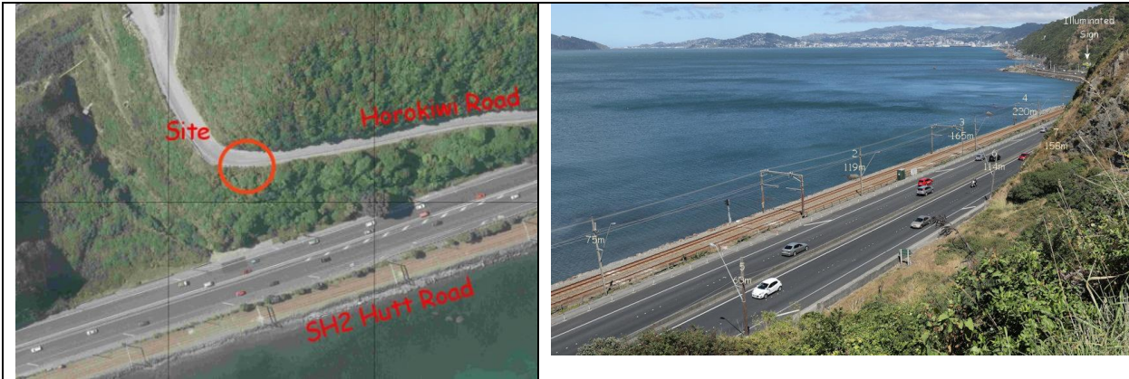
Figure 4-10: Horokiwi road site and its view of Hutt road
