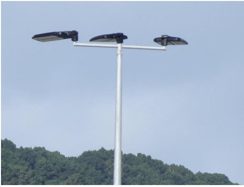
Figure 4-15: Light A with zero °s tilt. It produced uplight of 40 cd- less than a single HPS luminaire.
