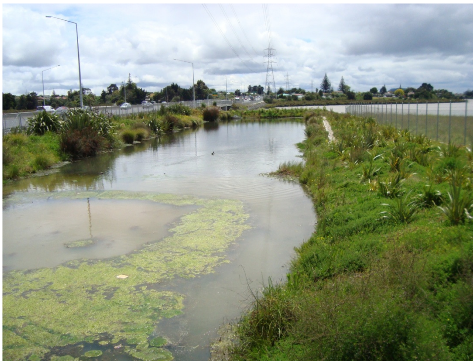
Photo 8: Pond where the forebay looks as if it needs sediment cleaning
