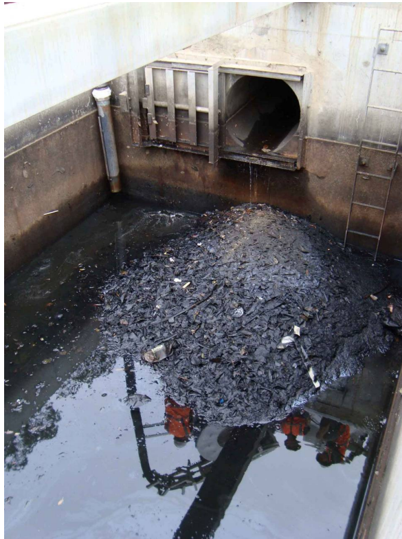
Photo 5: A sediment Chamber full of Sediments
