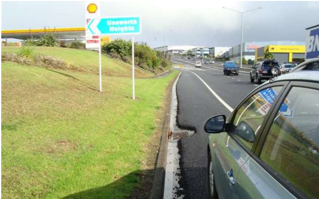
Figure 5-3 Catch pit sediment, SH18 Upper Harbour Corridor (westbound) at Unsworth Drive
