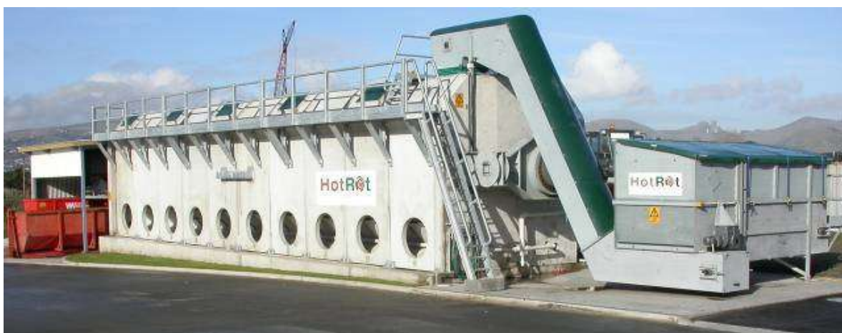
Figure 8-2 Example of an in vessel composting system
