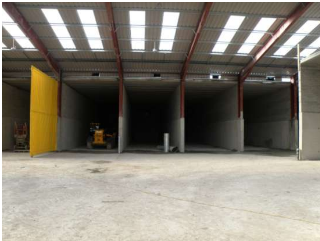
● Figure 8-4 Inside of Composting Building – Tipperary
