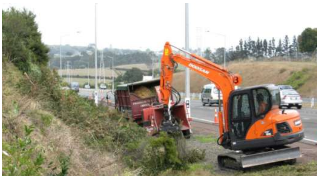
Figure 7-1 Arborist mulch being produced woody weeds (cotoneaster, privet and spanish heath) at Ramarama. This mulch must be composted to kill weed seeds before reuse.
