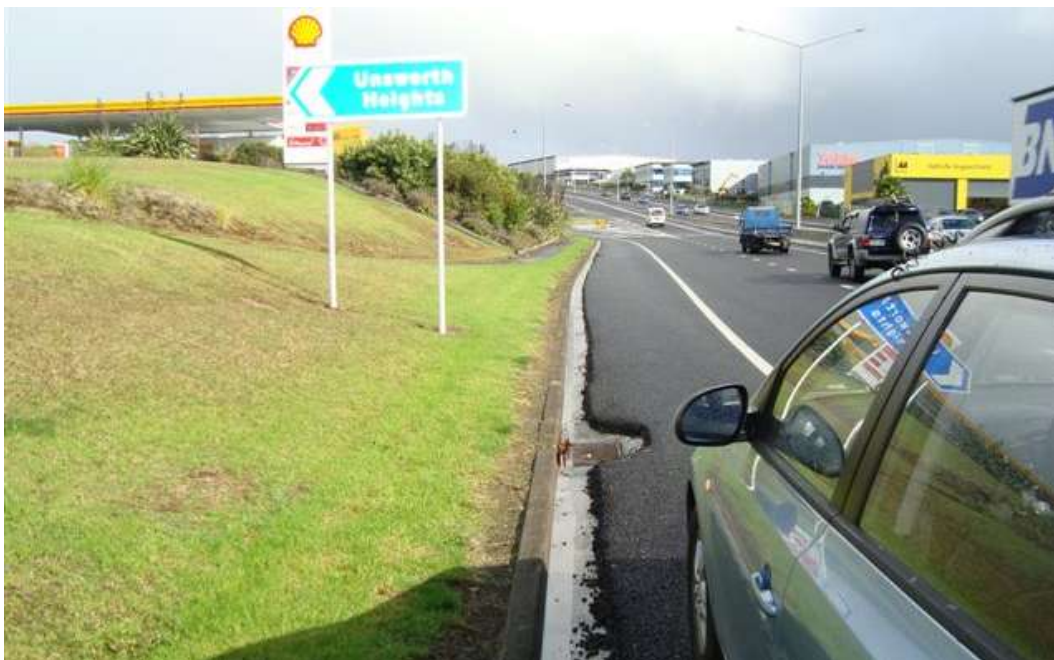
Figure 0-3– catch pit sediment, SH18 Upper Harbour Corridor (westbound) at Unsworth Drive
