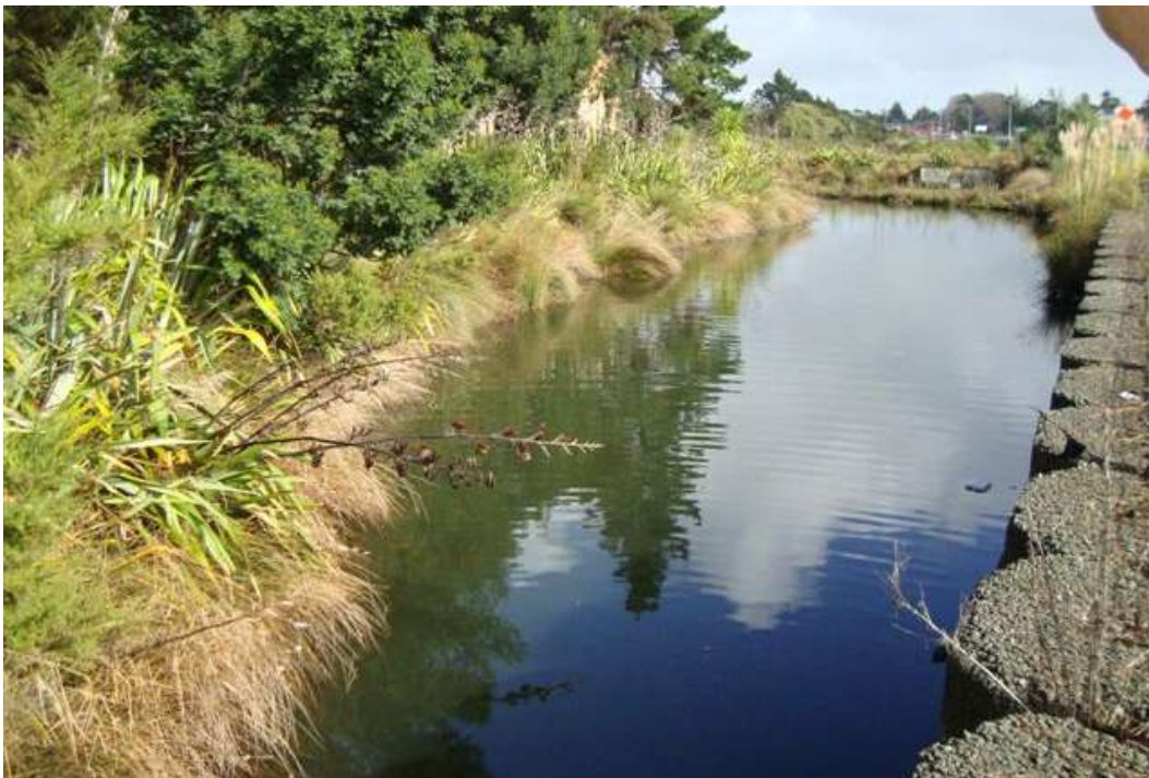
Figure 0-2– Causeway Lagoon Pond, SH18 (westbound) Upper Harbour Bridge and Causeway (AMA-2)
