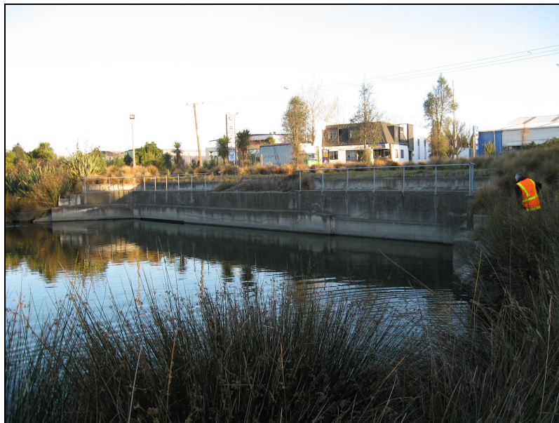
Photo 1: Halswell Retention Basin – Pond Inlet Area
