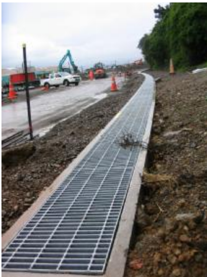
Photos 5 & 6: New open channel cut off drain and the new 1800 diameter Percy culvert inlet during heavy rainfall part way through construction
