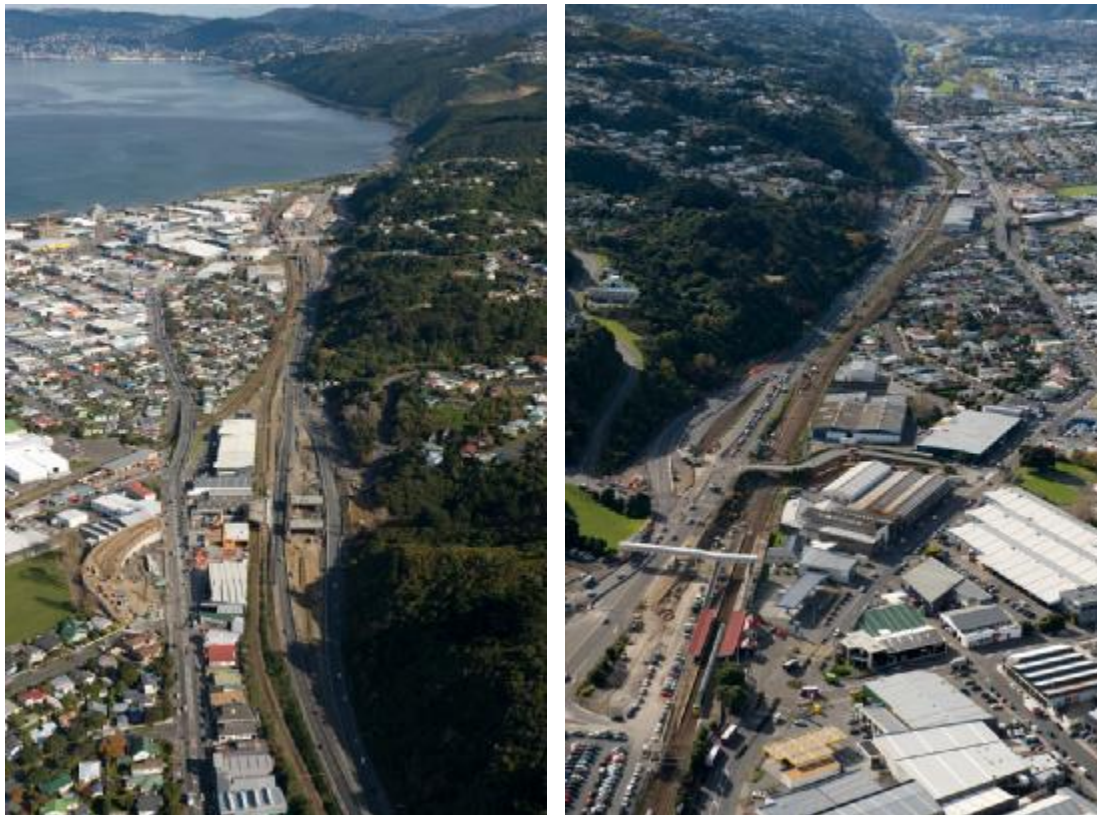
Pictures 2 and 3: Western half of the SH2 D2P site looking west towards the Harbour (left photo) and the eastern half of the site looking east towards the Hutt River (photos courtesy of Above Ground Ltd).
