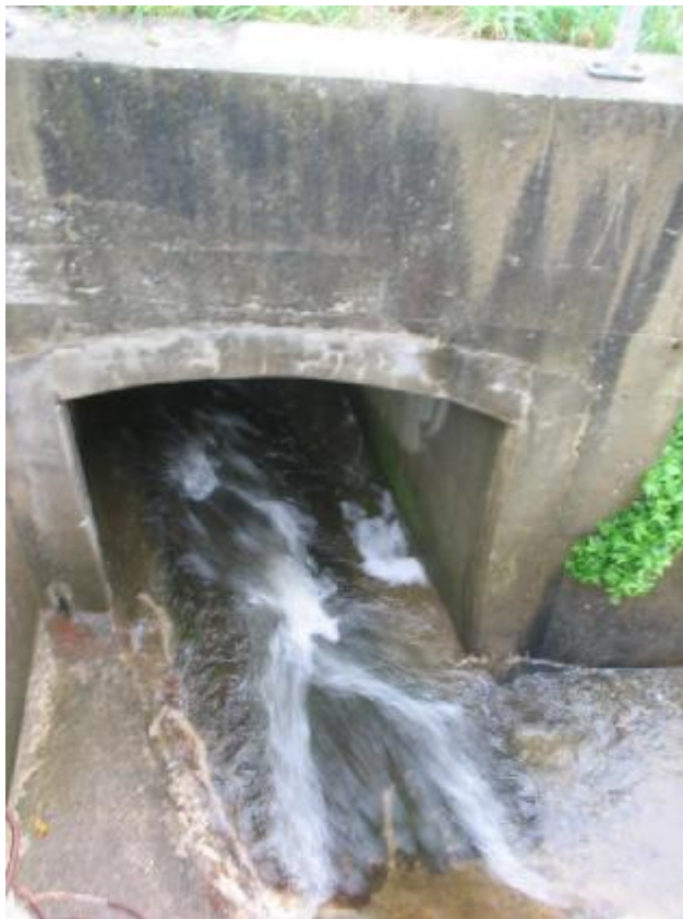
Photo 4: Existing entrance to the Western Hills Culvert
