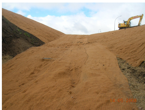
Stabilisation by revegetation and Gabion basket
