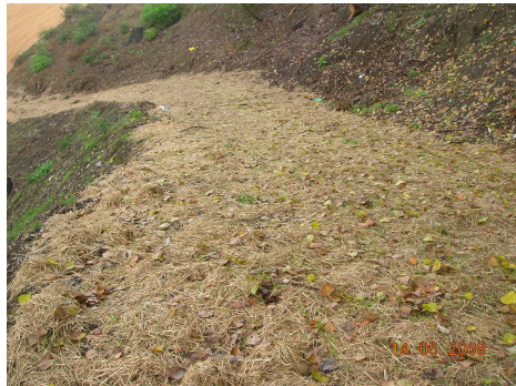
Mulching (Protective layer of straw)
