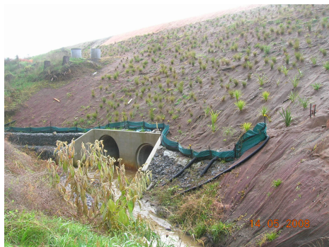
Stabilisation by revegetation and Gabion basket
