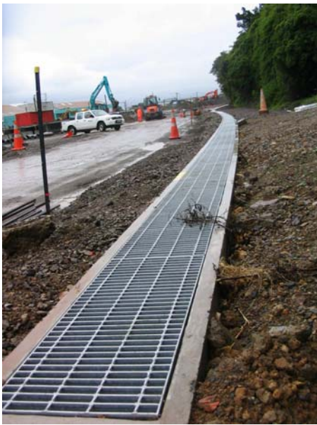
Pictures 5 & 6: New open channel cut off drain and the new 1800 diameter Percy culvert inlet during heavy rainfall part way through construction
