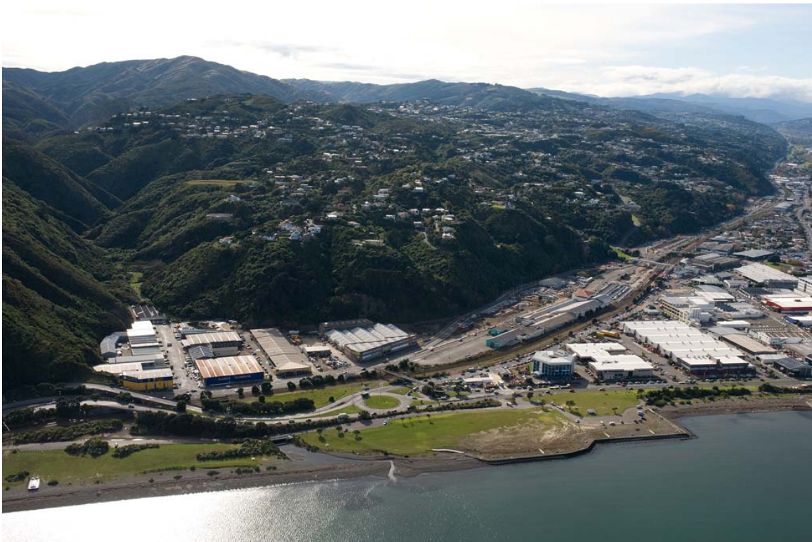
Picture 1: Western end of the site showing Korokoro Stream valley on the left with the stream outfall in Wellington Harbour in the foreground (photos courtesy of Above Ground Level).
