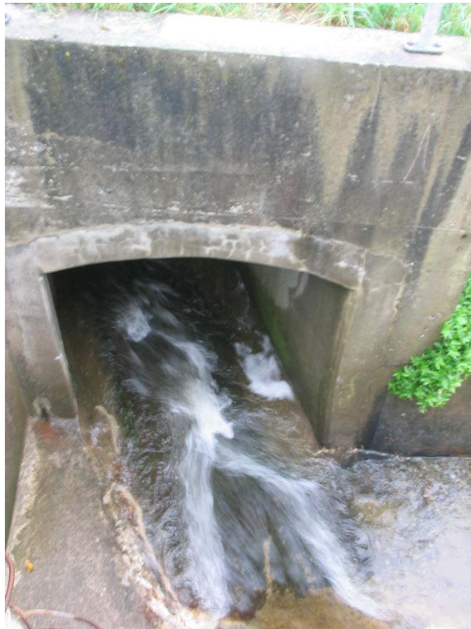
Picture 4: Existing entrance to the Western Hills Culvert
