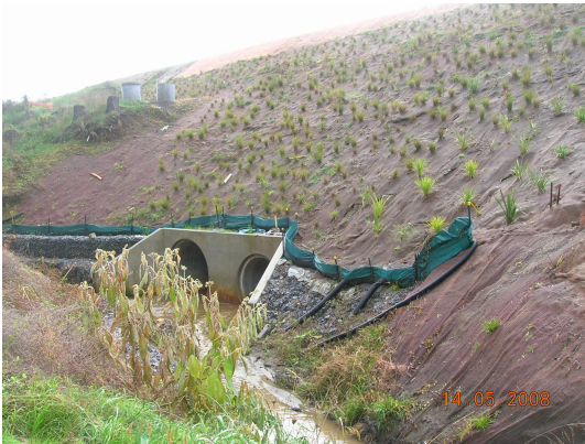
Stabilisation by revegetation and Gabion basket
