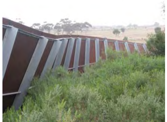
Figure 3.34 Visually effective low level planting against metal noise barrier, Melbourne
