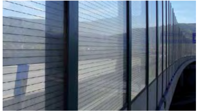
Figure 4.14 Some manufacturers are now producing barriers with bird deterrent markings in the form of thin black stripes. It is purported that these stripes are visible obstacles for birds while providing maximum transparency of the panel. (Source: Evonik Industries)
