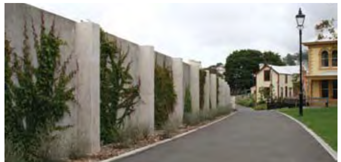
Figure 3.3 The location of noise barriers in relation to public space, shared paths and edge planting can help retain the character of an area, Wellington
