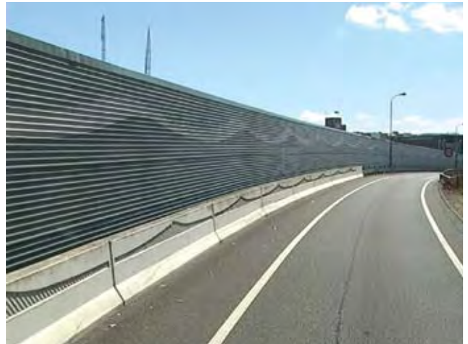
Figure 4.31 Corrugated metal panels can be used as a barrier, Khyber Pass offramp, SH1, Auckland
