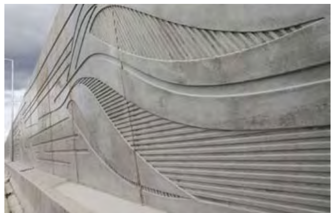
Figure 3.17 An integrated concrete safety and noise barrier, with simple, uncomplicated pattern so as not to distract drivers, SH20, Auckland
