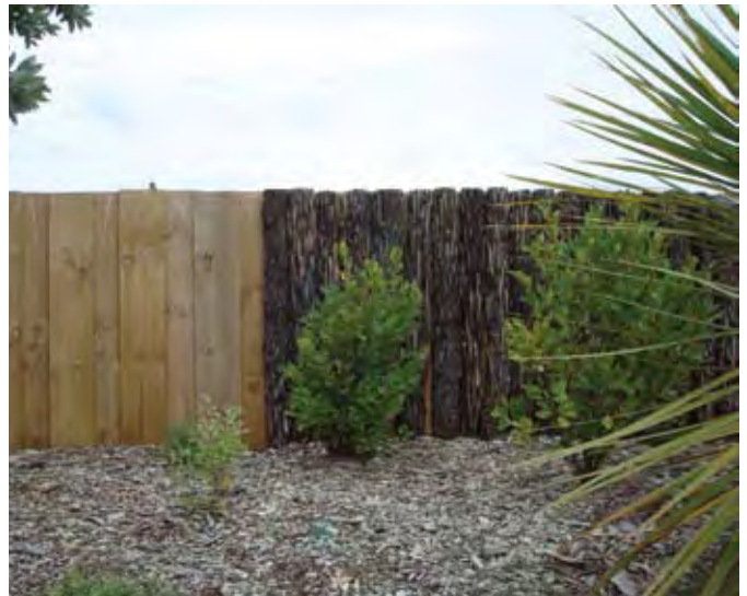
Figure 4.24 The design of the noise barrier surface can be an effective graffiti deterrent, such as the use of Punga logs on these timber noise barriers on the Tauranga Harbour Link
