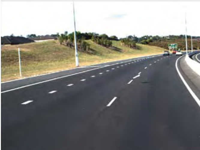
Figure 4.22 Planting grass on bunds requires regular mowing and therefore increased maintenance costs, SH18, Auckland
