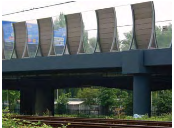
Figure 4.29 Transparent panels can be used on bridges to reduce the overall visual bulk of the noise barrier, Holland (Source: Forman Building Systems)
