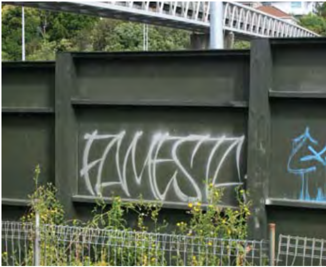
Figure 4.25 Graffiti or tagging is one of the biggest noise barrier maintenance issues facing the NZTA, Newton onramp, SH16, Auckland
