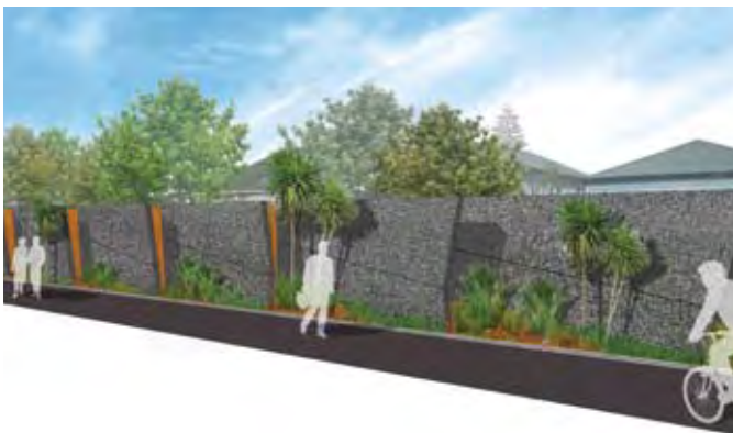
Figure 3.20 I-section posts can be emphasised attractively with colour where panels overlap, SH16 concept, Auckland
