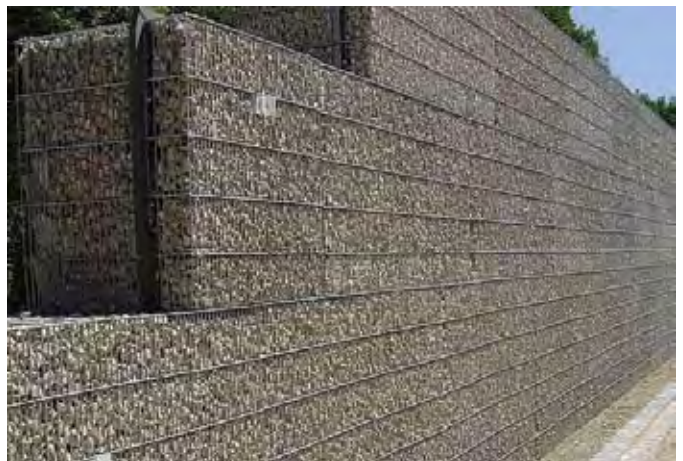
Figure 3.31 Gabions walls can be a visually effective noise barrier
