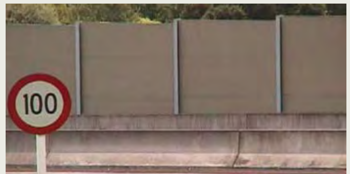
Noise barriers outside the Auckland Botanic Gardens were later removed after residential opposition
