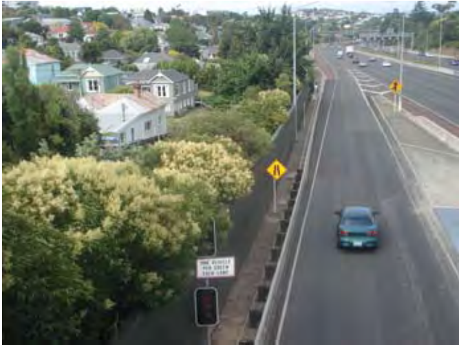
Figure 2.19 Vegetation can provide a perception of noise reduction greater than the objective barrier performance, Newton onramp, SH16, Auckland
