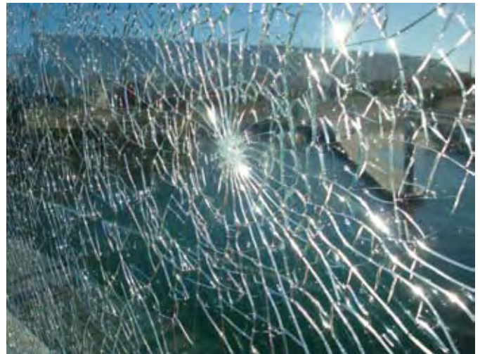
Figure 4.30 Transparent glass noise barriers are easily smashed by vandals, Tauranga Harbour Link
