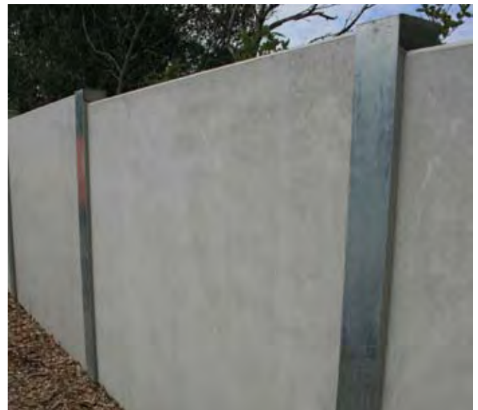
Figure 4.27 Lightweight modular precast concrete panels can be used in noise barrier design, Market Road, Auckland (pre-landscaping)
