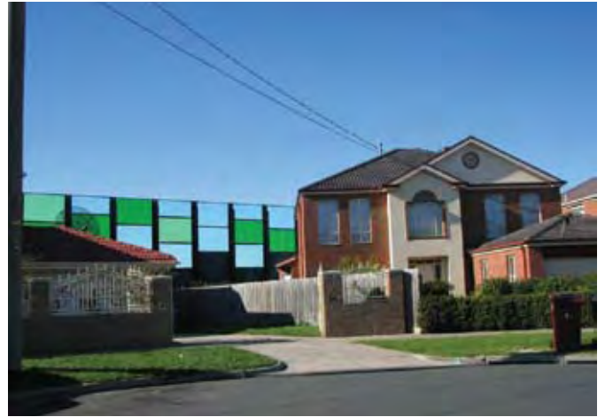
Figure 3.27 Transparent panels can be built taller and closer to buildings as they are less visually intrusive, Melbourne
