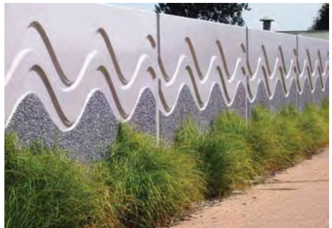
Figure 1.2 Noise wall, Avalon Drive, Hamilton
