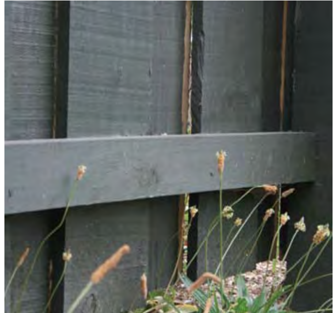
Figure 2.17 Timber planks are prone to warping, Auckland
