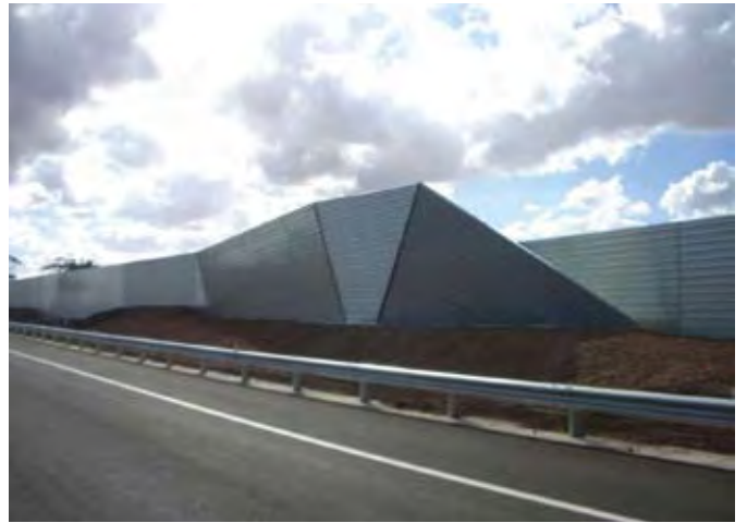
Figure 3.10 Architectural noise barrier emphasises change in height and overlap, Melbourne
