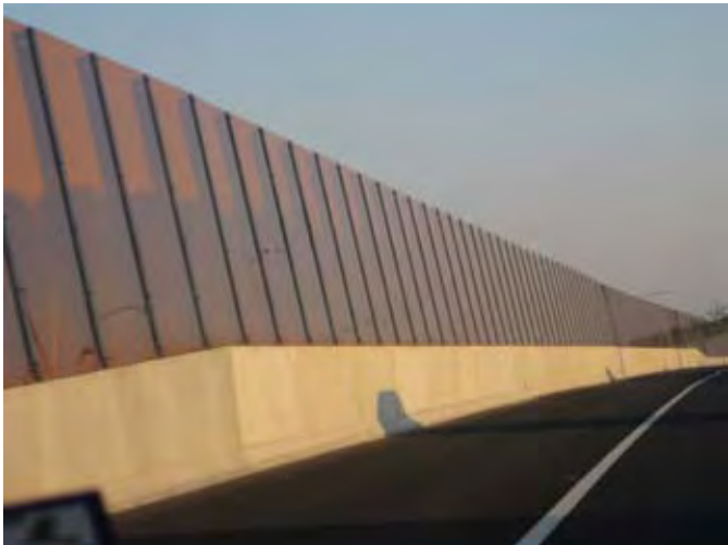
Figure 3.11 Angled transparent noise barrier, Melbourne
