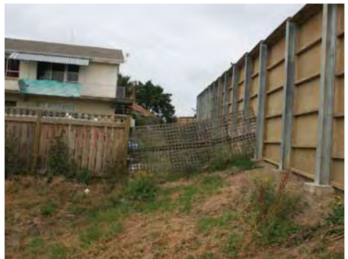
Figure 4.21 Placement of noise barriers back from property boundaries can lead to encroachment into road reserve, Auckland
