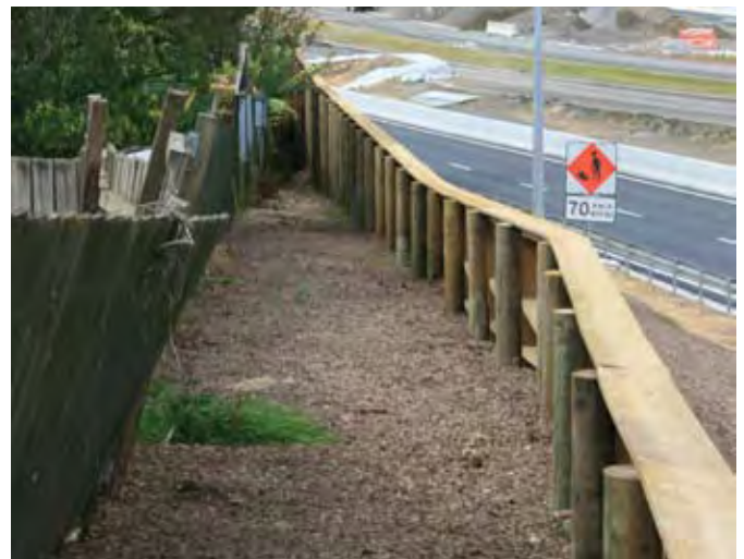
Figure 4.20 No mans land can be created when noise barriers are not placed on the boundary, Auckland
