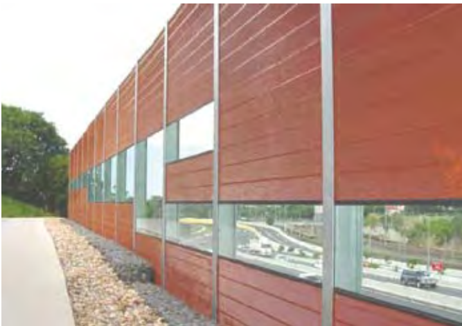
Figure 3.25 Transparent panels can give visual relief for pedestrians, Brisbane
