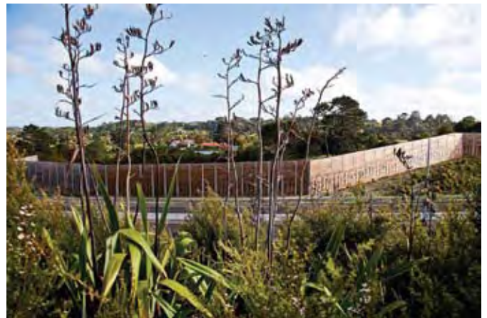
Figure 4.11 Noise barriers can be planted with native NZ species to enhance biodiversity, SH18, Auckland
