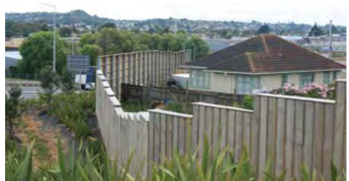
Figure 3.16 Poorly considered stepping is unattractive, Maoro Street, Auckland
