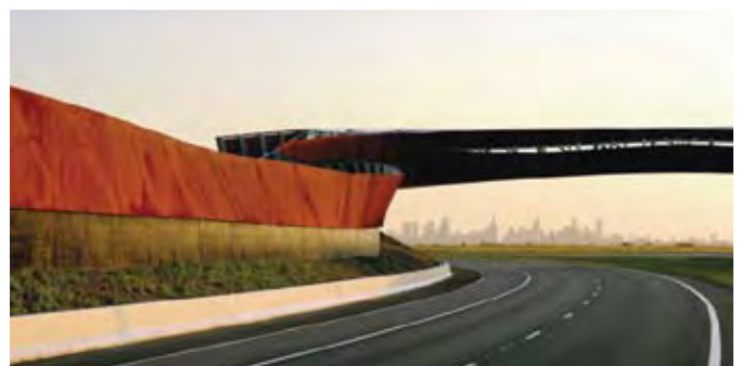
Figure 3.4 The design of the Craigieburn bypass noise barrier blurs the boundaries between function, sculptural features and a pedestrian bridge, creating a unified roadway experience, Melbourne
