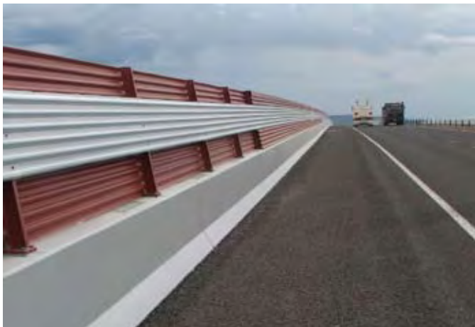
Figure 3.30 Corrugated iron panels attached to safety barrier with simple horizontal colours, Pakenham Bypass, Adelaide
