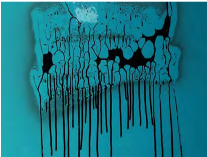
Figure 4.26 A paint repelling coating on the surface prevents paint from adhering properly (Source: SEI Chemicals)
