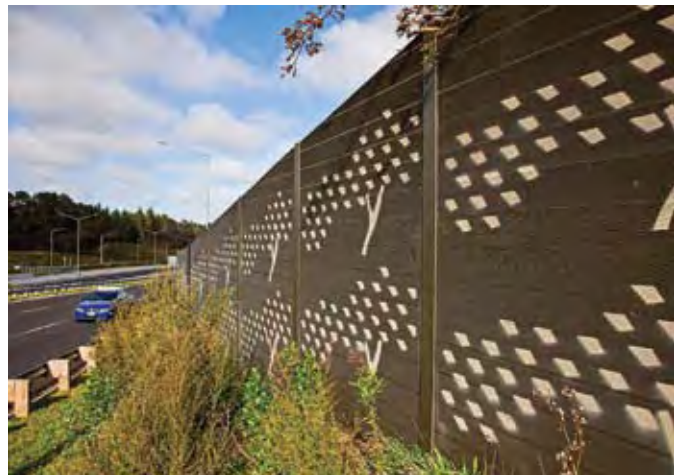
Figure 3.22 Visually appealing stencil designs on noise barriers can also act as an effective graffiti prevention measure, SH18, Hobsonville
