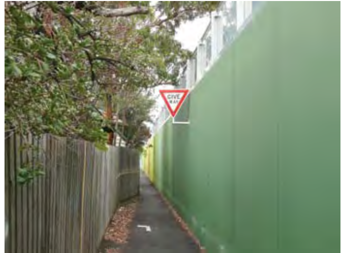
Figure 4.8 Noise barriers can create unsafe environments for the public where there are no clear sightlines, Tullamarine, Australia
