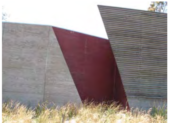
Figure 3.29 Timber noise barrier showing added design detail, Melbourne
