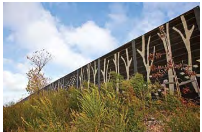
Figure 3.35 Noise barriers can play a large role in the overall landscaping of surrounding environments, SH18, Auckland
