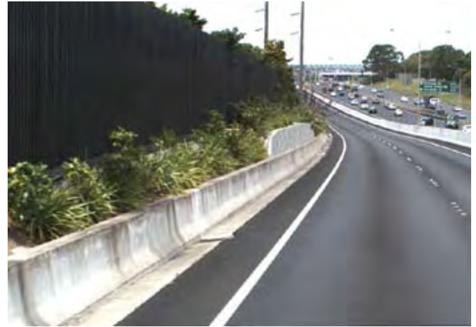
Figure 1.4 Noise barriers should provide effective noise relief as well as visually blending with the surrounding environment
