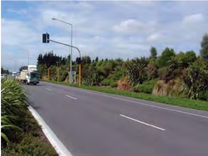
Figure 4.32 Earth bunds can make use of excess fill from road construction, Rolleston
