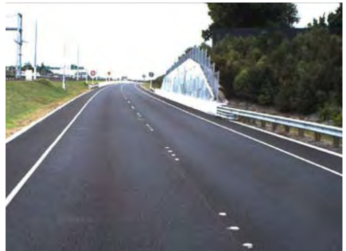
Figure 4.3 Retaining walls can be used to stabilise steeper slopes, SH1, Auckland
