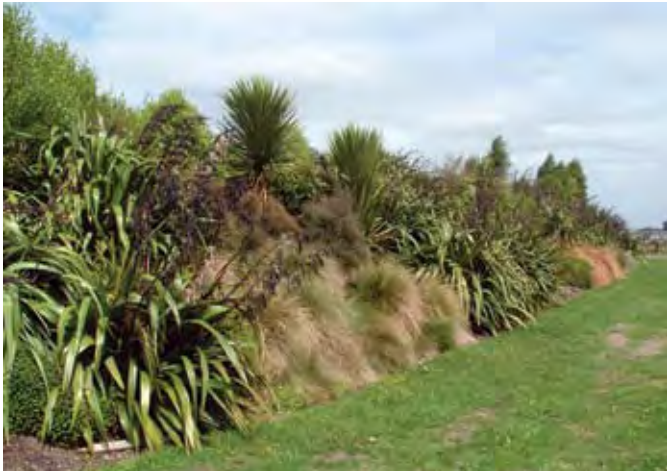
Figure 3.32 An earth bund planted with native plant species can be a good noise mitigation solution, SH1, Rolleston
