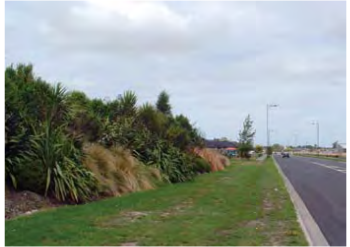
Figure 1.1 Earth bund, Rolleston
