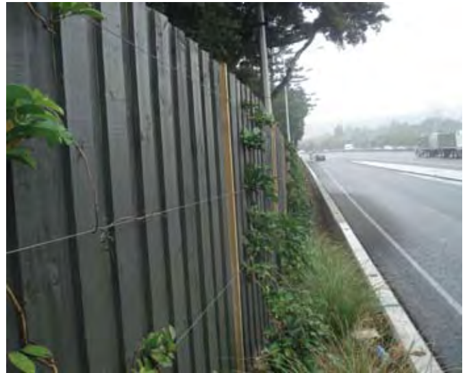
Figure 4.23 Climbing plants supported on wires can screen the wall surfaces and provide an organic and difficult face to graffiti, Hill Road, SH1, Auckland
