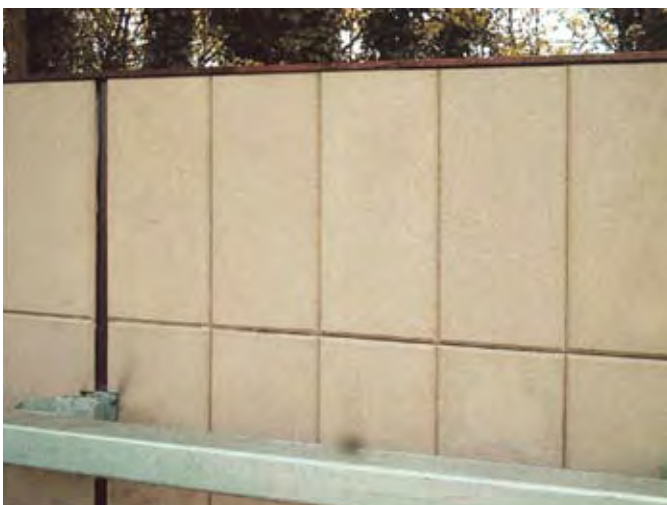
Figure 4.33 Absorptive porous concrete panels can be used to reduce sound reflection (Source: Forman Building Systems)
