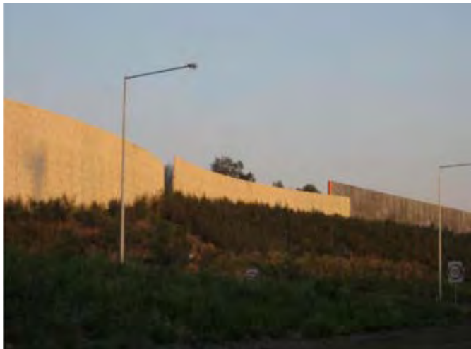
Figure 3.33 Noise walls can be located at the top of an earth bund, Melbourne
