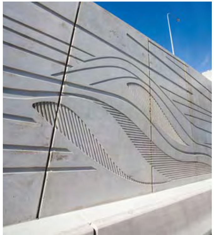
Figure 4.6 Noise barriers can be integrated with safety barriers, SH20 Mt Roskill Extension, Auckland
