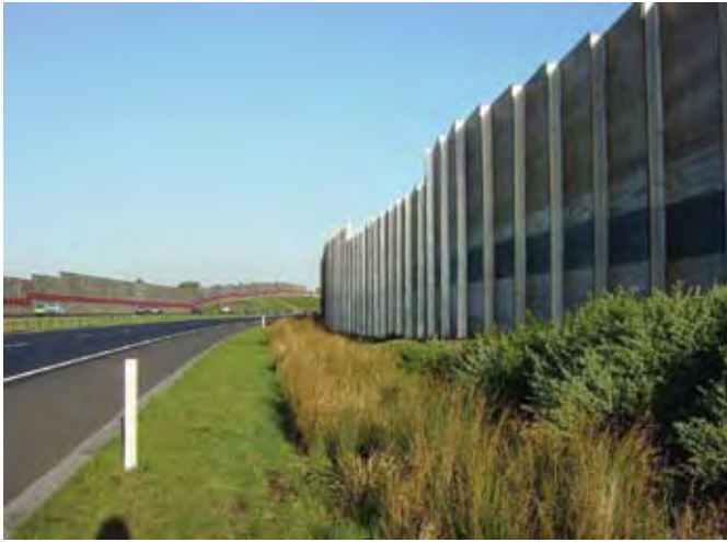
Figure 4.5 Swales can provide a stormwater solution next to a noise barrier
