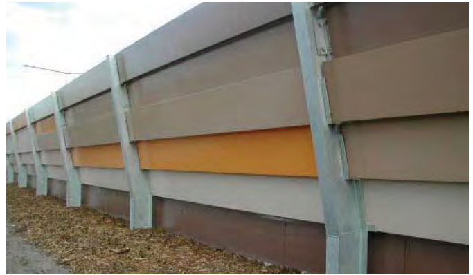
Figure 3.7 Angled noise barrier, Melbourne
