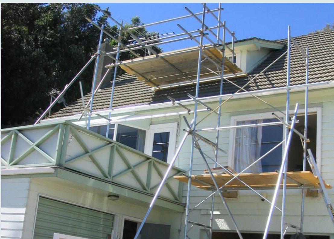
FIGURE 52: GLAZING UPGRADE WORKS IN PROGRESS
