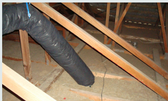
FIGURE 43: DUCTWORK PROVIDING ACOUSTIC ATTENUATION
