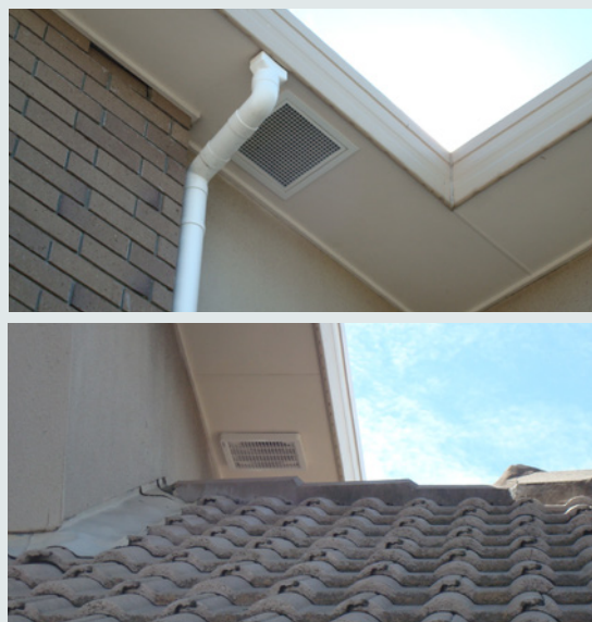
FIGURE 43: DUCTWORK PROVIDING ACOUSTIC ATTENUATION
