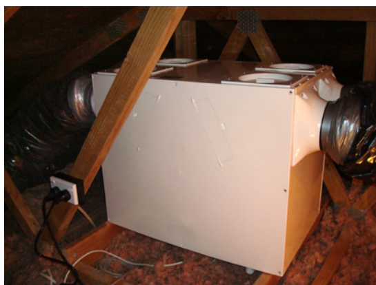
FIGURE 35: HEAT RECOVERY UNIT
