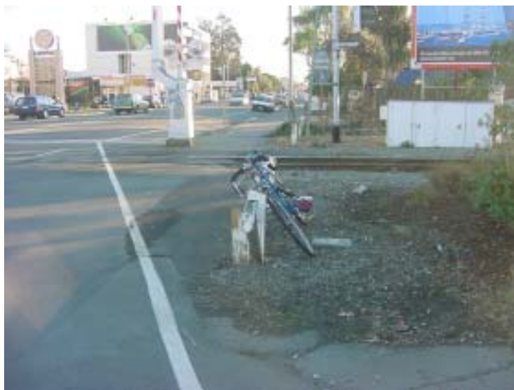
View looking west showing the pedestrian/vehicle conflict area where the footpath terminates and the roadside barrier.
