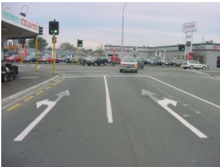
Example of redundant markings that are still visible – Clyde Road
