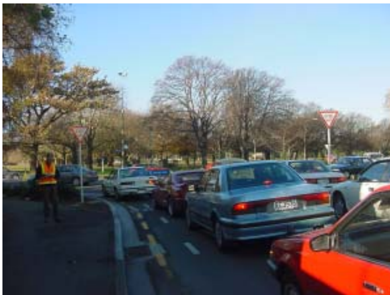
View looking east, on the approach to Deans Avenue Roundabout, showing an inadequate cycle lane. Note position of sump grate.
