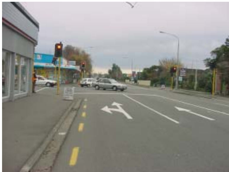
Looking west on approach to Wharenui Road intersection - Note two through lanes
