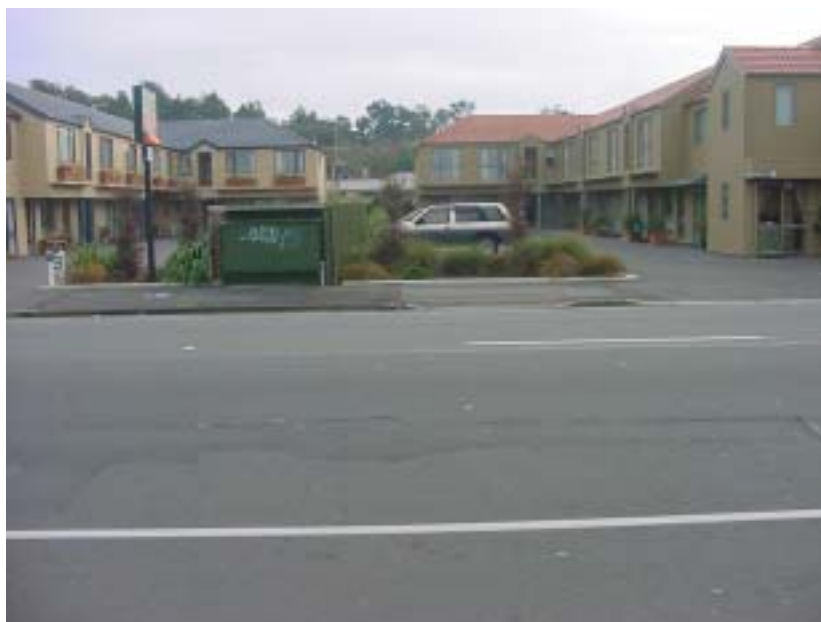
Suggested Pedestrian crossing point location adjacent No 140 on the north side of Riccarton Road
