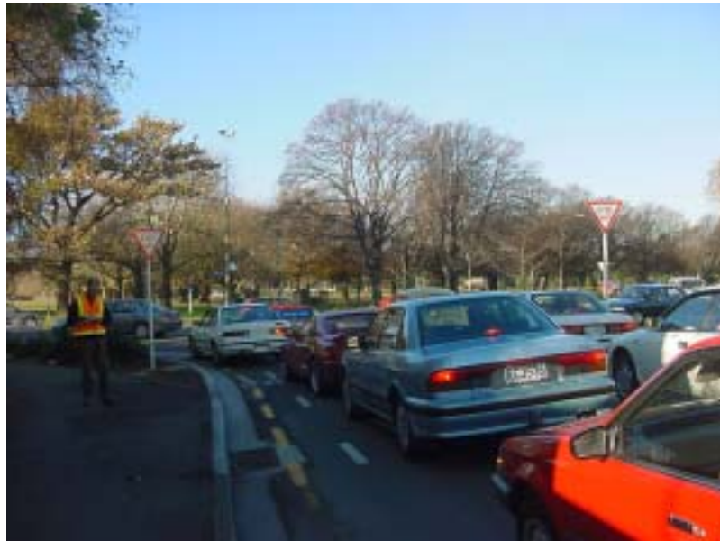
View looking east, on the approach to Deans Avenue Roundabout, showing an inadequate cycle lane. Note position of sump grate.
