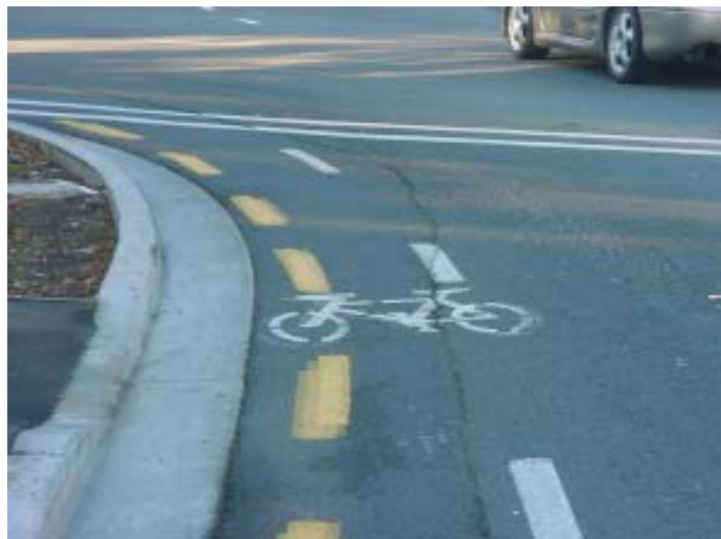
Close up, showing narrow cycle lane and cycle marking extending into live lane
