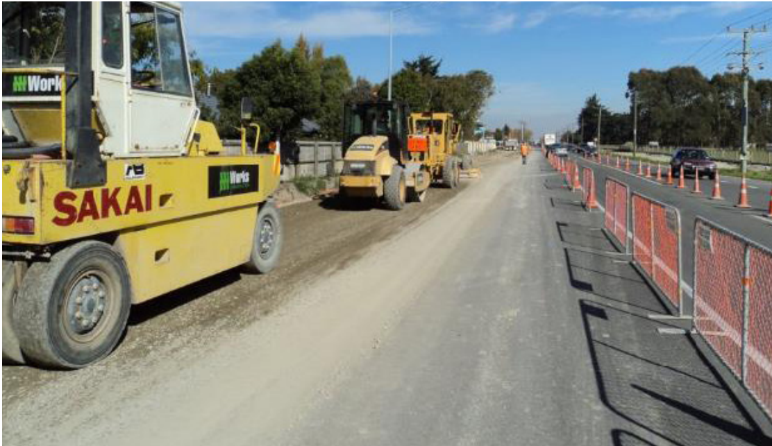
Works adjacent residences
