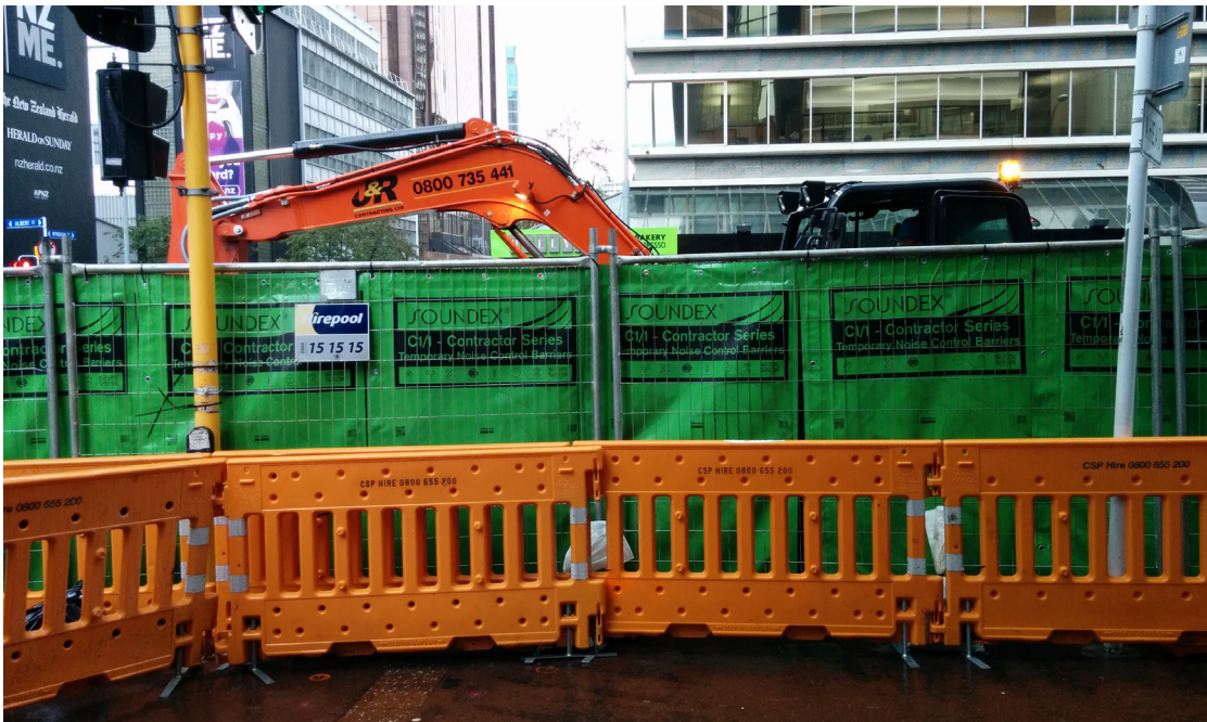
Temporary noise barriers
