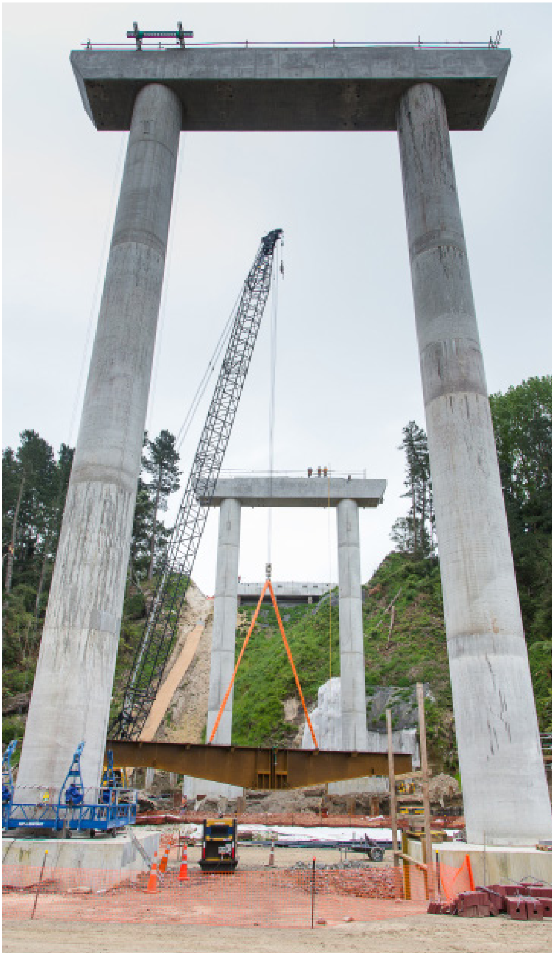
Bridge beam installation. Waikato Expressway
