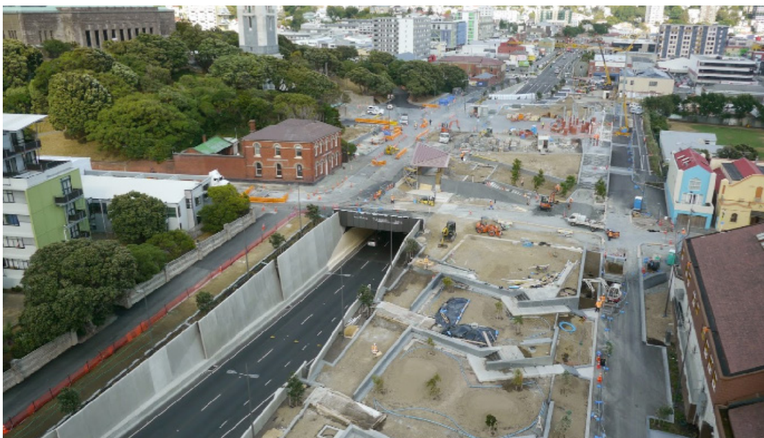
Arras Tunnel, Wellington
