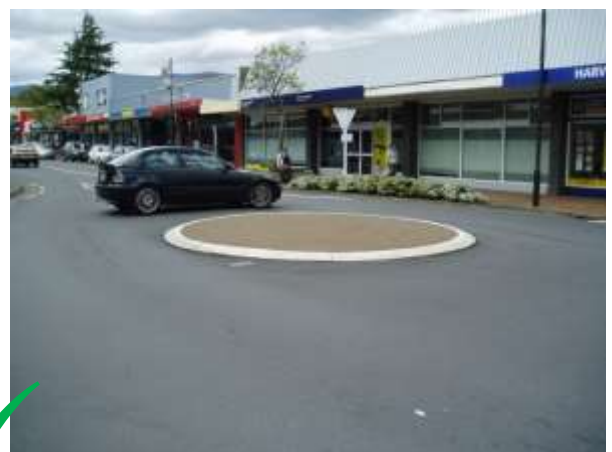
Low profile roundabouts and kerbs can cause loss of control crashes for motorcycles and scooters
