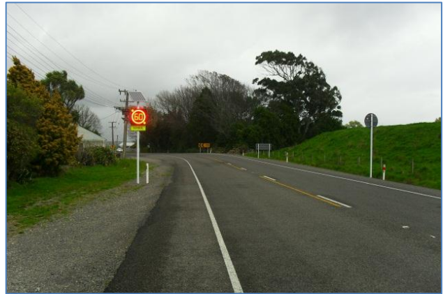
Figure 17 (i&ii) 60km/hr LED Mandatory Speed Sign Installed - Left: Northbound, Right: Southbound
