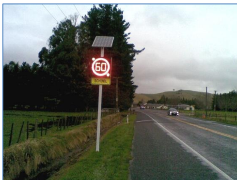
Figure 19 (i) 60km/hr LED Mandatory Speed Sign Installed - Southbound
