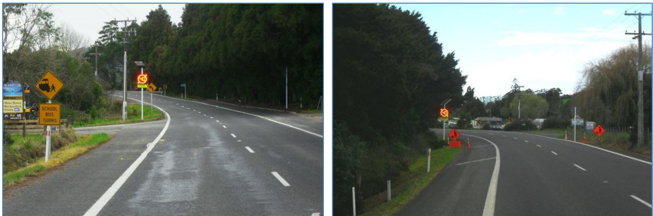
Figure 25 (i&ii) 40km/hr LED Mandatory Speed Sign Installed - Left: Northbound, Right: Southbound
