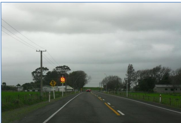
Figure 17 (i&ii) 60km/hr LED Mandatory Speed Sign Installed - Left: Northbound, Right: Southbound
