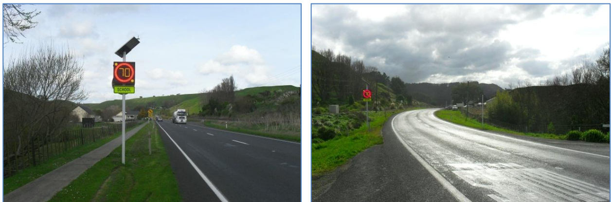
Figure 15 70km/hr LED Mandatory Speed Sign Installed - Left: Eastbound, Right: Westbound
