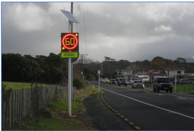
Figure 22 (i&ii) 60km/hr LED Mandatory Speed Sign Installed - Left: Westbound, Right: Eastbound
