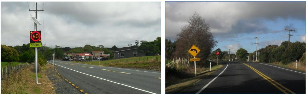
**Figure 22 (i&ii) 60km/h LED Mandatory Speed Sign Installed - Left: Westbound, Right: Eastbound**
