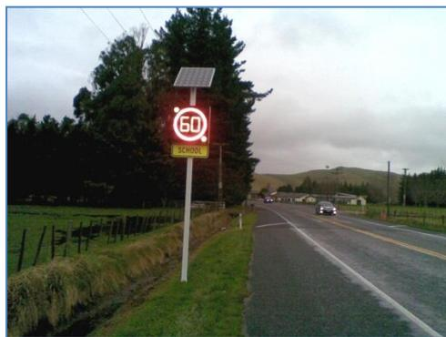
Figure 19 60km/h LED Mandatory Speed Sign Installed - Southbound
