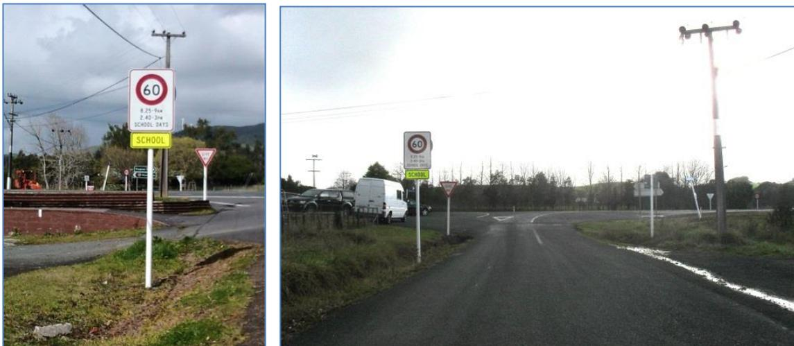
**Figure 23 (i&ii) Te Uku School - Side Road Warning Signs on Okete Rd (left) and Matakotea Road (right).**
