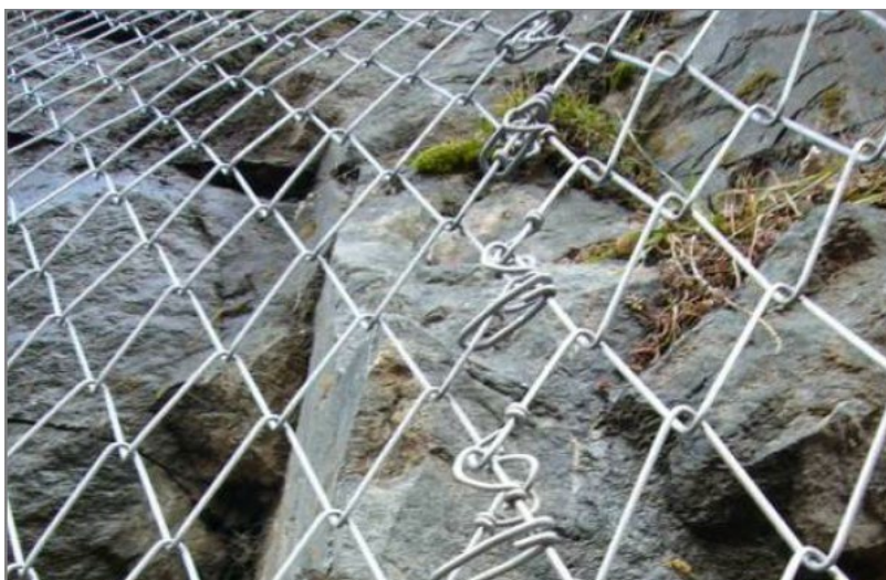
Image 6: Diamond Mesh, for example Geobruugg Tecco (Geobruugg, 2009)
