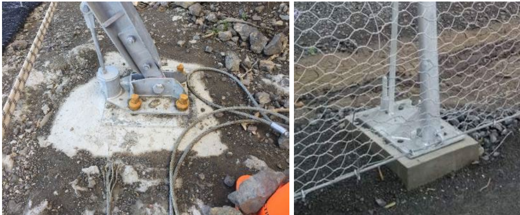
Image 9: A hinged post (left), a fixed post (right)
