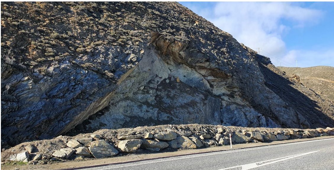
Image 12: An earth bund constructed from site won material
