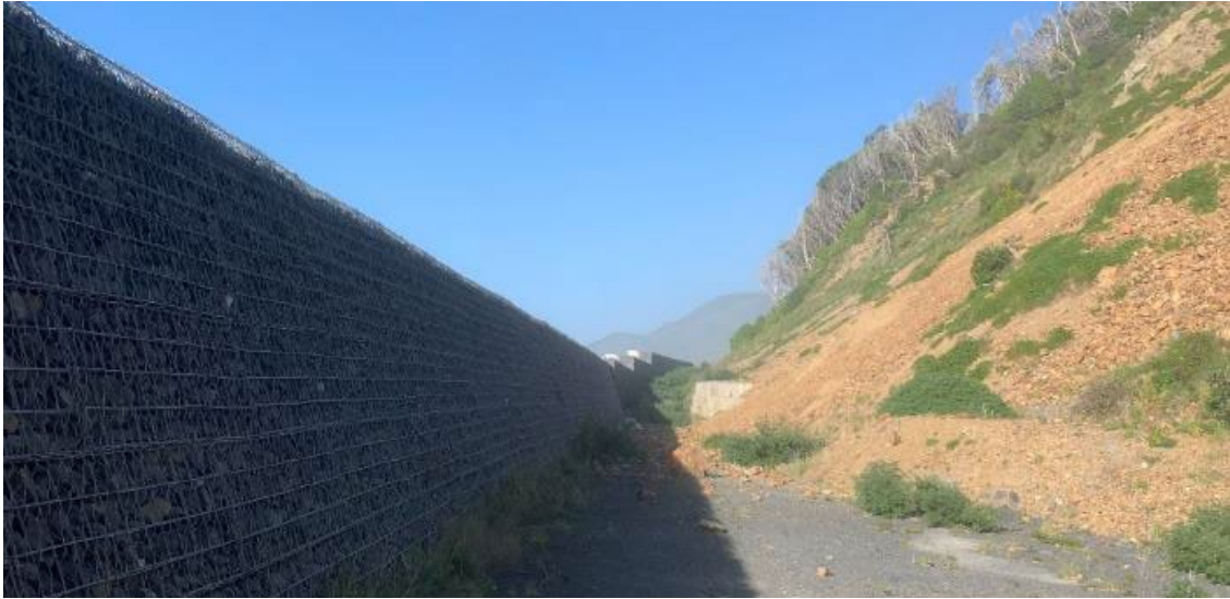
Image 11: A reinforced bund at the base of a slope
