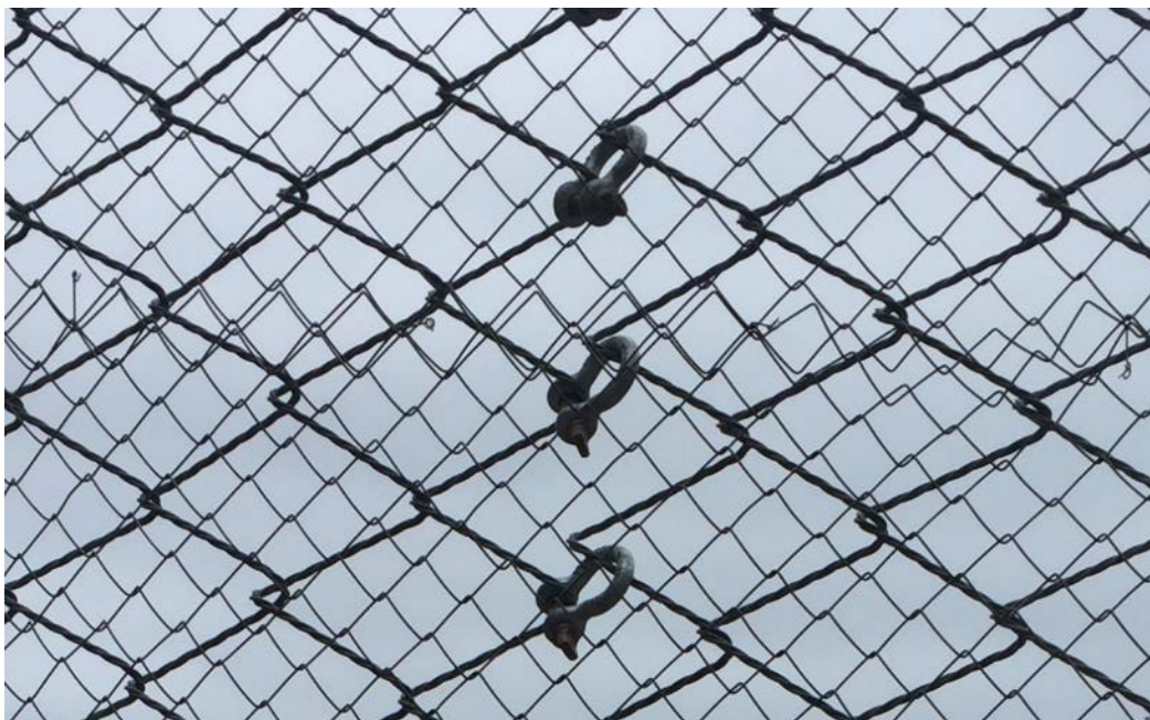
Image 5: Shackles used to connect two mesh panels.
