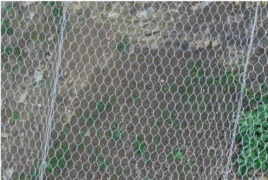
Image 7: Double Twist Mesh, for example Maccaferri DT Mesh
