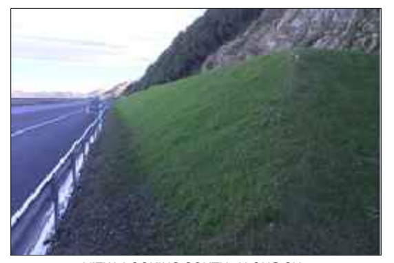
VIEW LOOKING SOUTH ALONG SH1 (1V:2H SECTION)
