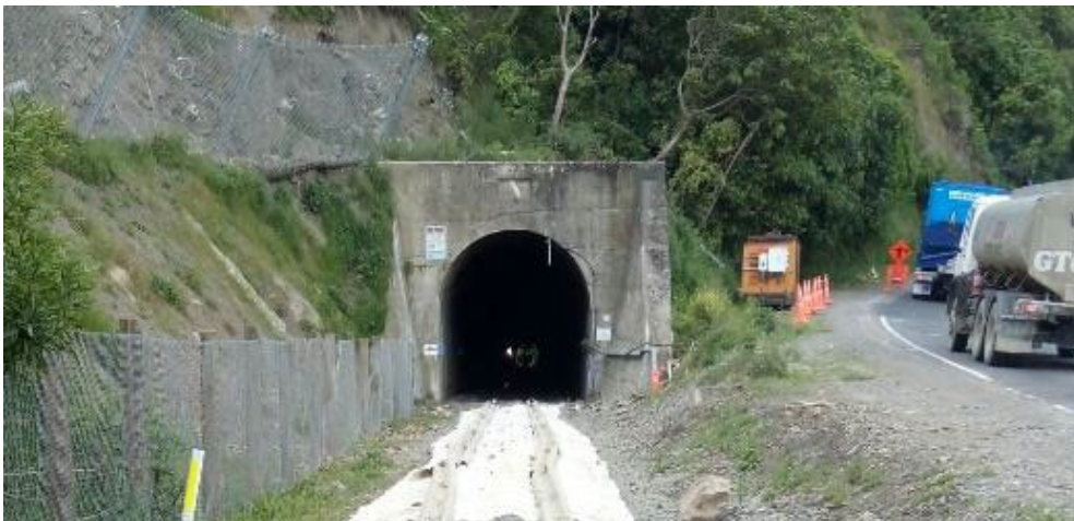
Image 4: An example of rail ballast contamination protection, to protect a third-party asset.
