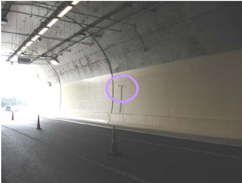
Figure 8: Location of the inlet for the continuous CO and NO 2 monitoring
