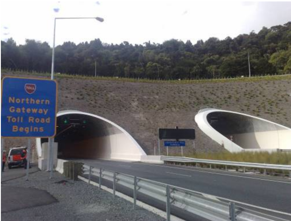
Figure 3: View of the Johnstone's Hill Twin Tunnels from the northern end
