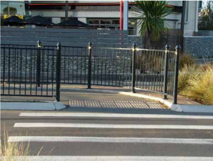
Photo 5.10: Example of a staggered median crossing with marked pedestrian crossing over the traffic lanes, (note: the barrier contrast could be better) (Photo: Tim Hughes).
