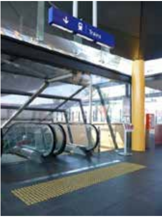
Photo 5.25: TGSIs at escalators (Photo: Michael Brown)
