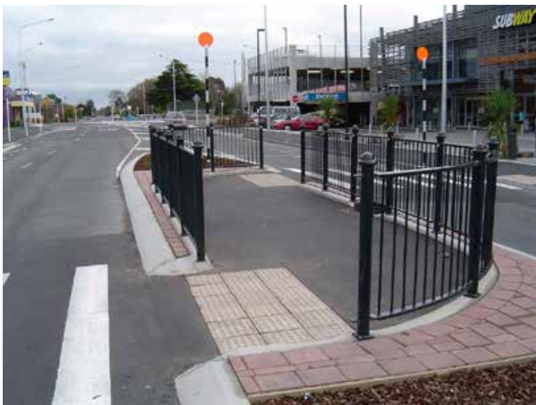
Photo 5.11: The kerb and fencing provides tactile cues within the staggered median to assist pedestrians who are blind or have low vision, so there is no need for directional indicators. (Photo: Tim Hughes).
