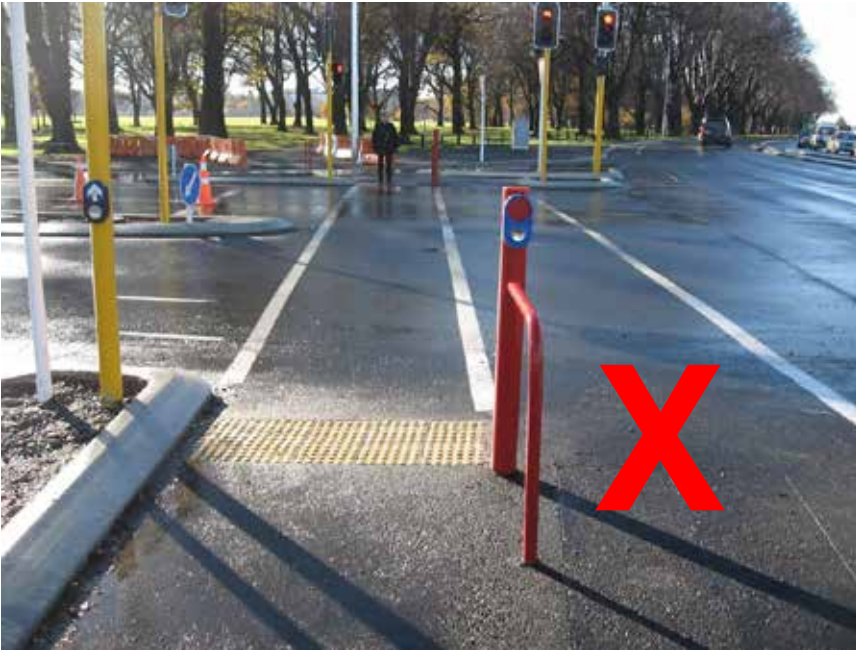
Photo 5.19: The TGSIs at this signalised pedestrian and cyclist crossing are installed across the pedestrian area only. The TGSIs should extend across the entire facility to ensure that a person who is blind or has low vision receives tactile warning if they mistakenly enter the cyclist crossing area.
