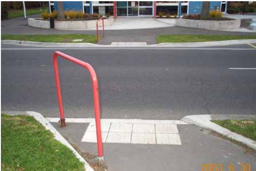
Photo 5.9: The warning indicators are aligned with the road crossing direction. (Note: not quite full width) (Photo: Susan Cambridge)
