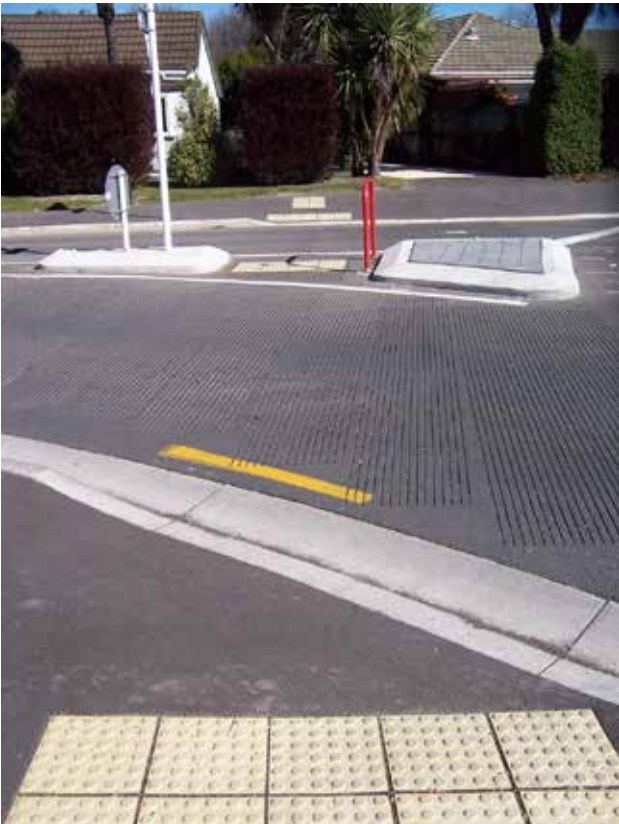
Photo 5.14: Actual example of the TGS layout shown in Figure 5.13 (Photo: Tim Hughes)
