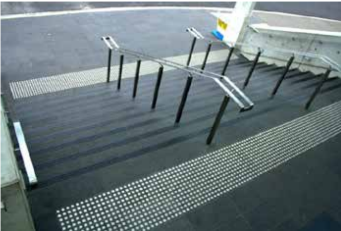
Photo 5.24: Example of TGS at the top and bottom of stairs (Photo: Michael Brown)
