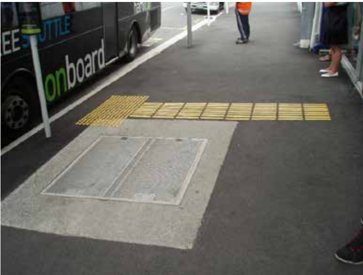
Photo 5.22: Directional indicators lead to warning indicators at a bus stop (Photo: Michael Brown).
