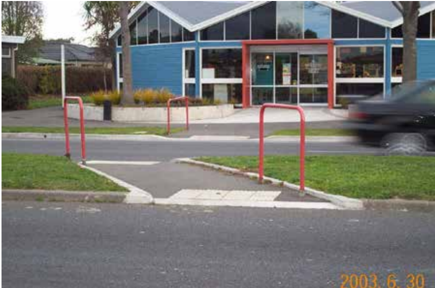
Photo 5.8: On deep medians, two sets of warning indicators are installed. (Note: not quite full width.) (Photo: Susan Cambridge)
