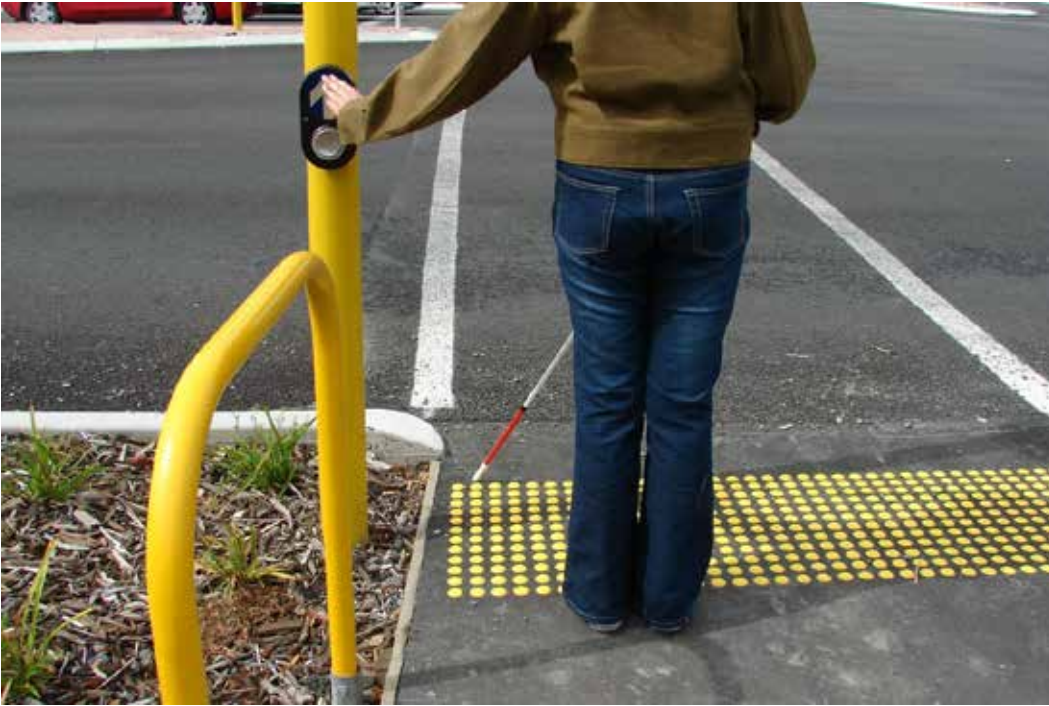
Photo 5.1: View of warning indicators. Note how the domes have been located to maintain equal spacing between domes across the entire warning indicator surface. (Photo: Carina Duke)
