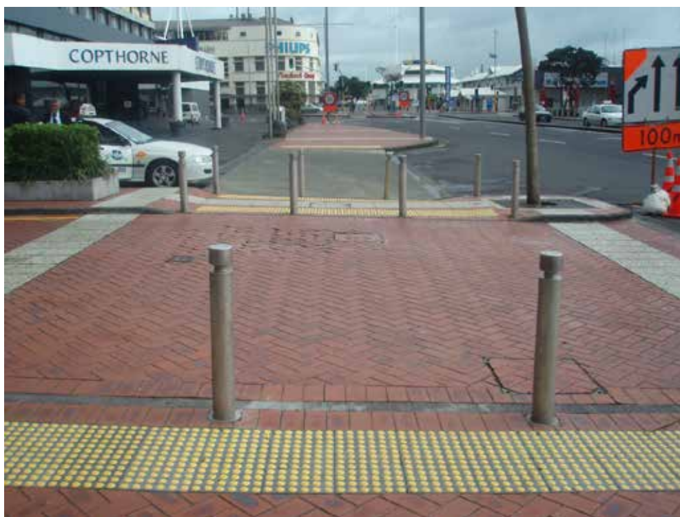
Photo 5.23: Warning indicators extend across the full width of the footpath outside a busy car park building (Photo: Michael Brown).
