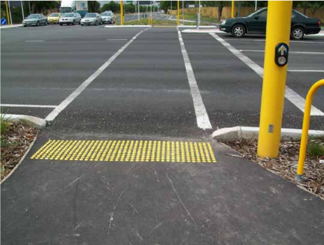
Photo 5.13. This installation is an example of “Best Practice” with the warning TGS and pedestrian call box both aligned with the crossing direction. The gap between the TGS and signal pole is so small that a person cannot inadvertently enter the road without receiving tactile warning. (Photo: Carina Duke)
