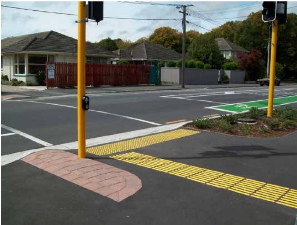
Photo 5.6: These directional indicators intercept all pedestrians on the continuous accessible path of travel. They lead directly to the warning indicators, and aligned for the use of the pedestrian push button. (Photo: Carina Duke).
