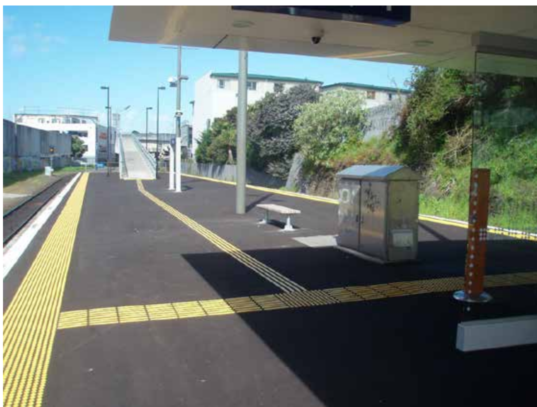
Photo 5.4: The warning indicators at this railway station are 600mm deep and set 600mm back from the platform edge (Photo: Michael Brown)
