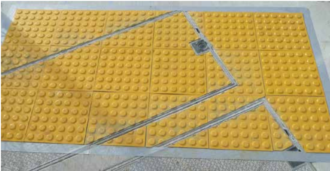
Photo 5.18: An example of how warning TSGI can be integrated into the design of utility service cover (Photo: Michael Brown).
