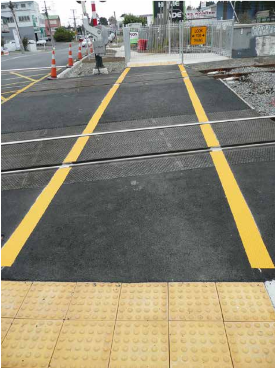
Photo 5.17: Tactile arrangement at a rail crossing (Photo: Michael Brown)
