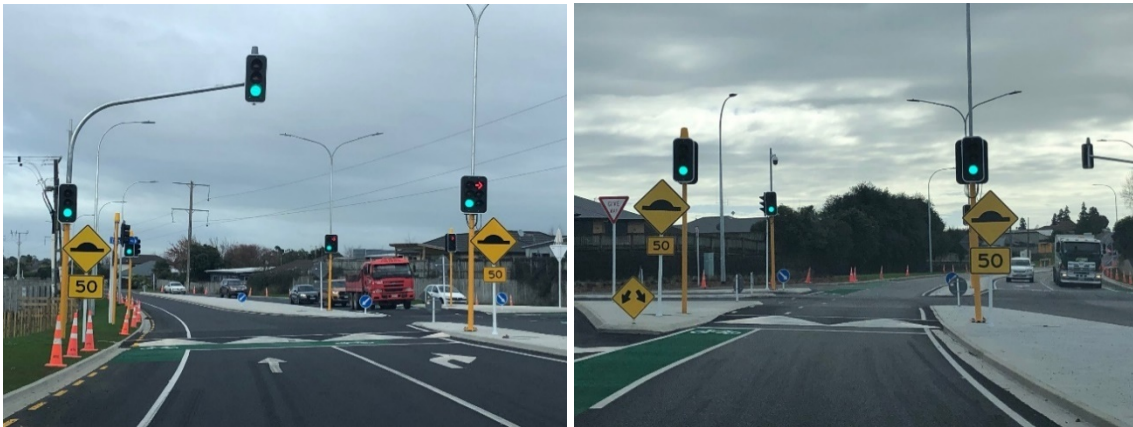
Figure 1 Example of RSP's at a new signalised intersection (Thomas Road / Gordonton Road, Hamilton)
