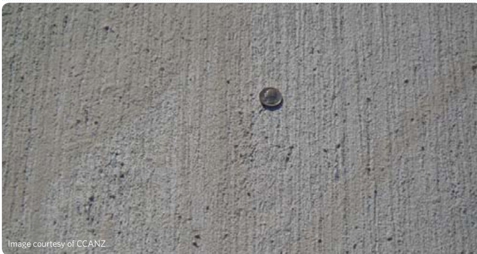
FIGURE 2.52 Diamond grinding
