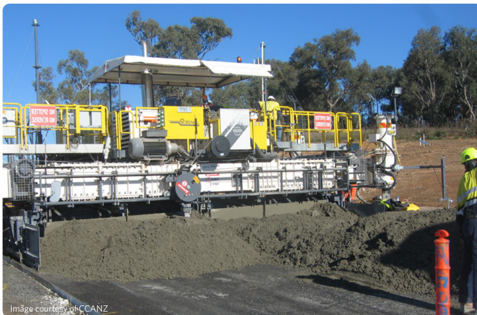
FIGURE 2.47 | Continuous concrete road construction using a slipformer
