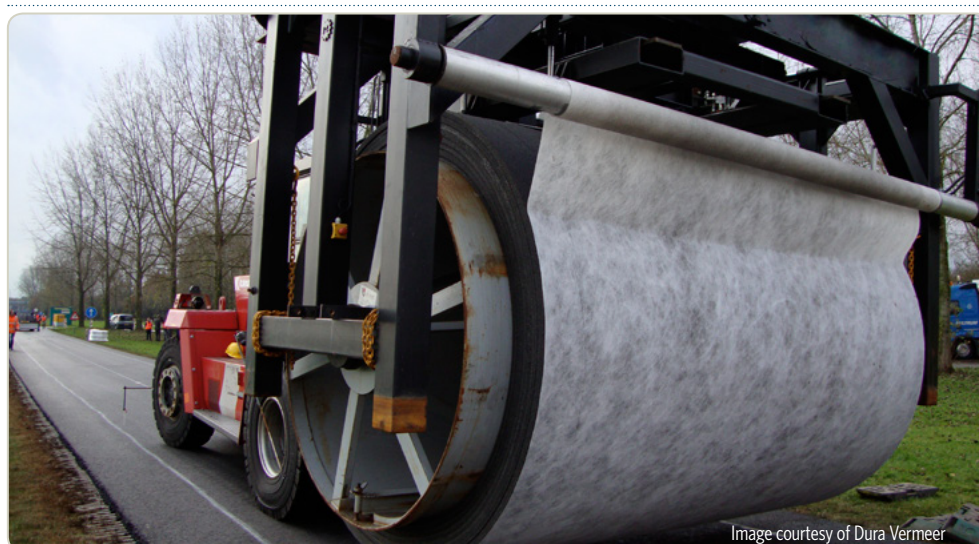
FIGURE 2.46 Laying of PERS
