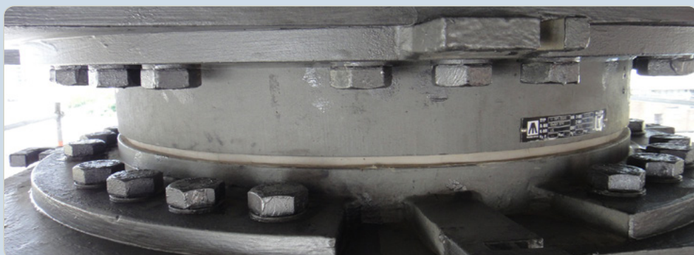
FIGURE 3.9 | Newmarket viaduct bridge bearing
