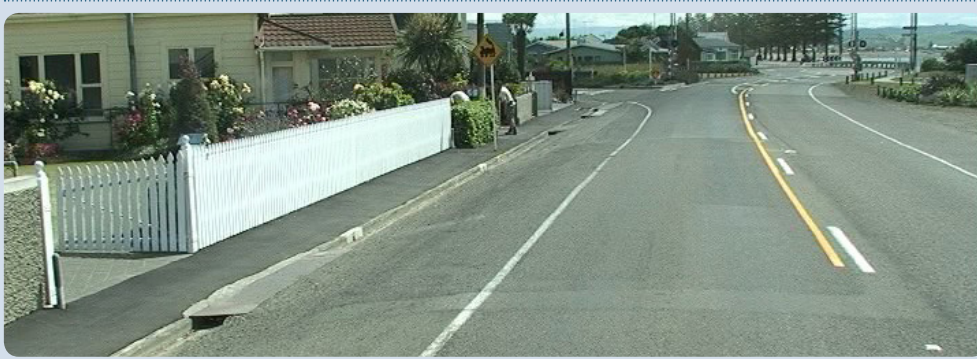
FIGURE 2.37 Breakwater Road with initial maintenance work completed
