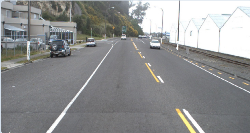
FIGURE 2.24 SH50 after 2008 resurfacing (house on hill to left above photograph)
