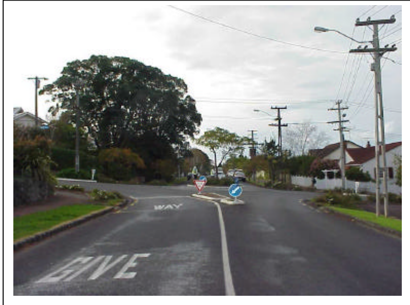
Photograph 13 : Low poorly defined and ineffective collar. Traffic travels straight through over collar with no deflection. The primary Give Way should be on the left at full mounting height
