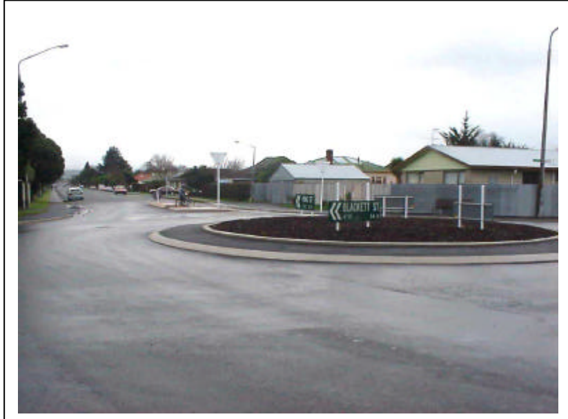
Photograph 3 : Good bold street name/chevron sign. Note cyclist using cut down on splitter island.
