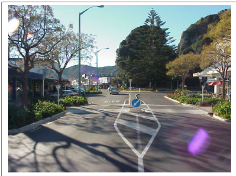
Photograph 12 : Pedestrian crossing point well back from roundabout. Note the give way signs for pedestrians.
