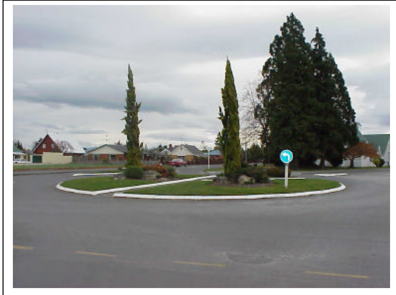
Photograph 9 : Old roundabout with pedestrian paths through central island and inappropriate use of mandatory turn left sign.
