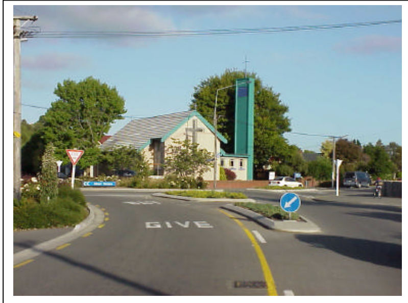
Photograph 7: Deflection by approach alignment and splitter island.
