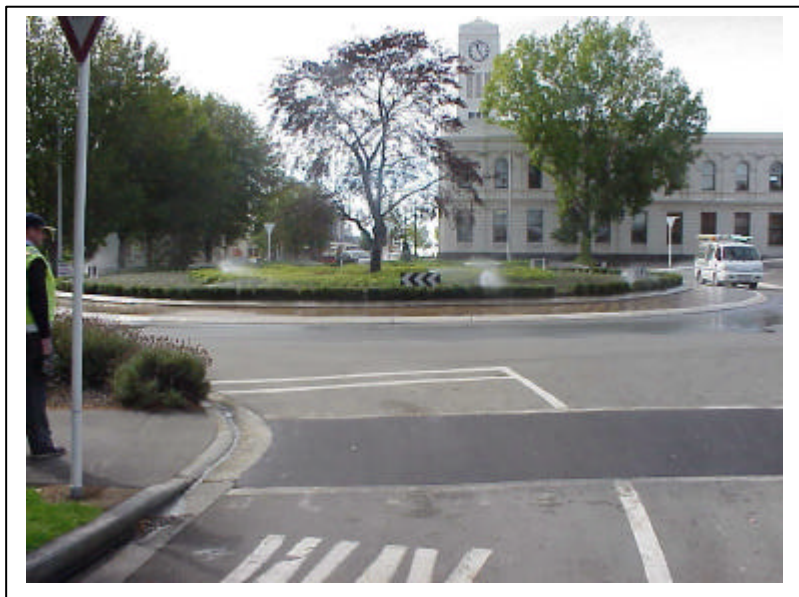
Photograph 10 : Paving removed from pedestrian crossing point to avoid matching paved collar.
