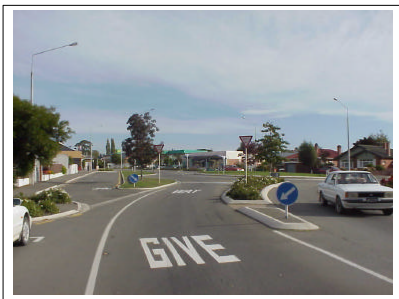
Photograph 6: Deflection by approach alignment. Service road to properties on the left. Note incorrect use of keep left RG17 sign.
