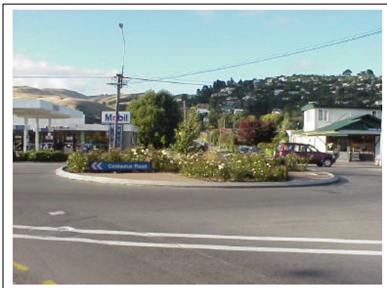
Photograph 1: Standard roundabout. Quadrant paving/landscaping for good visibility of street name/chevron sign.
