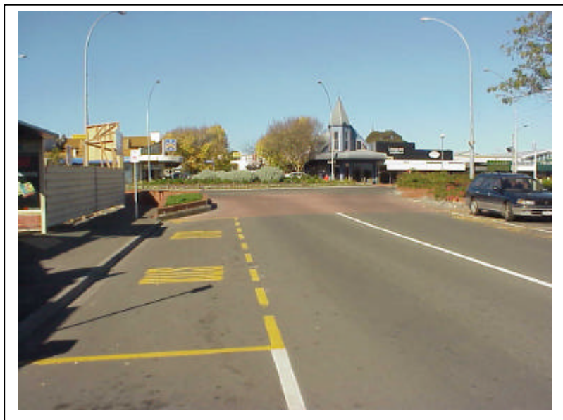
Photograph 8 : Large central island roundabout. Island and speed humps force low operating speed. Constructed in 1980. Not to current standards but works well with low speeds.
