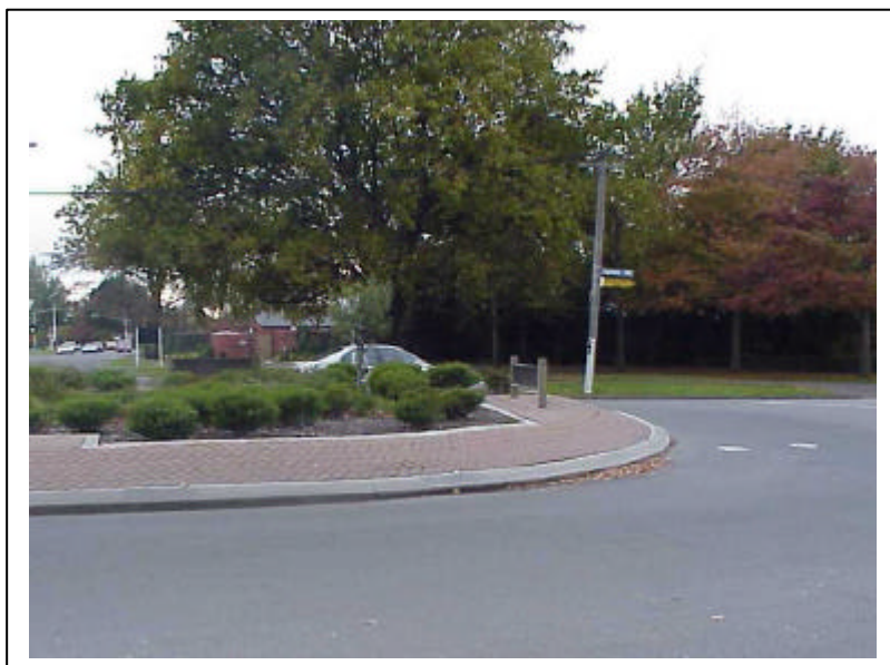
Photograph 14 : Walled roundabout but badly located pole (with hazard marker) on exit.
