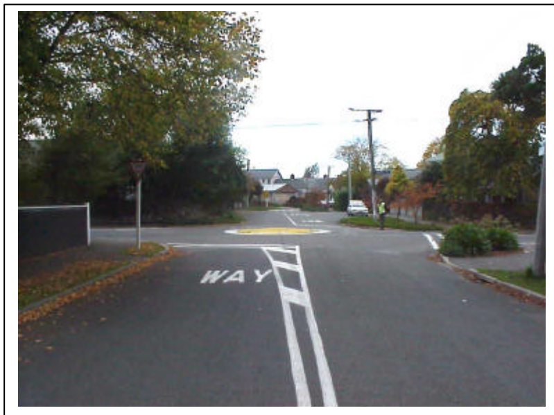
Photograph 5: Dome roundabout on local roads with other traffic calming (note speed hump in background) Beware of vegetation growth obscuring signs
