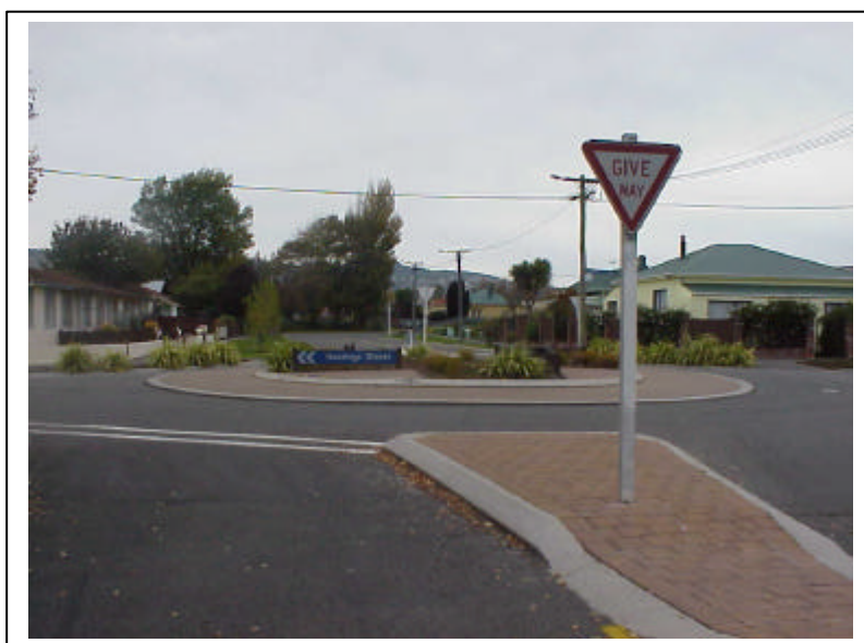
Photograph 2: Collared roundabout. Quadrant paving/landscaping for good visibility of street name/chevron sign.
