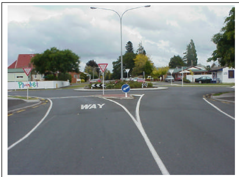
Photograph 4: Good collared roundabout with good deflection. Typical chevron sign.
