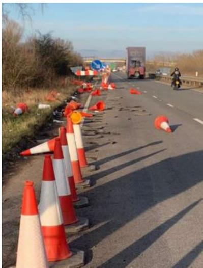
The TTM involved three permanent lane closures to increase the working area. HRS Intellicone Smart Taper was used as an enhanced safety measure. This provides immediate digital notification of any strike. The metric for determining success was time to reinstatement compared to time to reinstatement without the smart cones.
