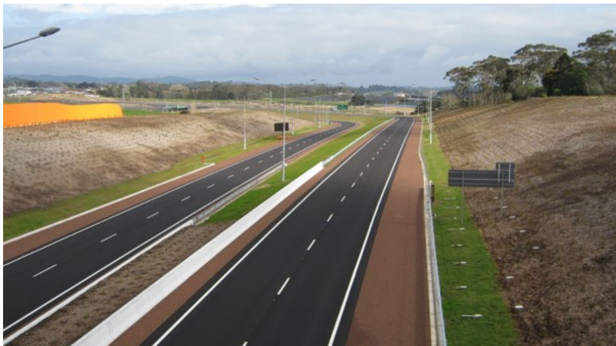
Figure 3.3 Hobsonville section of SH18 looking west from Trig Road interchange, showing orange noise wall, extensive lighting, and native planting into mulched, re-contoured and earthworked areas. 61 (Photo taken in 2011.)
