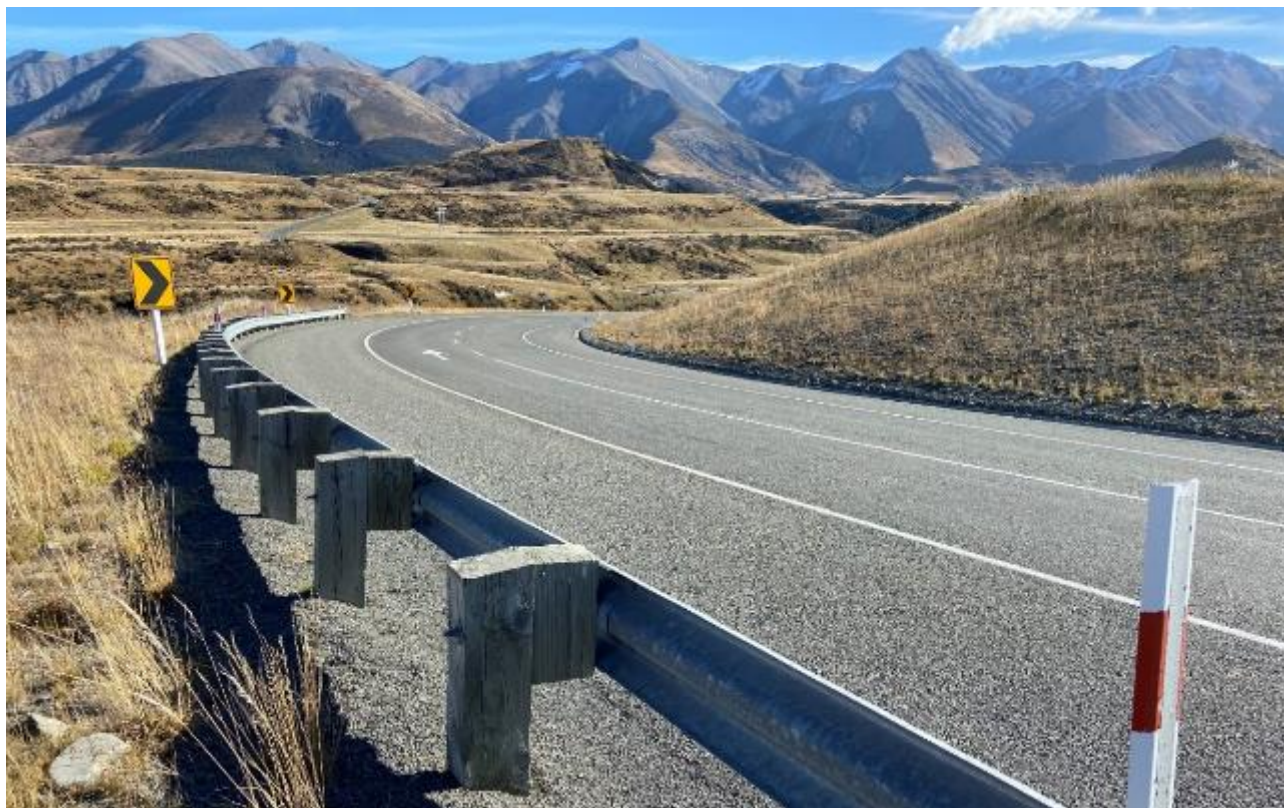
Figure 4.5 The Great Alpine Highway looking towards Castle Hill from Cave Stream Reserve. Here the road passes through extensively grazed farmland. Large road cuts create sparsely vegetated slopes (right). (Photo taken April 2021.)
