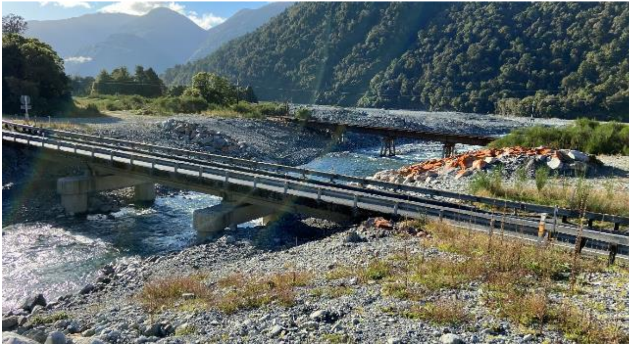
Figure 2.15 Co-location of linear infrastructure can concentrate impacts, generally leading to better ecological outcomes than separating them across landscapes, as shown here where riverbed and banks needed to be heavily modified to protect SH73 and rail bridges from flood damage. (Photo taken April 2021.)
