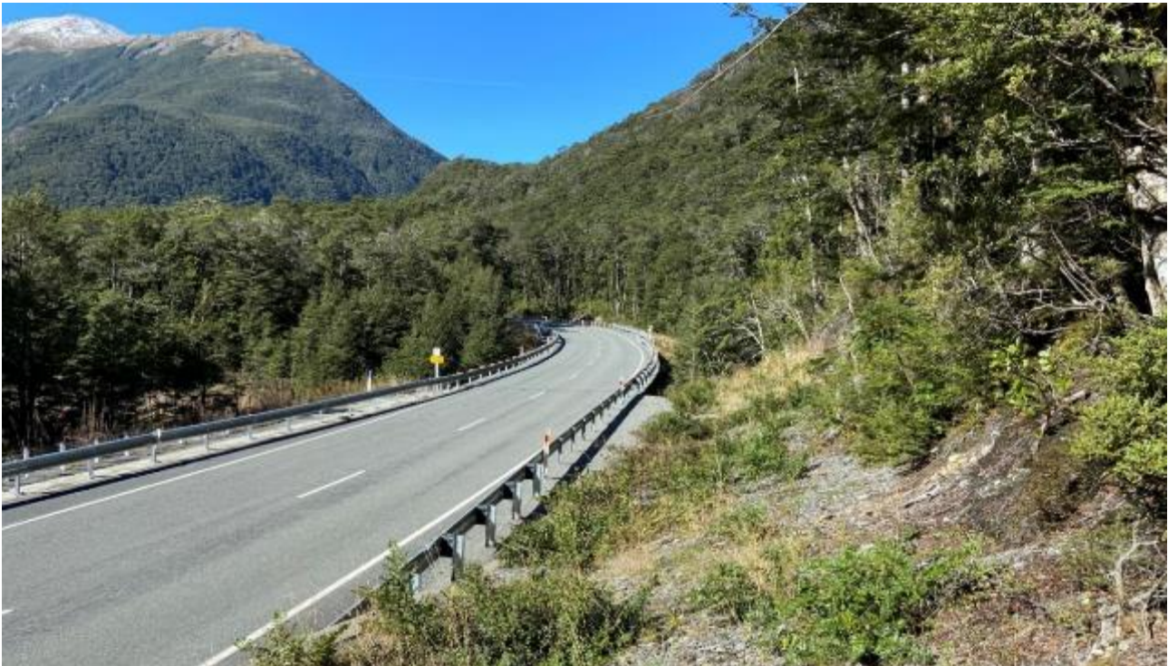
Figure 4.24 New bridge and road construction that minimises impacts of fragmentation and weed invasion with forest generally retained close to the road edge. Tutu and beech seedlings are naturally establishing along the exposed edge (foreground). (Mingha Bluff realignment; photo taken April 2021; the bridge is also shown in Figure 4.17.)
