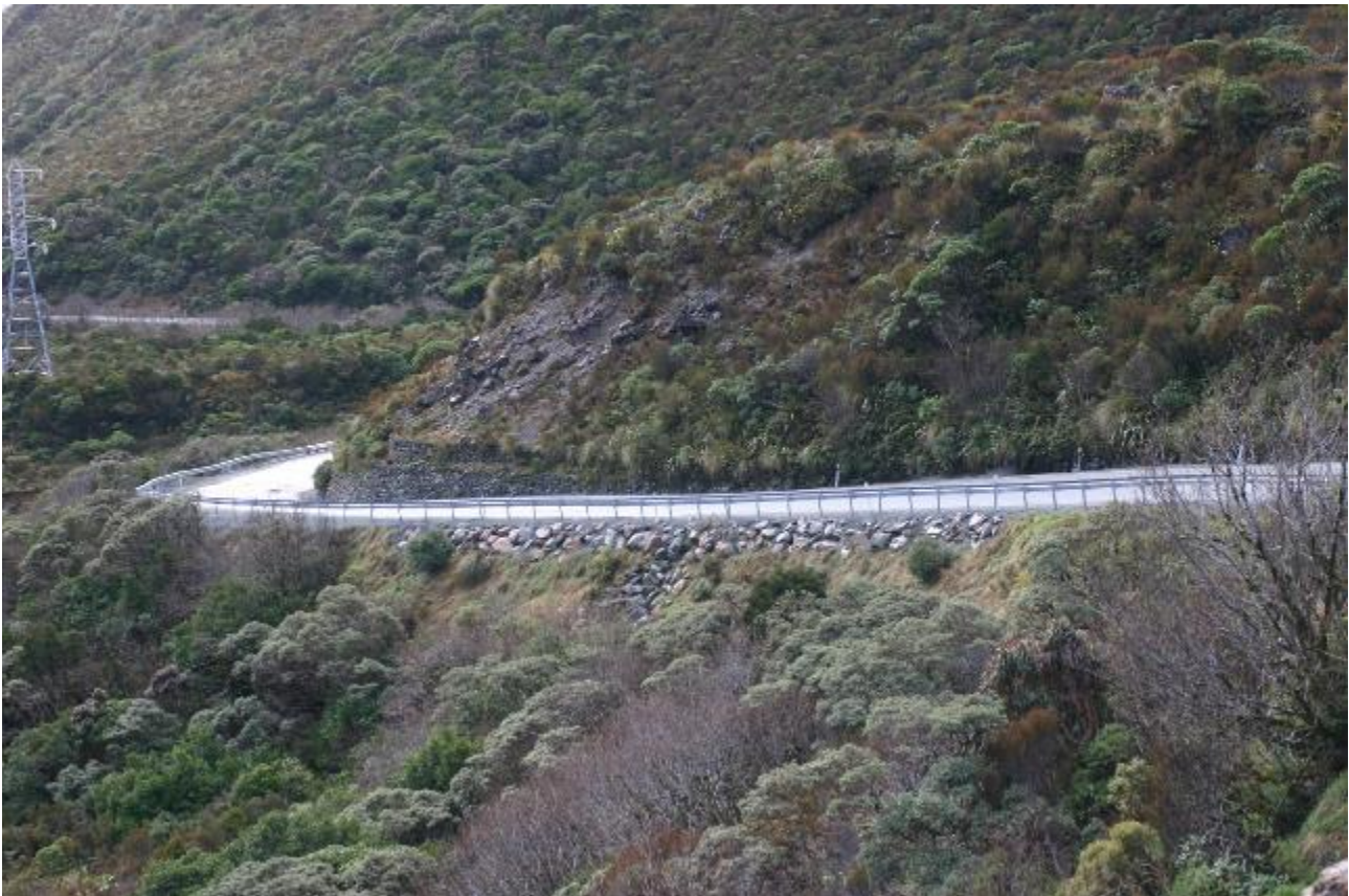
Figure 4.23 Fragmentation and edge effects of SH73 in alpine shrubland is limited by constraining the non-vegetated area using narrow lanes with safety barriers and retaining walls. (Photo taken July 2013.)
