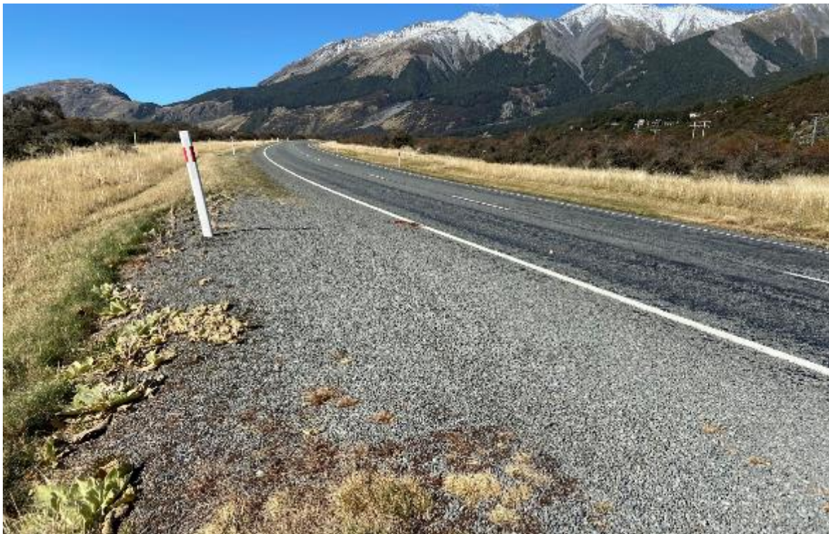
Figure 2.18 Use of herbicide to maintain a ‘vegetation clear zone’ around marker posts has created bare strips ~6–10 m long (the specification is minimum 3 m). These allow more aggressive species to establish that may have greater potential to invade adjacent natural habitats than the browntop grasses that otherwise cover the ground in mown areas. (Photo taken April 2021.)
