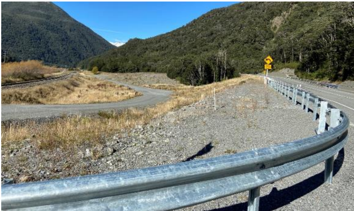
Figure 2.19 A large area beside the railway used during construction of the new highway to store resources and excavated gravels creates a very wide but localised zone of impact that is partly naturally revegetating but vulnerable to invasion from weeds such as broom and Russell lupin. (Photo taken April 2021.)
