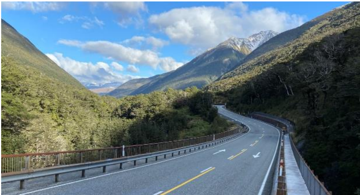
Figure 4.2 Near the summit of SH73 looking down towards Arthur’s Pass Village. This section is a barrier to pest plants as the native vegetation is dense and road design minimises exposed soil or gravel by placing edge marker posts on barriers, using concrete dish drains rather than gravel drains, and using retaining walls to minimise the disturbance footprint. (Photo taken April 2021.)
