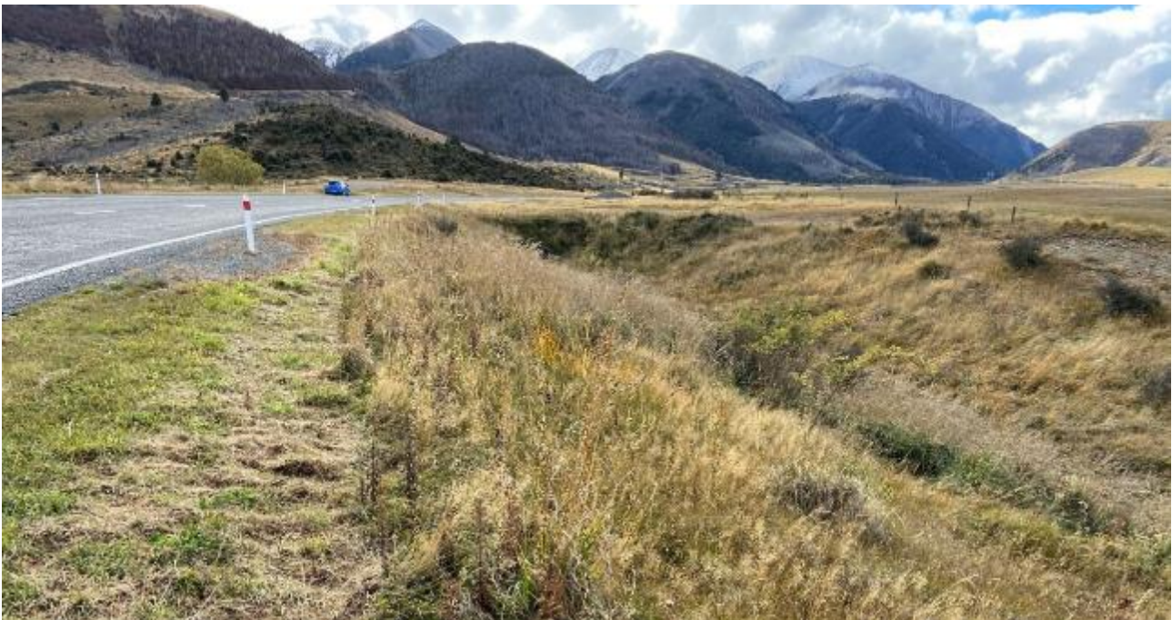
Figure 2.22 The inside of a curve on SH73 creates a large area crossing a shallow gully that is not grazed and includes a small wetland. This is an opportunity to create a biodiversity 'node' or steppingstone across a farmed valley floor where adjacent pasture has low biodiversity values. (Photo taken April 2021.)
