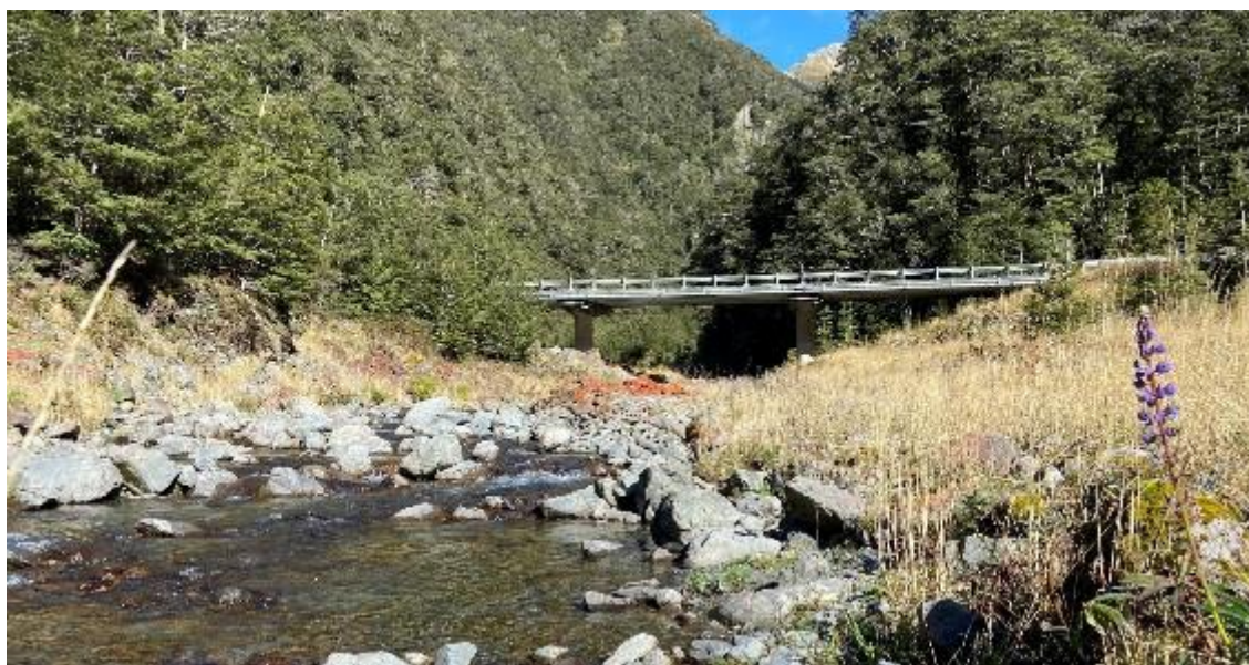
Figure 4.17 Bridge in Arthur's Pass National Park. The bridge has a low impact – its piers are set back from the river, so they do not impact the bed; its narrow width minimises shading; and road runoff discharges to permeable gravels. See Figure 4.24 for a 'road view' of the bridge. Russell lupin (right foreground) spreads downstream. (Photo taken April 2021.)
