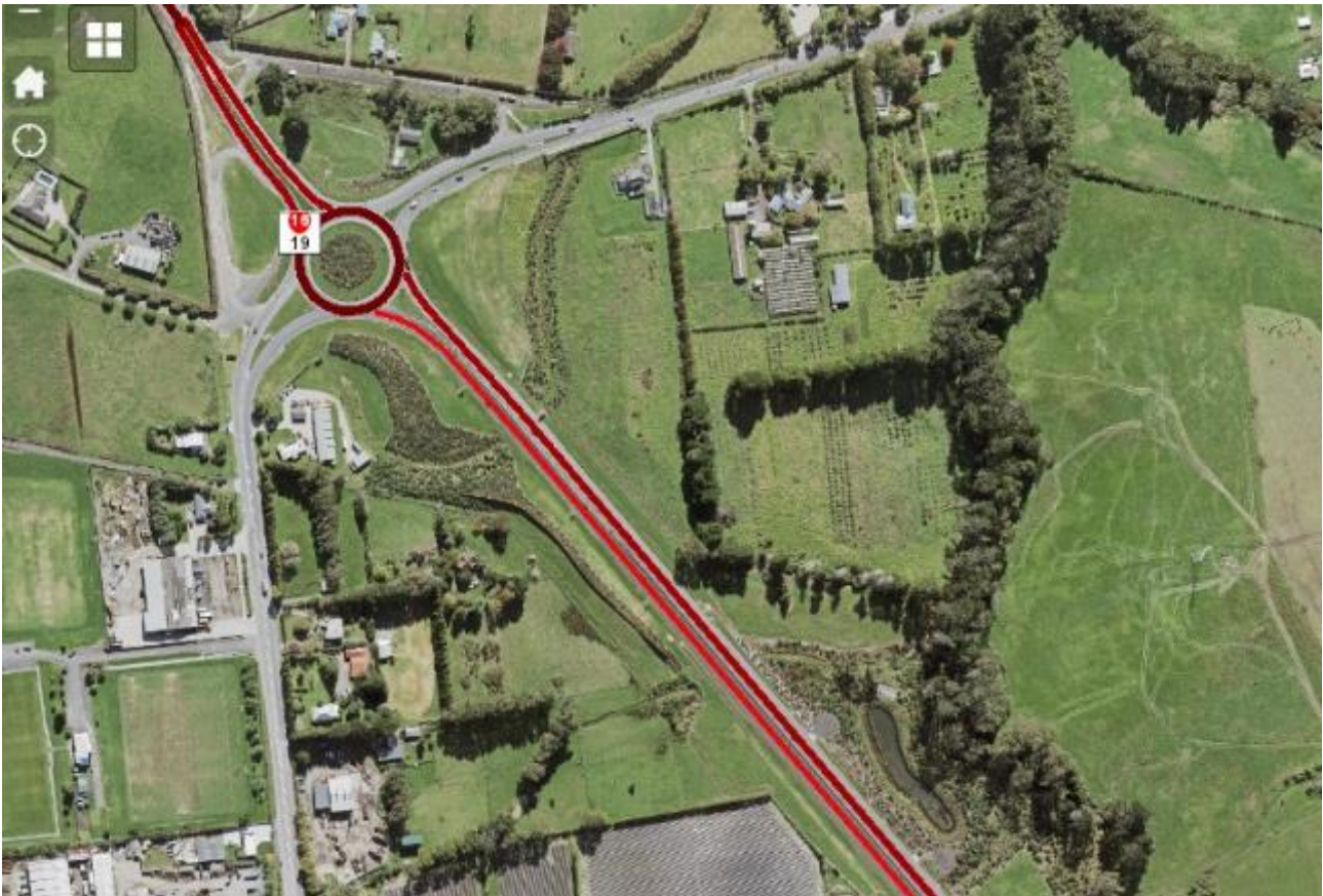
Figure 3.23 Site E. Aerial view of SH16 and Brigham Creek Road intersection. The old highways are single-lane in each direction with very narrow road buffers that have very low ecological values due to regular mowing and/or herbicide use, high noise, and exposure. The new highway stormwater pond (bottom right) is enhanced with native planting, which could be extended south into pasture. Space to the right of the roundabout may be retained for another stormwater treatment device.
