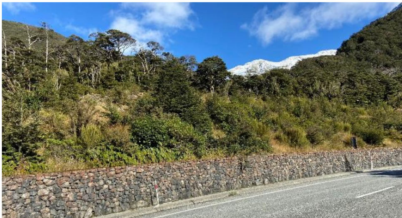
Figure 4.26 The road footprint in Arthur's Pass National Park is reduced by using vertical rock walls and reduced margin with concrete kerb. The vertical wall could also be a barrier to kiwi. (Photo taken in April 2021.)
