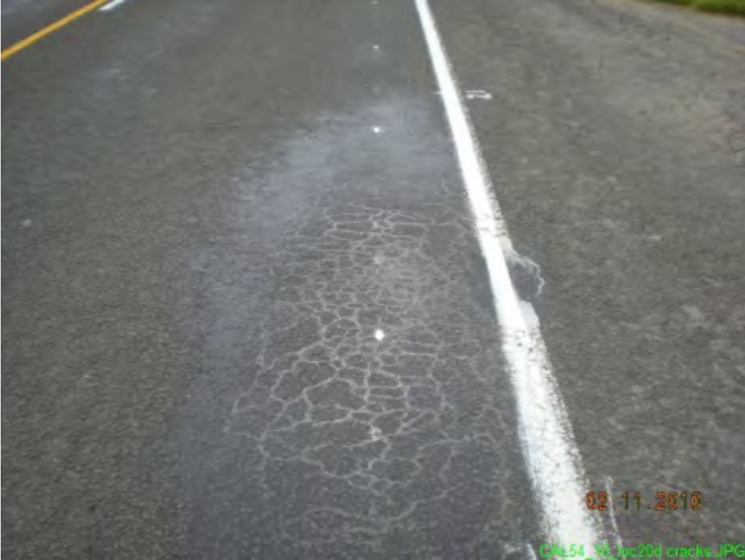
Figure A.5 Photograph 5, CAL- 54, 2 November 2010 loc 20- 21d flushing and cracking
