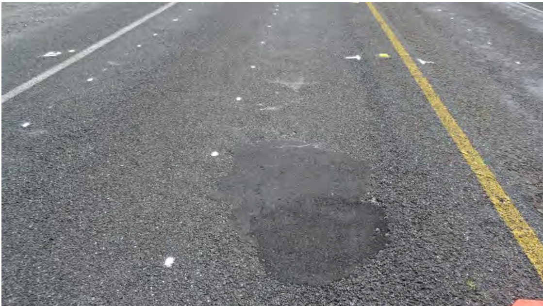
Figure A.11 Photograph 11, CAL- 54, 29 October 2015 loc 20- 21d cracking and patching in the 2014 maintenance repair
