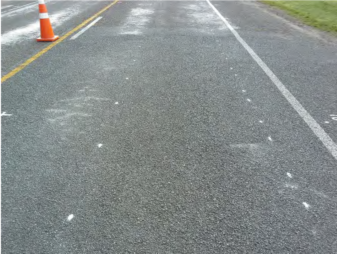
Figure A.11 Photograph 11, CAL- 54, 29 October 2015 loc 20- 21d cracking and patching in the 2014 maintenance repair
