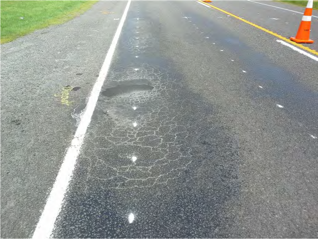
Figure A.9 Photograph 9, CAL- 54, 17 October 2013 loc 20- 21d flushing and cracking
