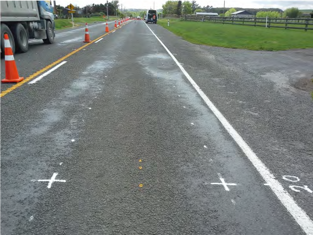
Figure A.9 Photograph 9, CAL- 54, 17 October 2013 loc 20- 21d flushing and cracking
