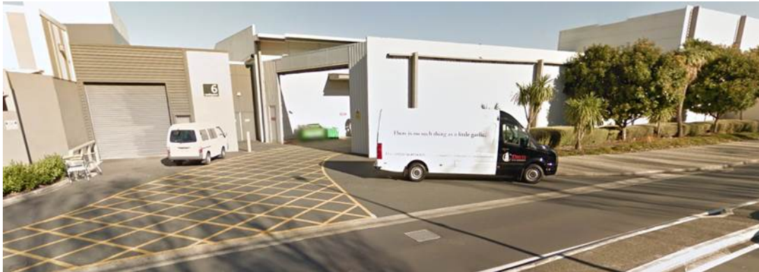
Figure 8.25 Larger loading dock and inward goods area at the southern end of Sylvia Park
