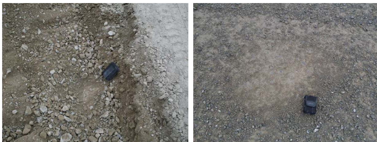
Figure 6.3 In-situ cement stabilisation and finished surface appearance
