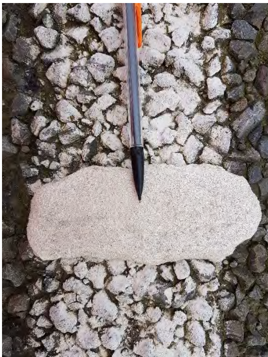
Site two baseline edgeline with ATP
