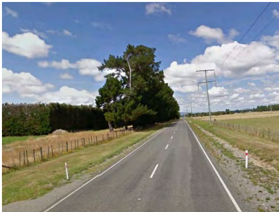
Full EMP: Straight road before intervention with EMPs, RRPMS, edgelines and centrelines
