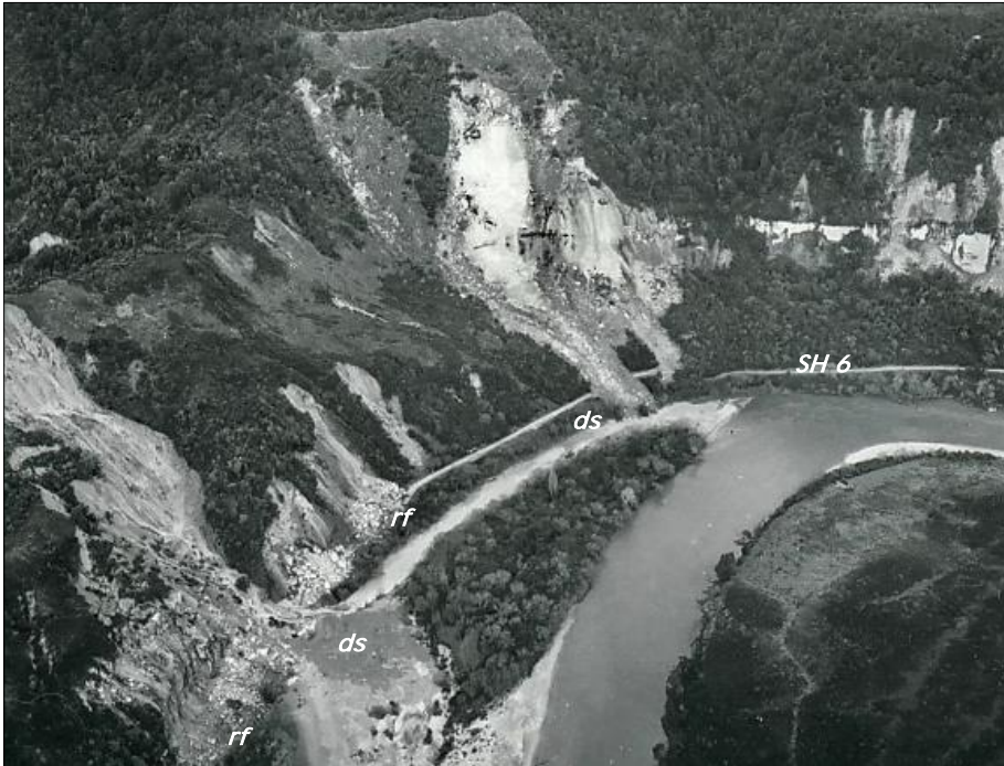
Figure A.13 Rock falls ( rf ) and debris slides ( ds ) from road cuts and bluffs of Tertiary limestone during the Inangahua earthquake buried SH6 for a length of about 1km along the Buller River at White Cliffs, 4km northwest of Inangahua, causing that section of the highway to be relocated well out from the base of the cliffs.
