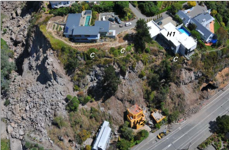
Figure A.7 Houses at the foot of the old sea cliff at Redcliffs were damaged by rock falls, and houses at the top of the cliff were damaged by ground cracking ( C ) during the 22 February mainshock and were undermined during subsequent cliff collapses during aftershocks. Two houses ( H1 , H2 ), had to be demolished at this site.
