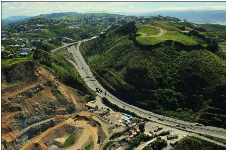
Figure A.18 The steep ( 60\text{--}65^\circ ) 60m cut slopes along SH1 in the Ngauranga Gorge (bottom right) are believed to be vulnerable to landsliding during a Wellington fault earthquake (MM9-10, with PGAs of \sim 0.5 to 1.0g or > ). These cuts have not been tested by a large earthquake since they were constructed in the 1950s.
