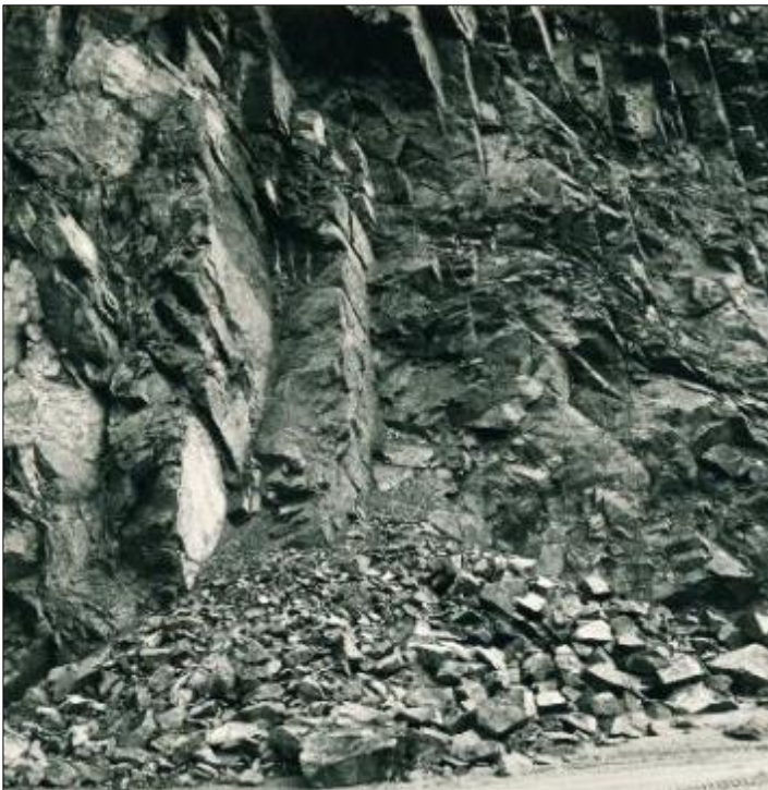
Figure A.23 Joint-controlled rock falls in weathered granite damaged many SH6 road cuts in the upper Buller Gorge during the 1968 Inangahua earthquake. In this photo most of the rock fall debris that initially blocked the road has been cleared away, but the cut slope is still highly vulnerable to further rock falls.
