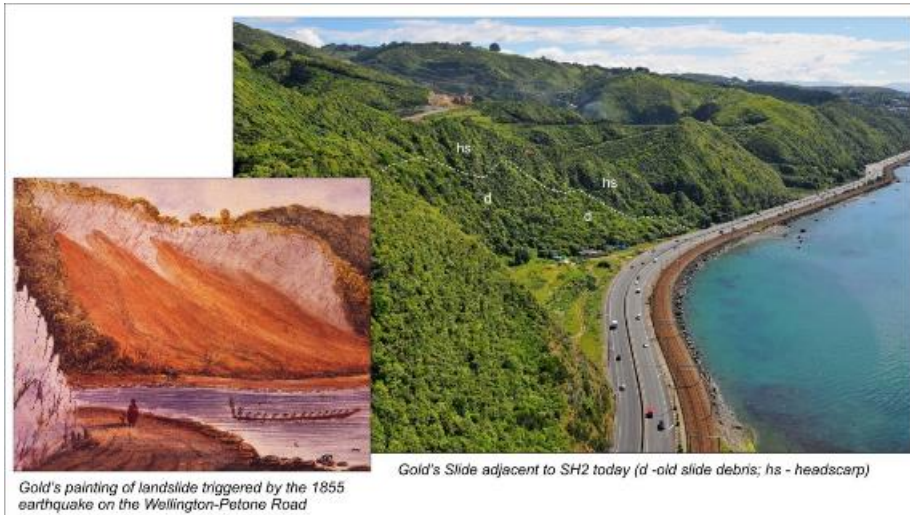
Figure A.17 'Gold's Landslide' ( \sim 300,000\text{m}^3 ) on the Hutt Road (SH2), which was triggered by the 1855 Wairarapa earthquake, illustrates the potential for similar failures to occur during a Wellington fault earthquake.
