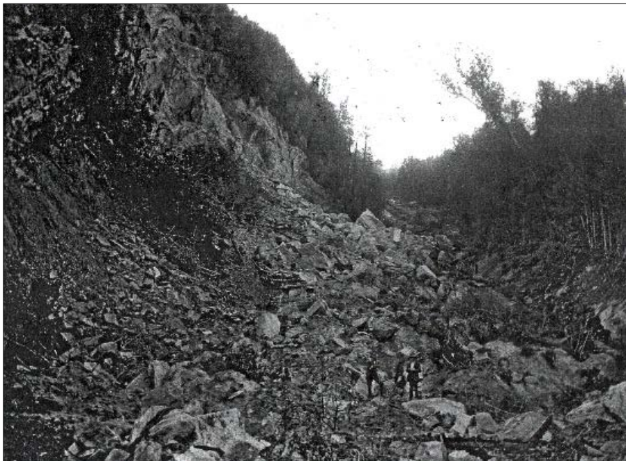
Figure A.16 Extensive rock falls triggered by the 1929 Murchison earthquake completely buried parts of the road in the upper Buller Gorge. Below, the extensive rock falls that covered the gorge road near Lyell Creek.
