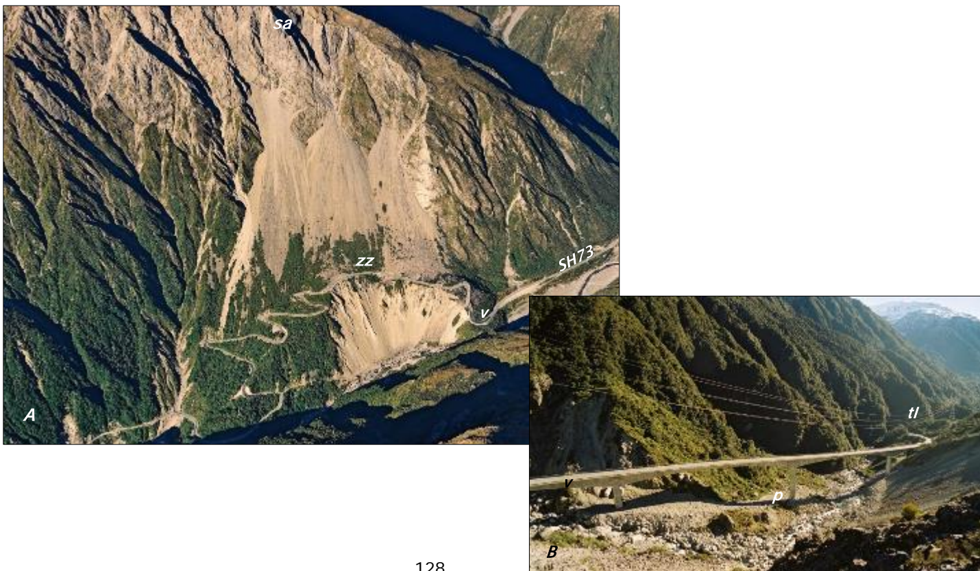
Figure A.31 Built below a prehistoric rock avalanche source area ( sa ) at the 'zig-zag' ( zz ) on SH73 at Arthur's Pass, the viaduct ( v ) and electricity transmission lines ( tl ) are at significant risk from another rock avalanche at this site during the next alpine fault earthquake and other large earthquakes in the region.
