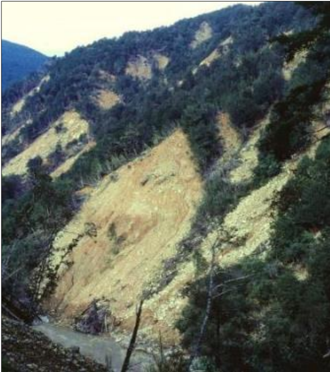
Figure A.23 Joint-controlled rock falls in weathered granite damaged many SH6 road cuts in the upper Buller Gorge during the 1968 Inangahua earthquake. In this photo most of the rock fall debris that initially blocked the road has been cleared away, but the cut slope is still highly vulnerable to further rock falls.
