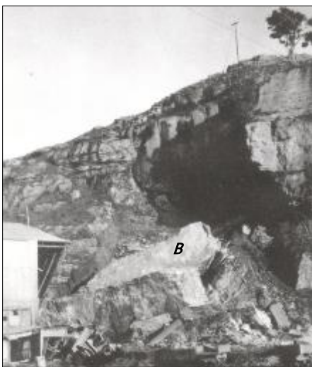
Figure A.33 The Murchison earthquake triggered a fall of large blocks (B) of Tertiary limestone on a cliff at the Tarakohe Cement Works near Takaka. The rock fall buried and destroyed the powerhouse and killed an engineer.
