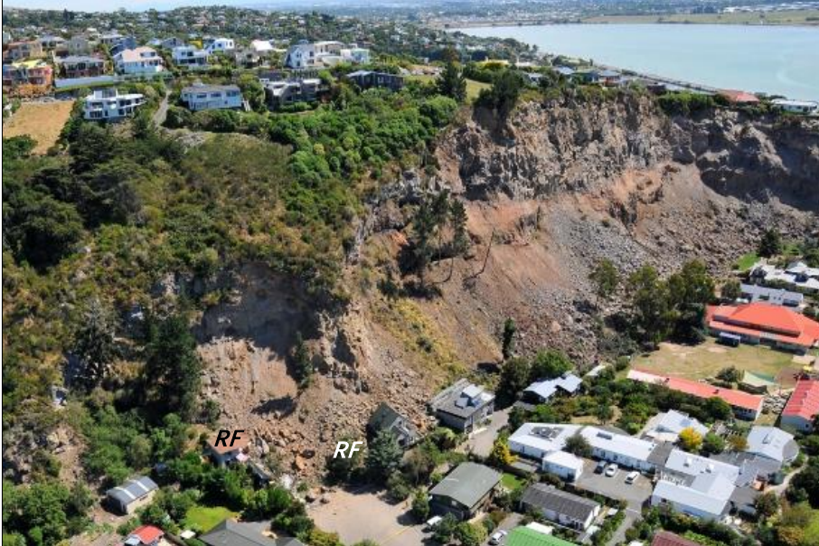
Figure A.7 Houses at the foot of the old sea cliff at Redcliffs were damaged by rock falls, and houses at the top of the cliff were damaged by ground cracking ( C ) during the 22 February mainshock and were undermined during subsequent cliff collapses during aftershocks. Two houses ( H1 , H2 ), had to be demolished at this site.
