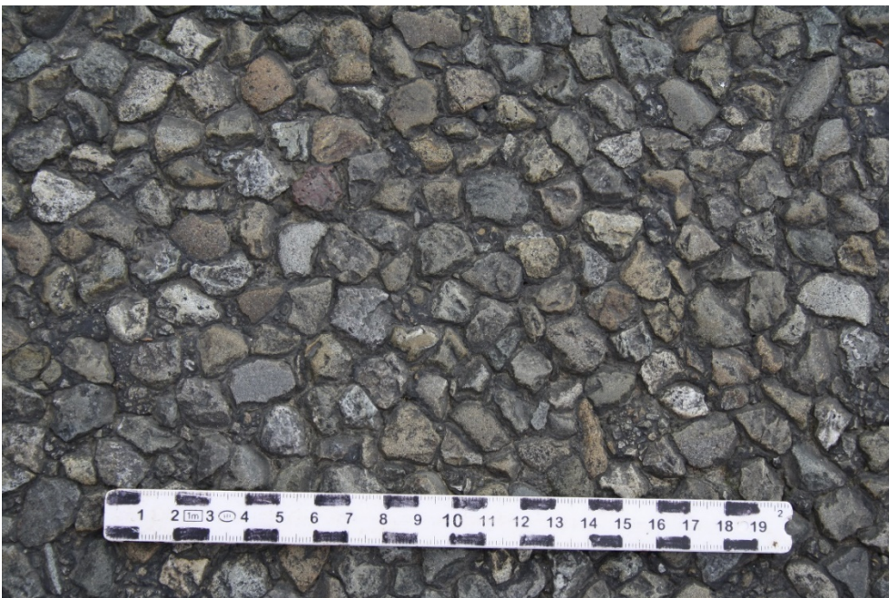
Figure 3.3 Binder is plastic rather than brittle
