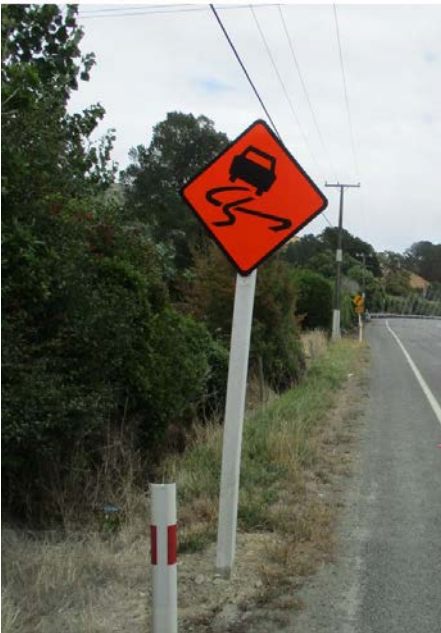
Figure 3.6 Temporary sign with no supplementary plate (reflectorised fluorescent orange)
