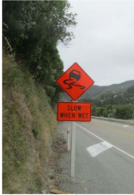
Figure 3.7 Temporary sign with 'Slow when wet' supplementary plate (reflectorised fluorescent orange)
