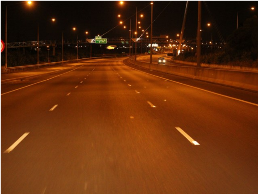
Figure D.6 A lighting scheme with a very high average luminance near the top end of the sample's distribution for both average luminance and uniformity [ \bar{L} = 1.6 , U_o = 0.65 , UI = 0.72 ]
