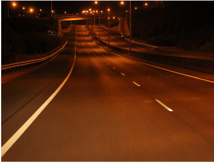
Figure D.2 An installation with strong dark bands illustrating poor longitudinal uniformity [ \bar{L} = 0.91 , U_o = 0.22 , U_l = 0.06 ]
