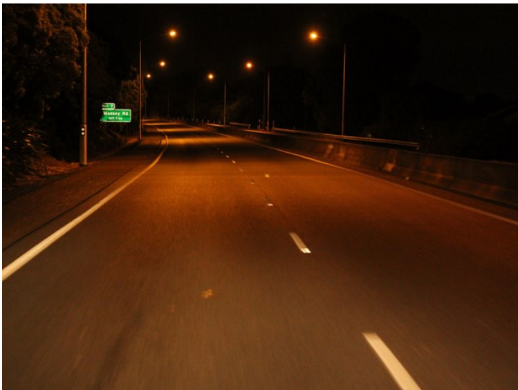
Figure D.2 An installation with strong dark bands illustrating poor longitudinal uniformity [ \bar{L} = 0.91 , U_o = 0.22 , U_l = 0.06 ]
