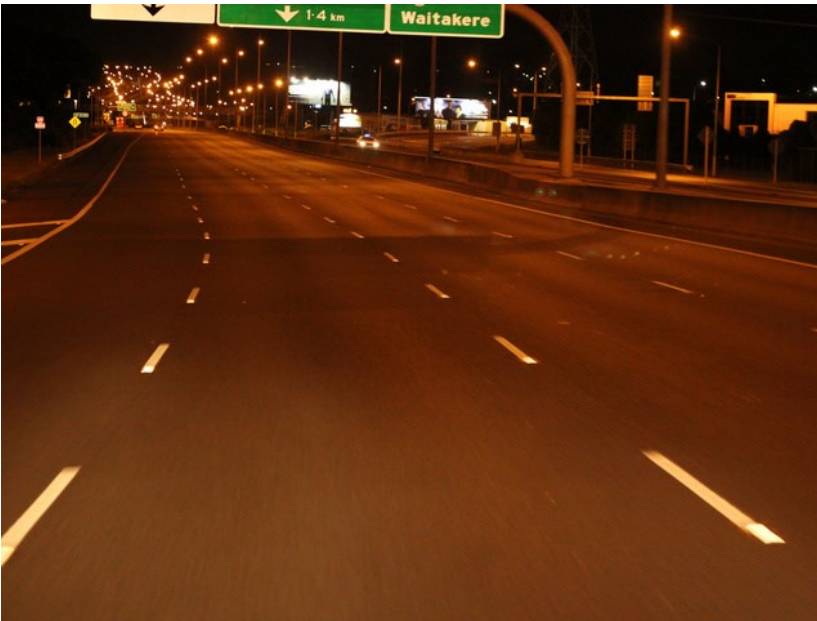
Figure D.4 An installation with a low average luminance but acceptable uniformity [ \bar{L} = 0.44 , U_o=0.33 , U_l = 0.36 ]
