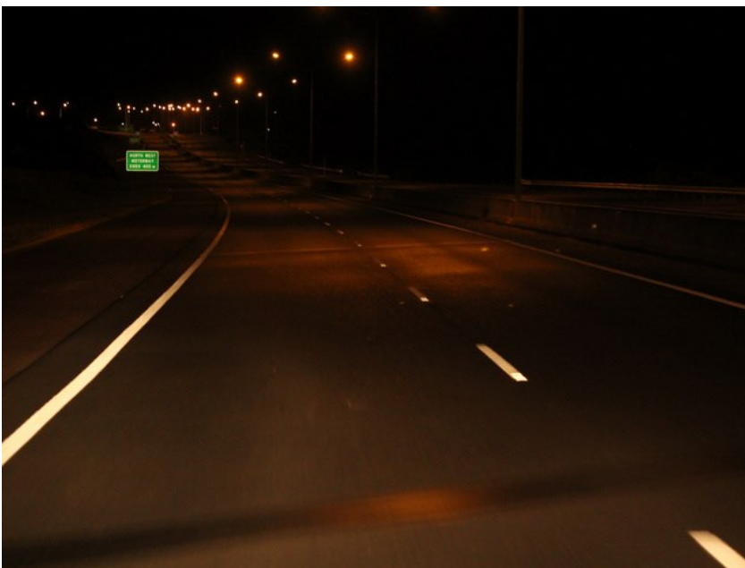
Figure D.4 An installation with a low average luminance but acceptable uniformity [ \bar{L} = 0.44 , U_o=0.33 , U_l = 0.36 ]
