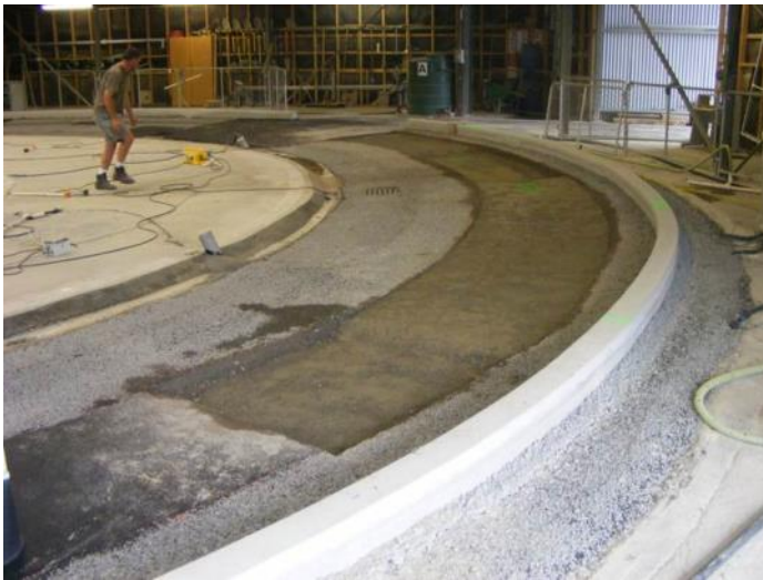
6 December 2011 section A repairs
