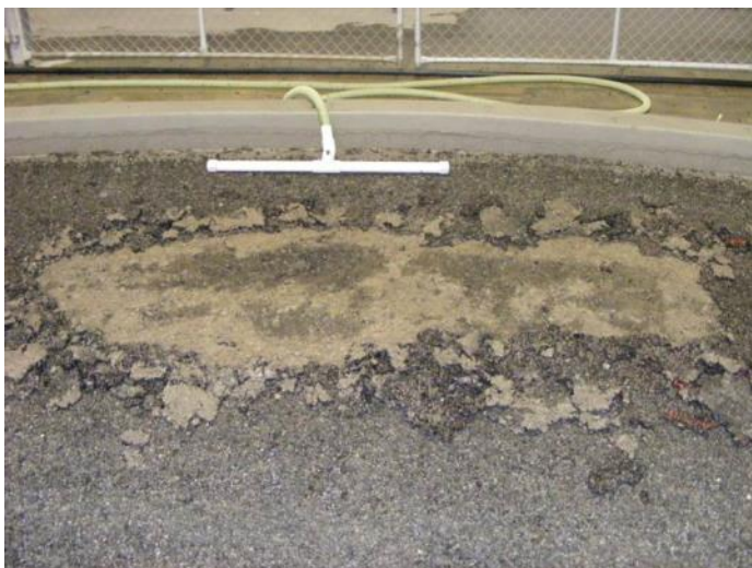
24 January 2012 section B top scraped back to dry material
