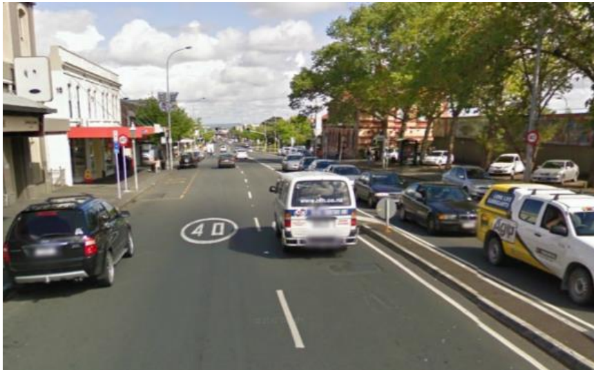
Figure 3.23 Example of signage and road markings visible when entering the Ponsonby Road lowered speed limit zone
