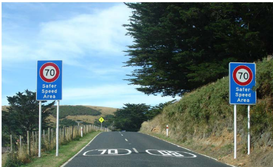
Figure 3.8 Example of signage and road markings used on the Otago Peninsula
