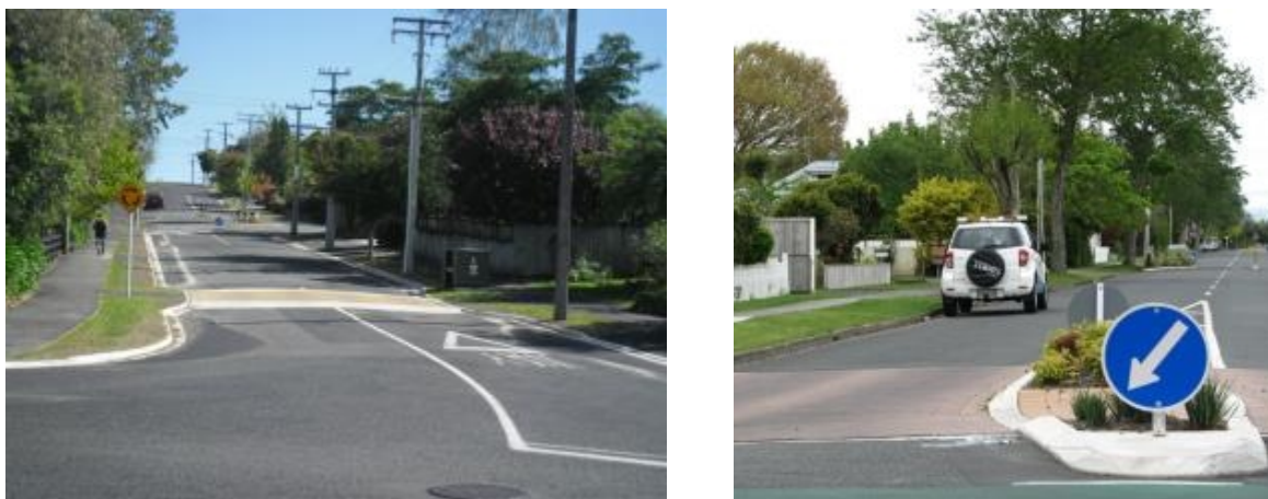
Figure 3.18 Examples of physical works conducted during the first stage
