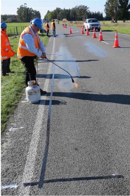
Figure 8.5 Binder and chip application
