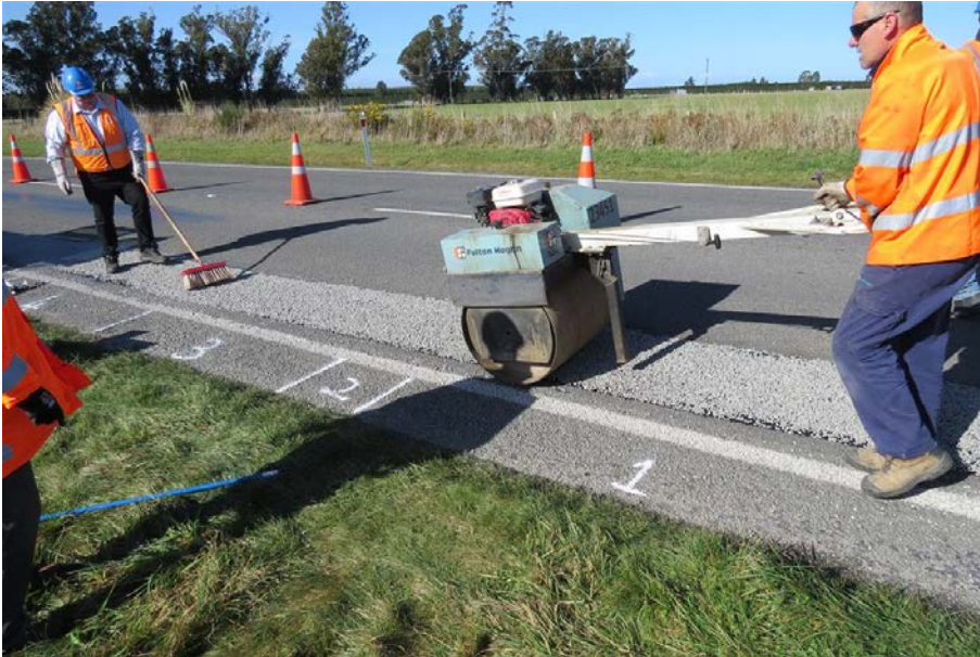
Figure 8.7 Rolling of the test patch and showing sections 1-4
