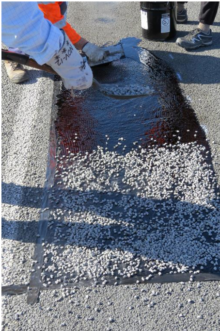
Figure 8.5 Binder and chip application
