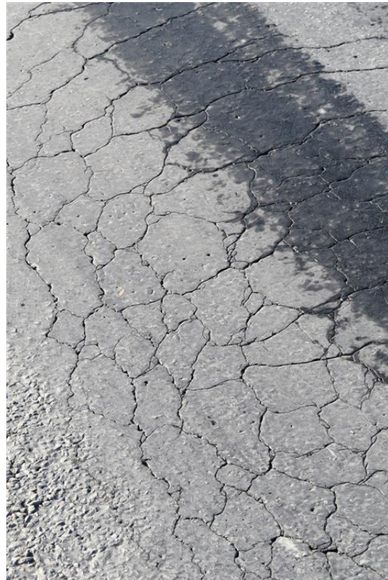
Venting holes are also apparent
