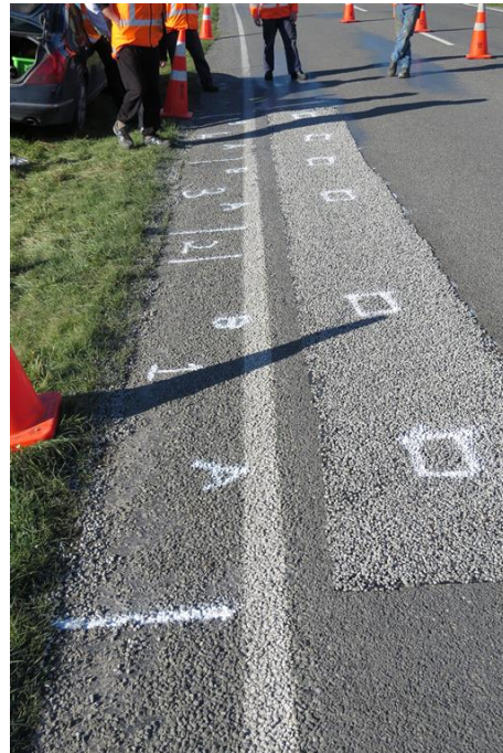
Figure 8.6 Completed patch with marked squares for chip counting
