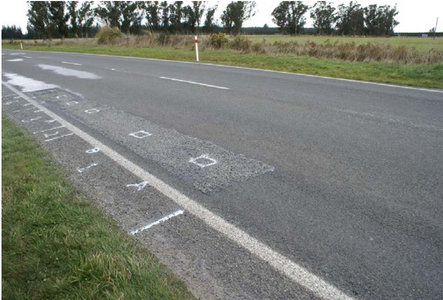
Figure 8.9 Test patch the day after construction showing chip loss through cohesive failure of the binder
