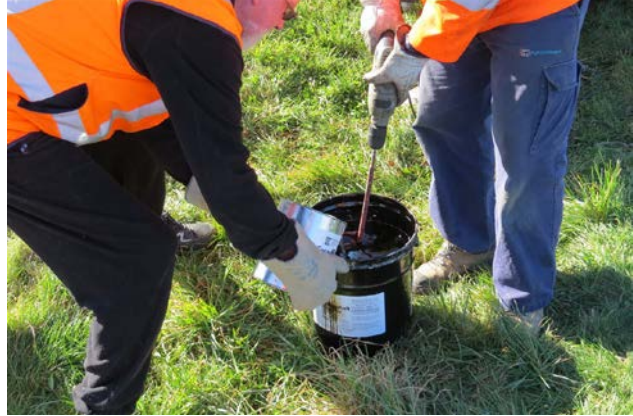
Figure 8.4 2% epoxy bitumen mixed on site
