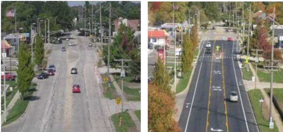
Figure 1.1 Before and after example of road space reallocation, city of Urbana, Illinois (VTPI 2013)
