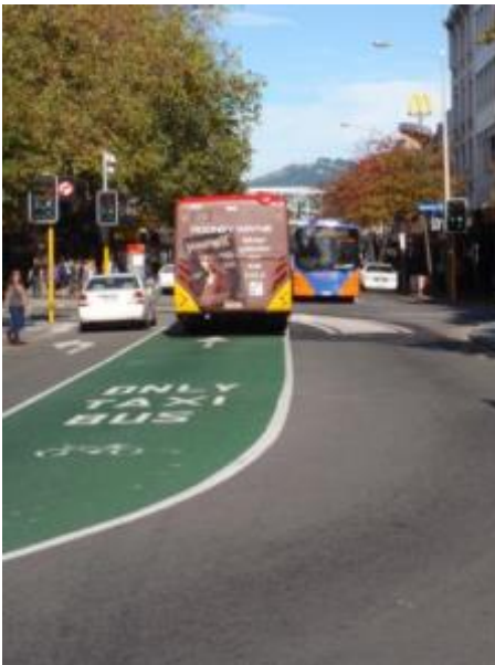
Figure 3.9 Example of a bus priority measure – Christchurch, New Zealand
