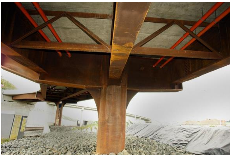
Figure 4.5 State Highway 1 Mercer to Longswamp off-ramp, shortly after construction
