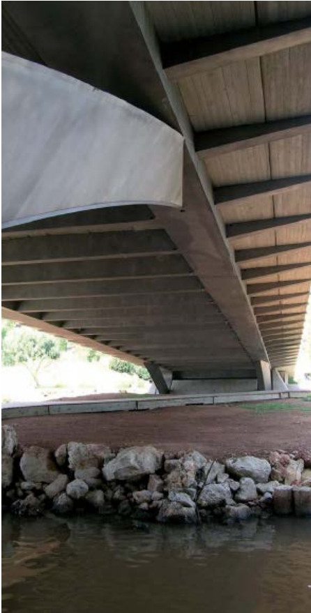
Figure 11.8 The underside of the Cala Galdana Bridge
