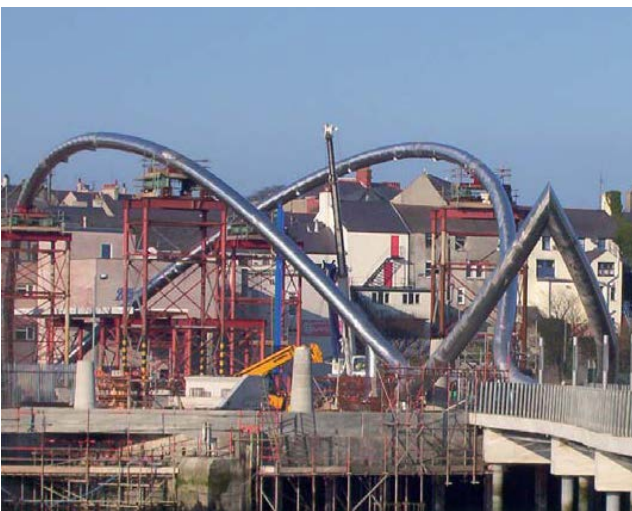
Figure 11.7 The Celtic Gateway Bridge in Holyhead, Wales
