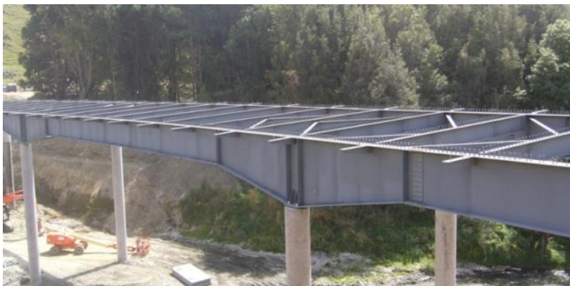
Figure 2.7 Ladder deck bridge with haunched main girders (image courtesy of Holmes Consulting Group)
