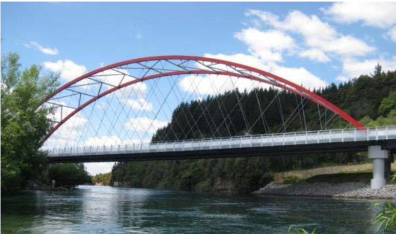
Figure 11.2 Waikato Network Arch Bridge near Taupo (image courtesy of Holmes Consulting Group)
