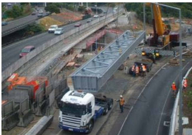
Figure 11.1 Steel-concrete composite box girder
