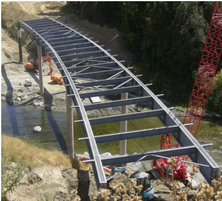
Figure 2.7 Ladder deck bridge with haunched main girders (image courtesy of Holmes Consulting Group)
