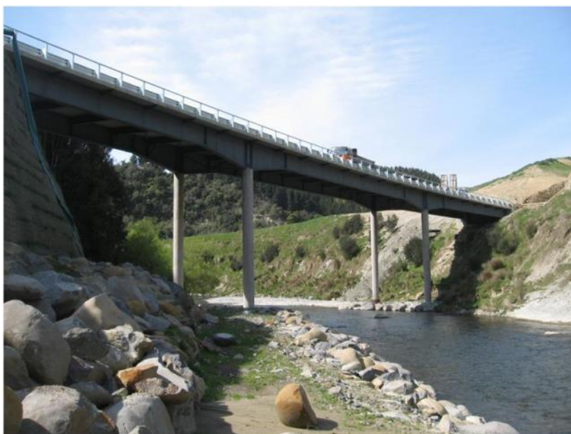
Figure 3.3 SH4 Okura Southern Bridge (image courtesy of Holmes Consulting Group)
