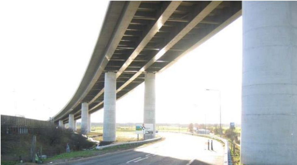
Figure 2.4 Crosshead girder in a multi-girder bridge
