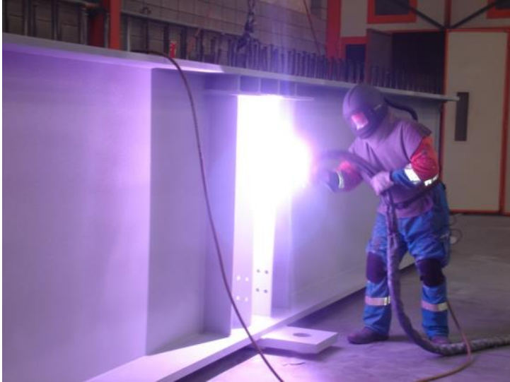
Figure 4.4 Coating application on the Kopu Bridge beam (image courtesy of D&H)
