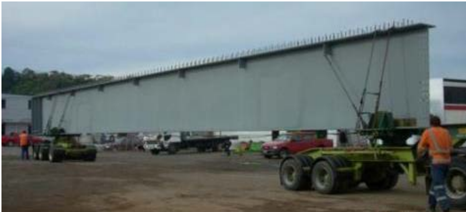
Figure 4.2 Transporting a 20.3m, 30.5 tonnes bridge girder (Image courtesy of Eastbridge)
