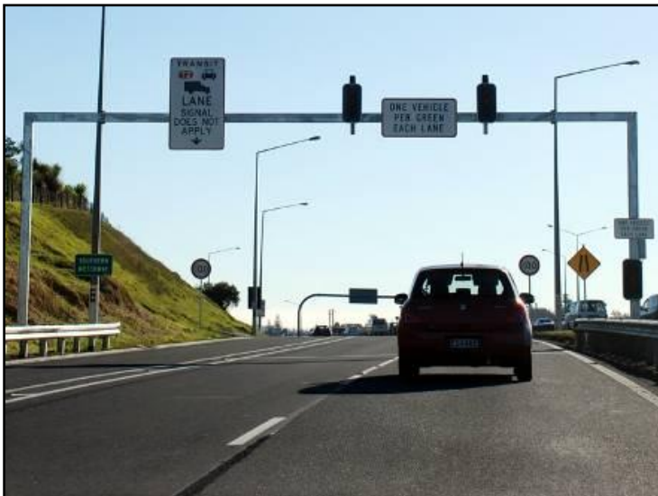
Figure A6.1 Ramp metering at Mt Wellington on-ramp SH1, with T2 (HOV2 +/bus) and truck bypass jump lane
