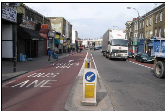
Figure B5.11 Contra-flow bus lane, UK
