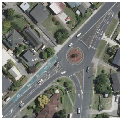
Northcote Road/Lake Road roundabout, Auckland, New Zealand
