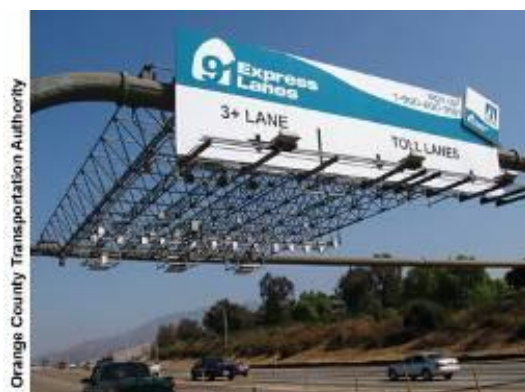
HOT lane, SR-91 Express Lanes, CA, USA
