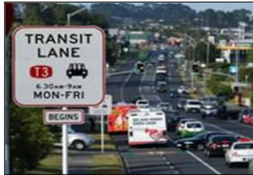
Figure B5.10 Transit lane at Constellation Drive, Auckland
