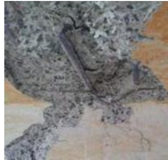
(b) Spalling
