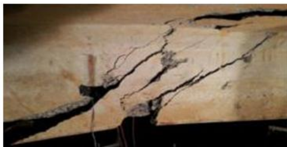
(b) Dominant crack at failure
