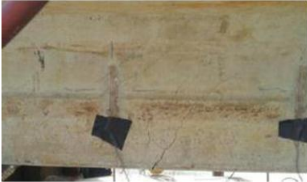
(a) Crack pattern during loading
