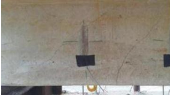
(a) Dominant crack during loading
