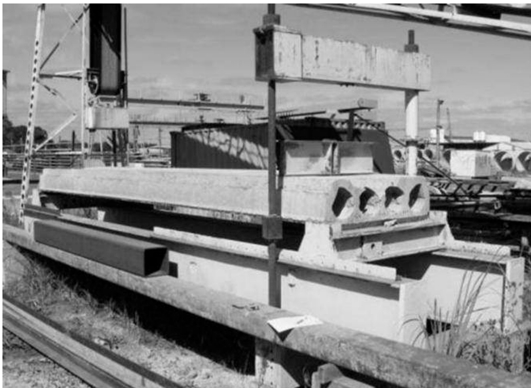
Figure 5.1 Condition of test rig at Stresscrete premises prior to project commencement
