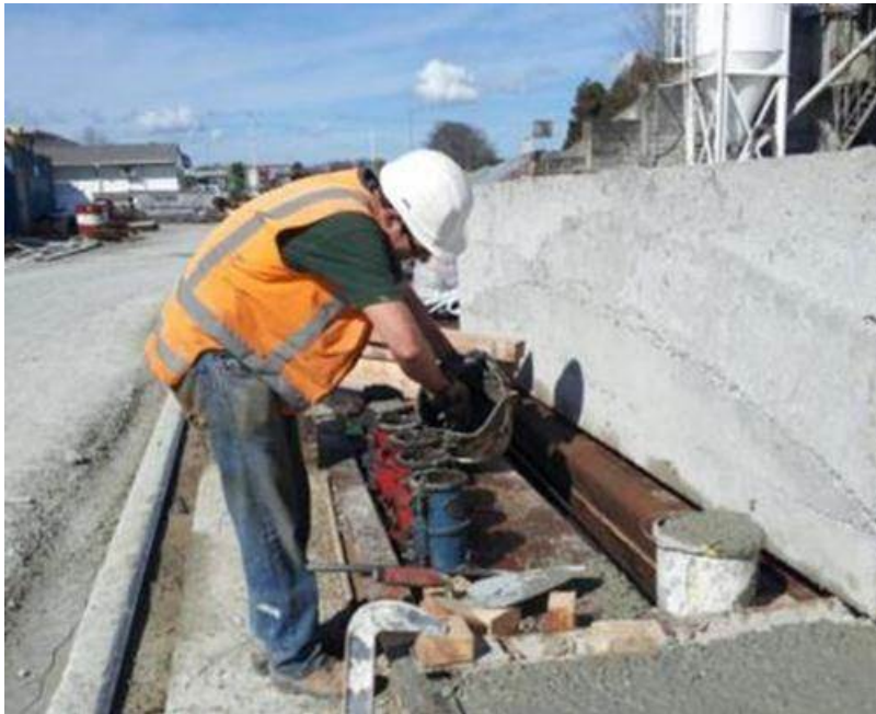
Figure 5.6 Making concrete cylinders
