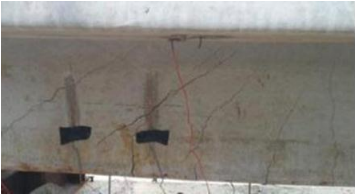
(a) Crack pattern during loading
