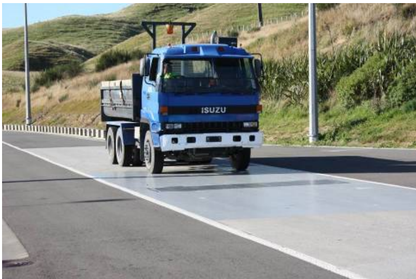
Figure 2.5 Low-speed WIM at Plimmerton Weigh Station (south) – 20m concrete approach and departure pads
