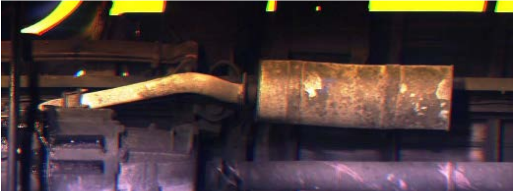
Figure 7.8 Under-vehicle camera image showing defective exhaust (courtesy of TRL and VOSA)
