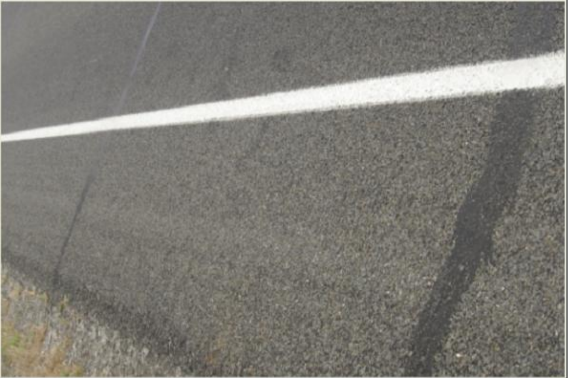
Figure E.6 SH50 RS 17/12.31 - the cracks appear to be equally spaced
