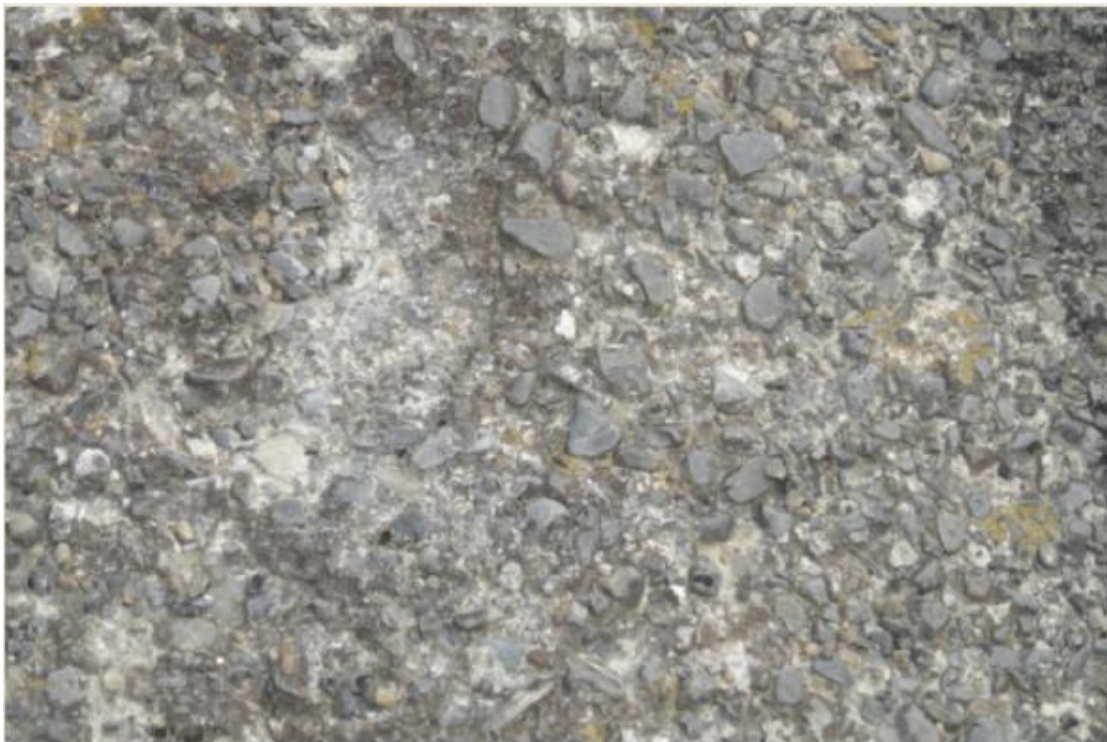
Figure E.2 SH2 RS 678\12.17 - stabilised layer visible through the shoulder (a close-up view)
