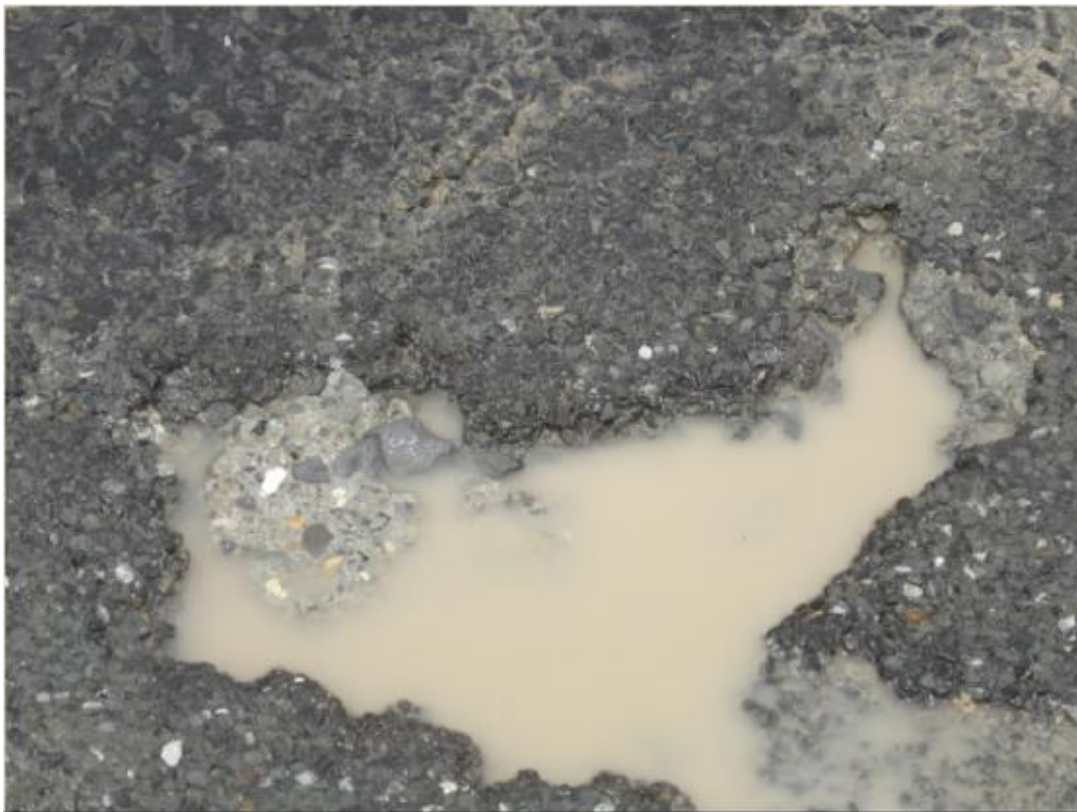
Figure E.22 Mangatu Road 10.07km - another pothole
