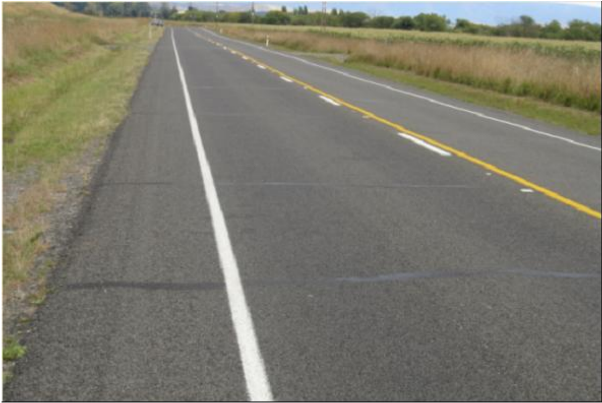
Figure E.10 SH50 RS 49/1.23 - the cracks appear in longitudinal and transverse directions
