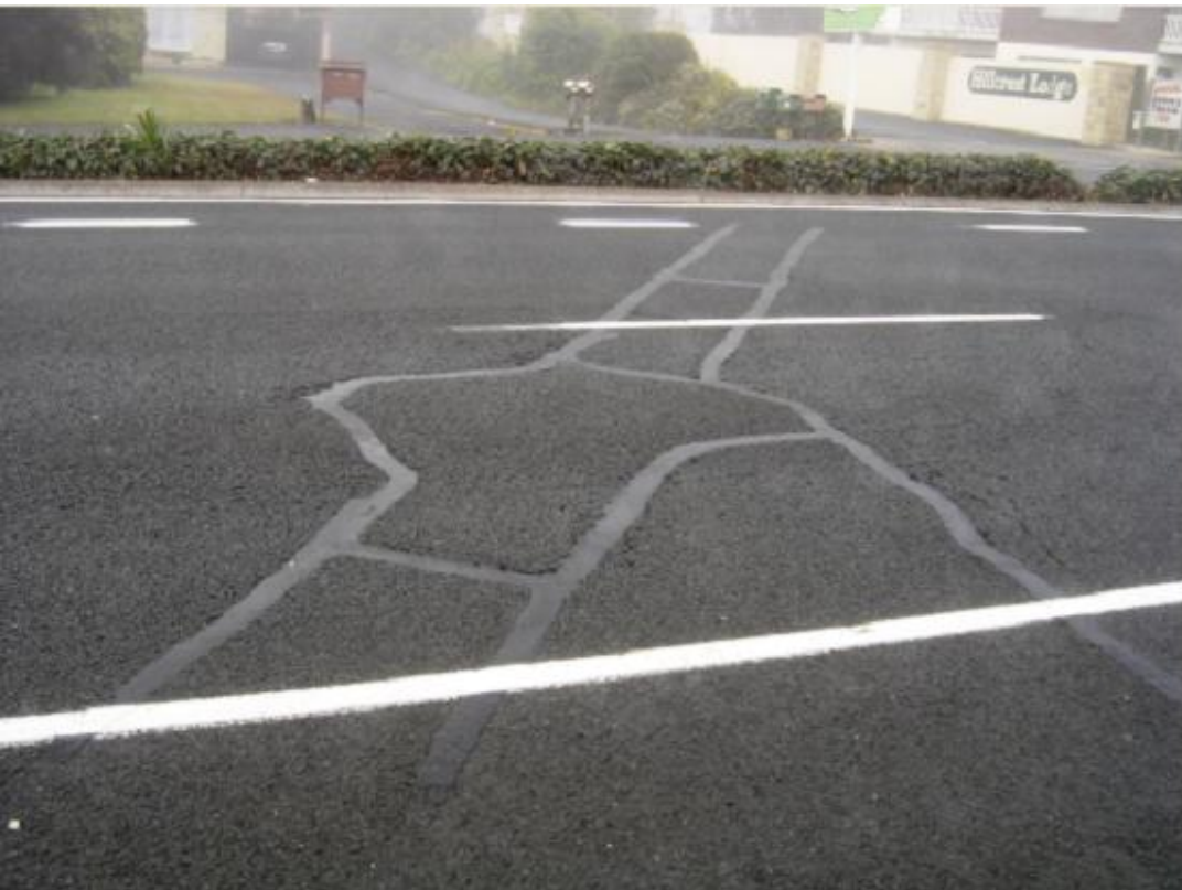
Figure E.32 SH1 RP 554/2.711 – cracks have been bandaged
