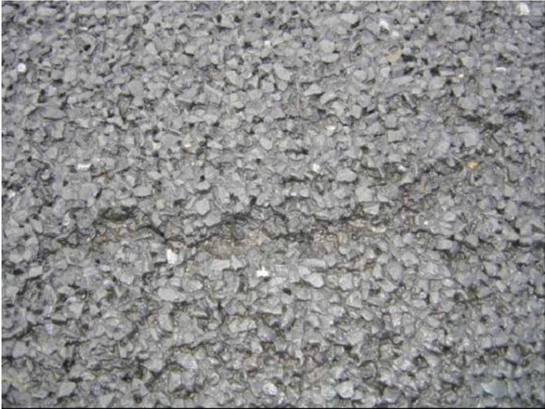
Figure E.34 SH1 RP 554/1.09 -several cracks have appeared
