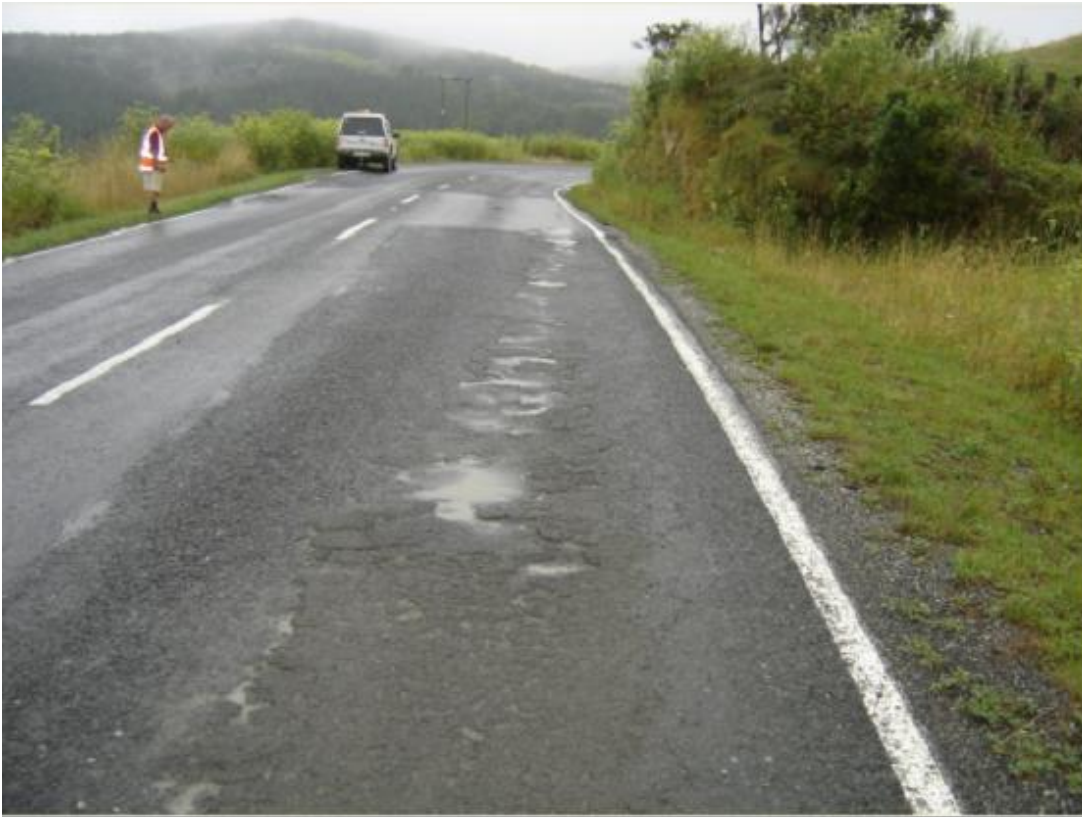
Figure E.24 Mangatu Road 10.07km – alligator cracks
