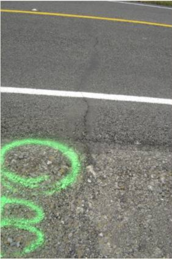
Figure E.4 SH2 RS 678\12.17 - a cracked pavement including shoulder (close-up photo)
