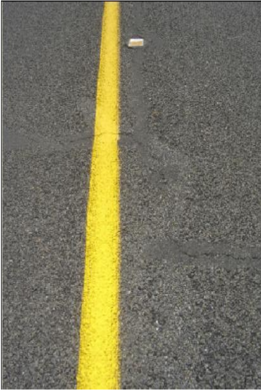
Figure E.10 SH50 RS 49/1.23 - the cracks appear in longitudinal and transverse directions
