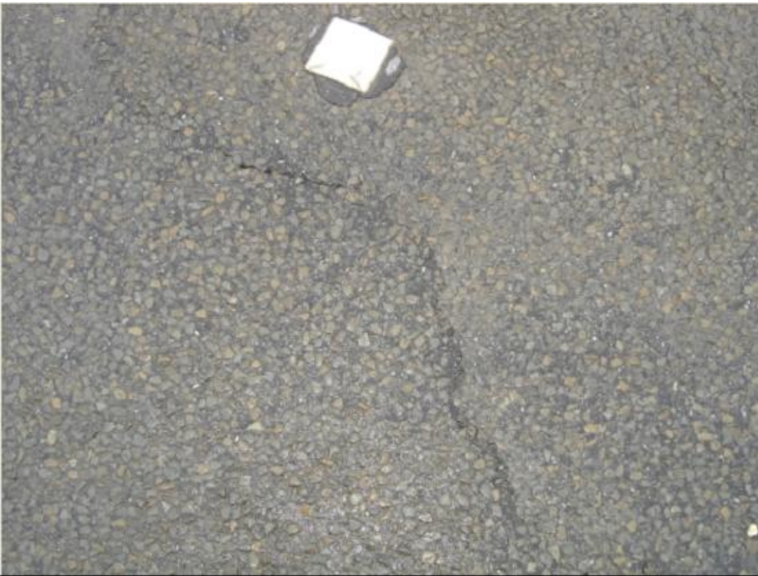
Figure E.32 SH1 RP 554/2.711 – cracks have been bandaged
