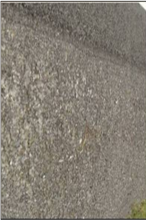
Figure E.2 SH2 RS 678\12.17 - stabilised layer visible through the shoulder (a close-up view)
