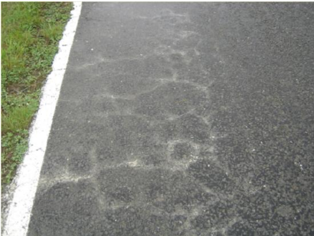
Figure E.24 Mangatu Road 10.07km – alligator cracks
