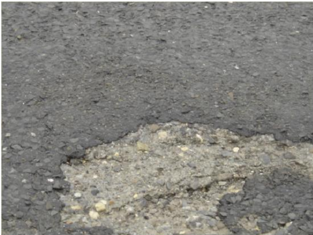
Figure E.22 Mangatu Road 10.07km - another pothole
