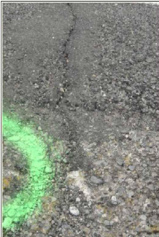
Figure E.4 SH2 RS 678\12.17 - a cracked pavement including shoulder (close-up photo)
