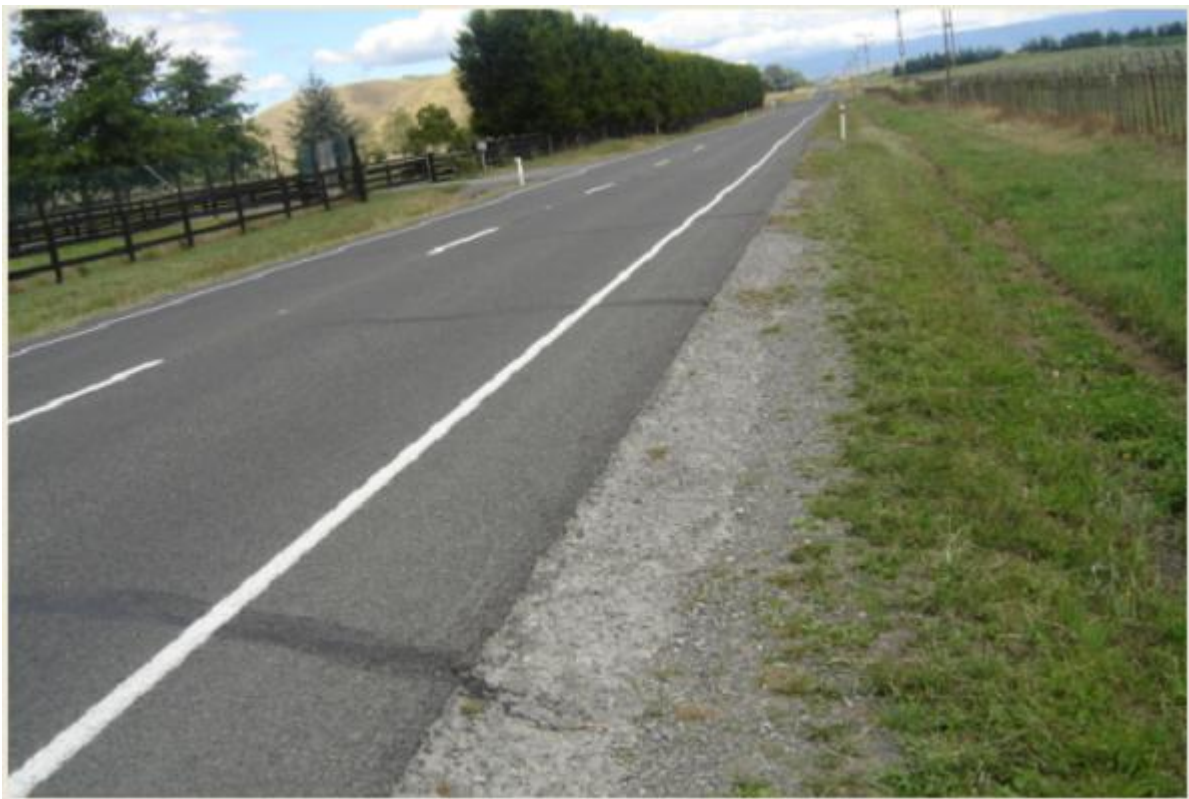
Figure E.8 SH50 RS 17/12.31 – the cracks appear to be approximately equally spaced (increasing direction)
