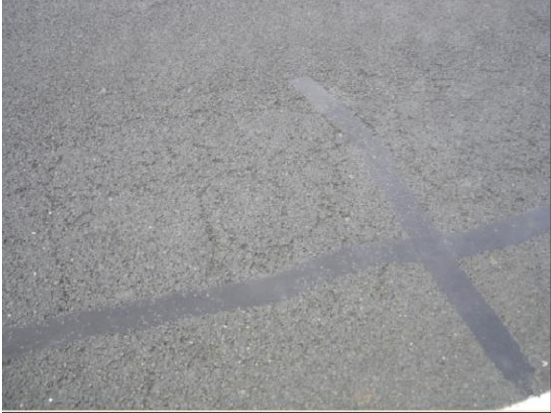
Figure E.34 SH1 RP 554/1.09 -several cracks have appeared
