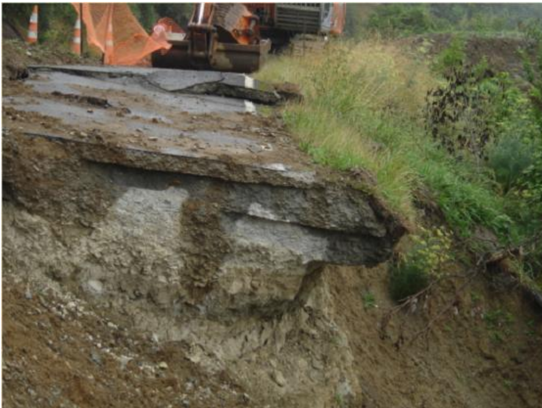
Figure E.14 Mangatu Road cross-section at 5.82km – an earth slip site (decreasing direction)
