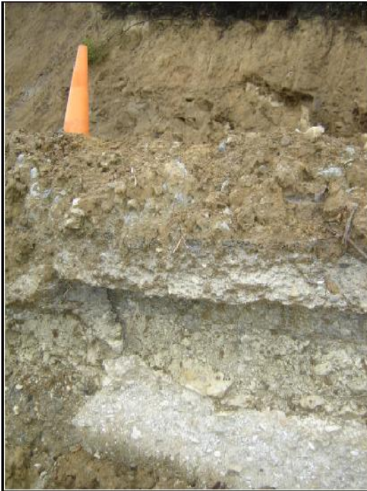
Figure E.14 Mangatu Road cross-section at 5.82km – an earth slip site (decreasing direction)
